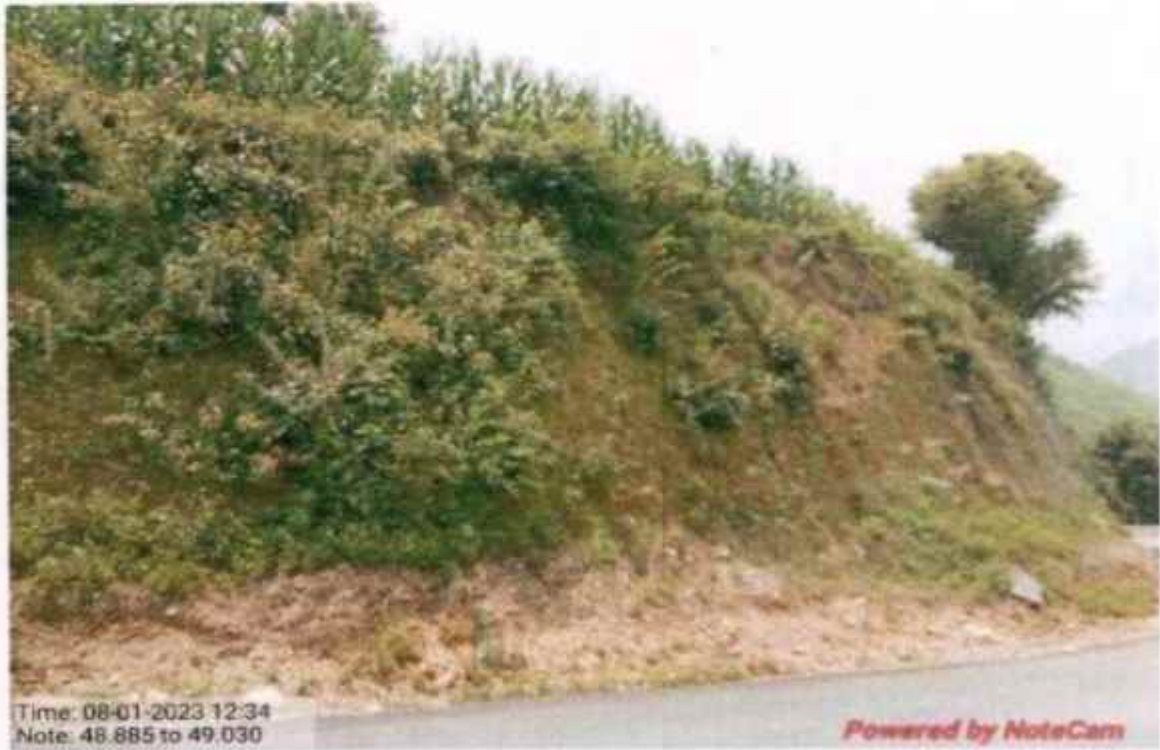
Interlink chain mesh work at km 48+885 to 49+030
