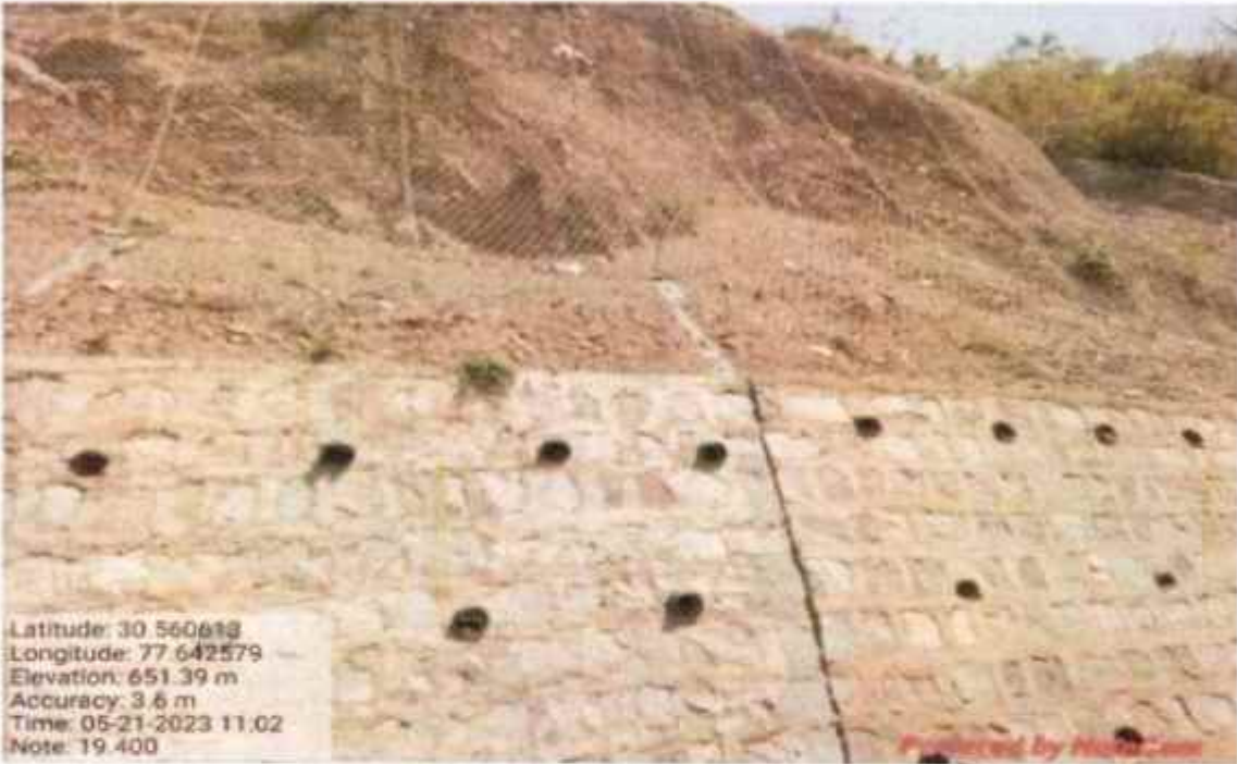
Interlink chain mesh work at Km 19+400
