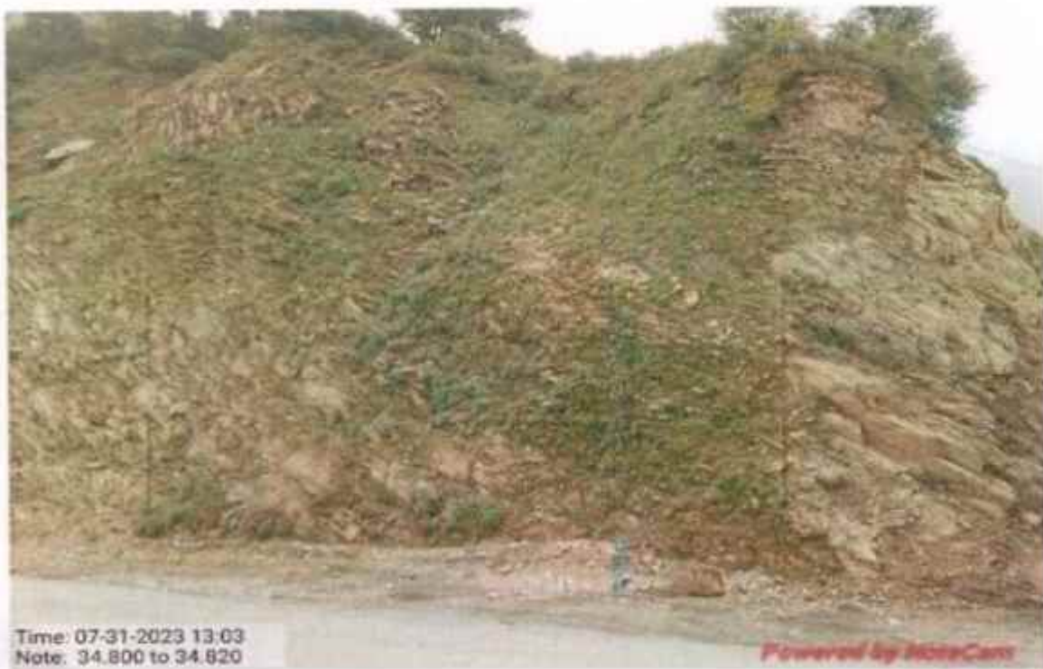
Hydro seeding work at km 34+800 to 34+820
