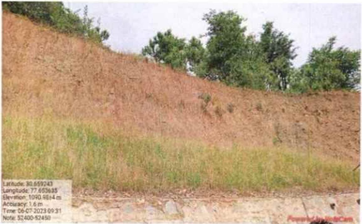
Hydro seeding work at km 52+400 to 52+450
