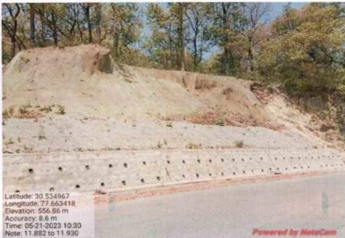
Coco fibre work at km 11+882 to 11+930
