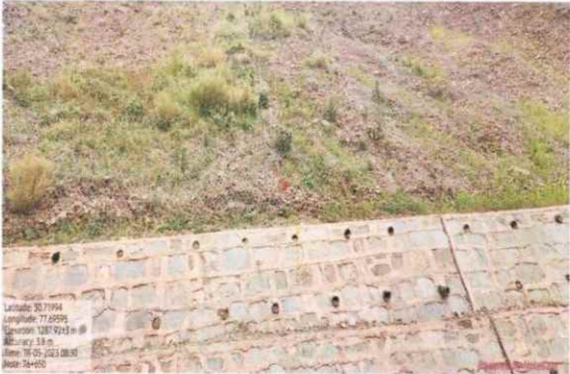
Interlink chain mesh work at km 76+650
