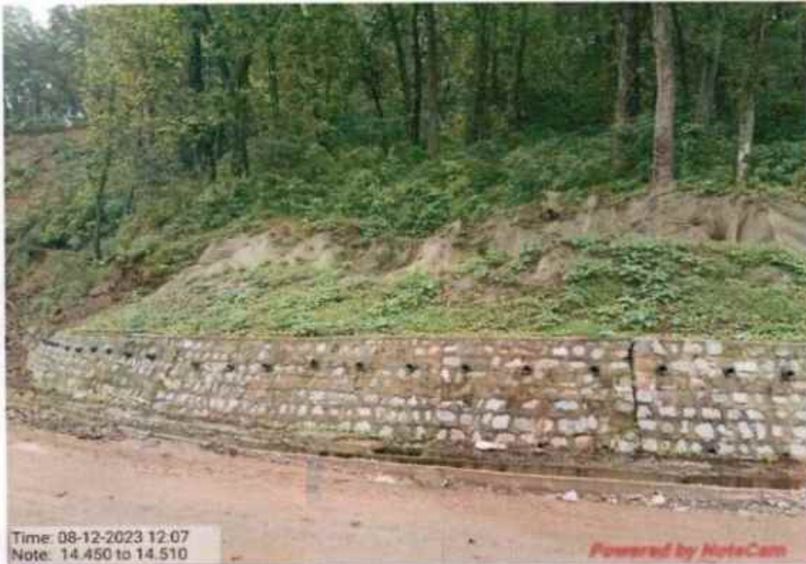
Coco fibre work at km 14.450 to 14.510
