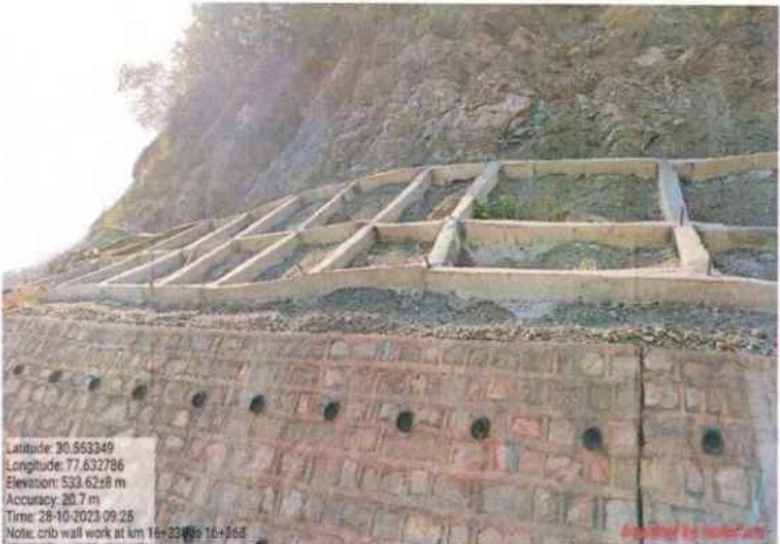
Shotcrete crib wall work at km 16+330 to 16+368
