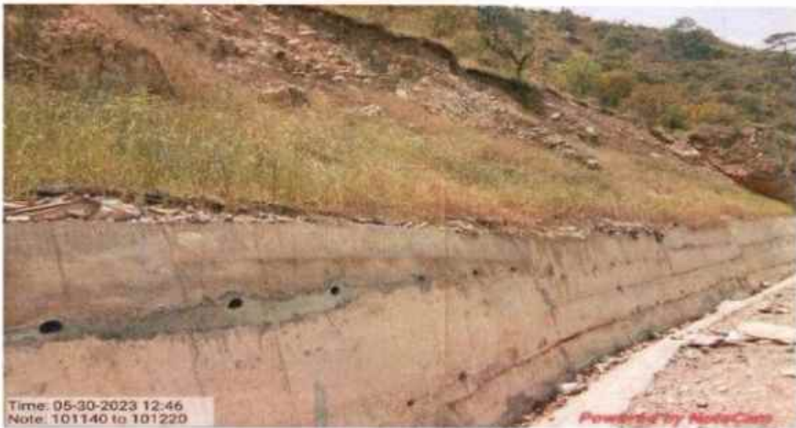
Geo cell with Hydro seeding work at km 101+140 to 101+220
