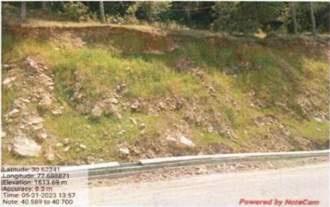
Coco fibre work at km 40+589 to 40.700
