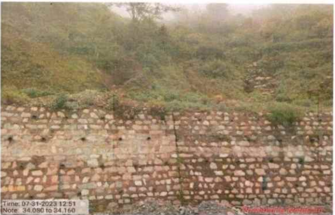
Hydro seeding work at km 34+080 to 34+160
