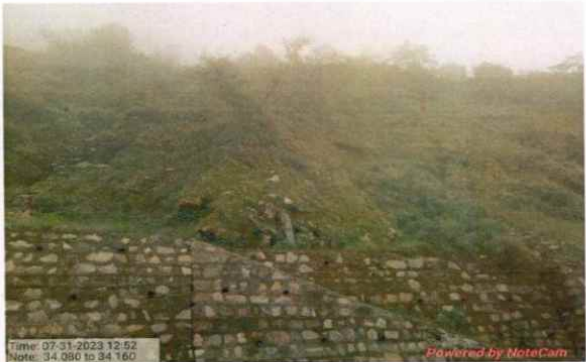
Hydro seeding work at km 34+080 to 34+160
