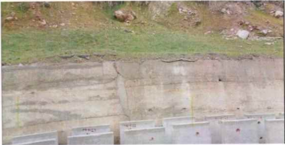
Geo cell with Hydro seeding work at km 101+140
