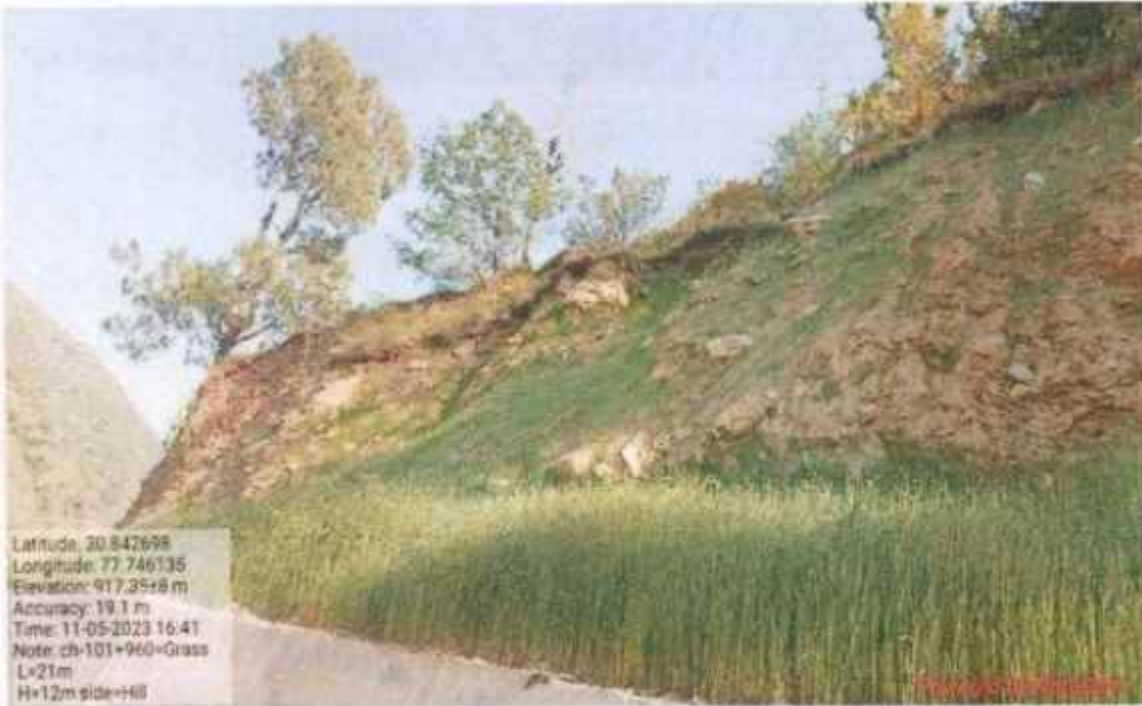
Hydro seeding and Geo cell with Hydro seeding work at km 101+960
