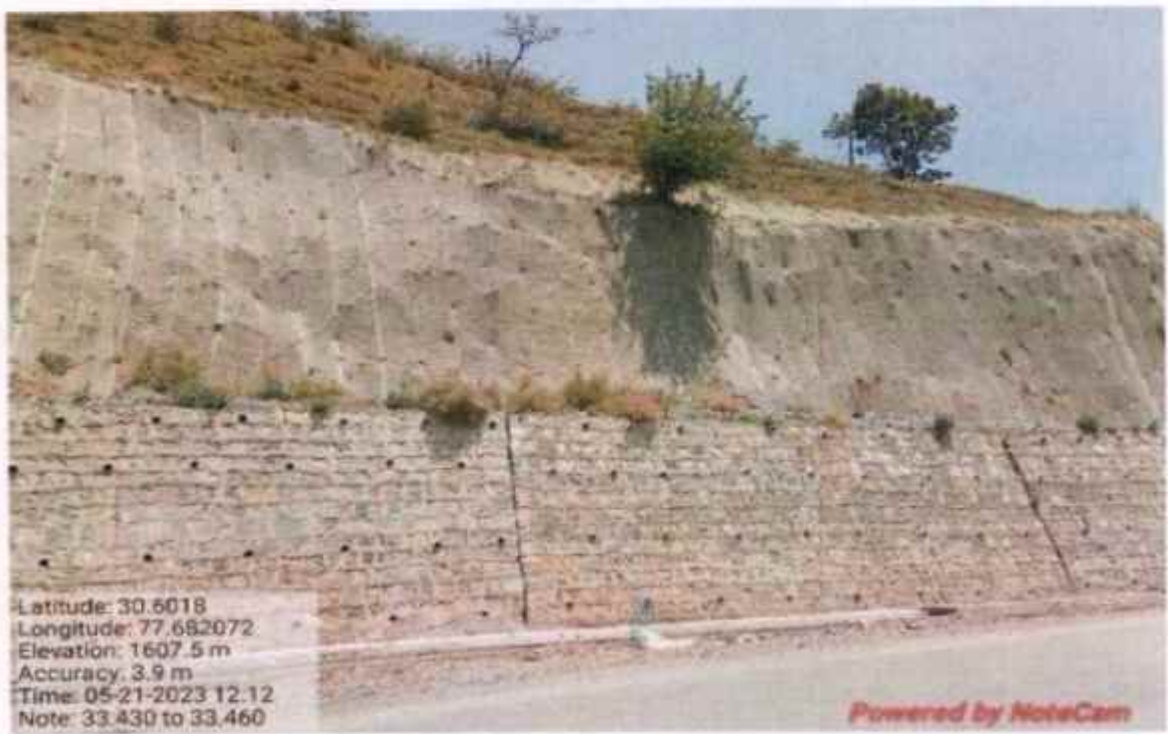
Coco fibre work at km 33+430 to 33+460
