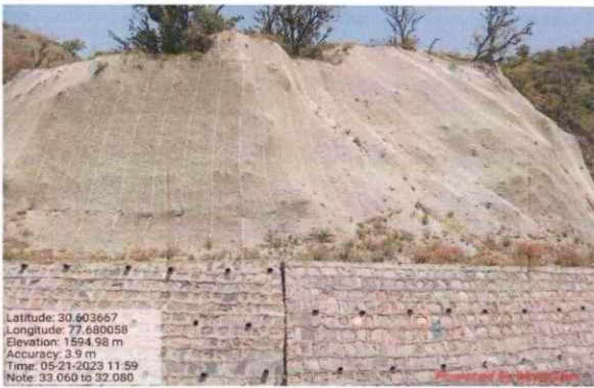
Coco fibre work at km 33+060 to 33+080
