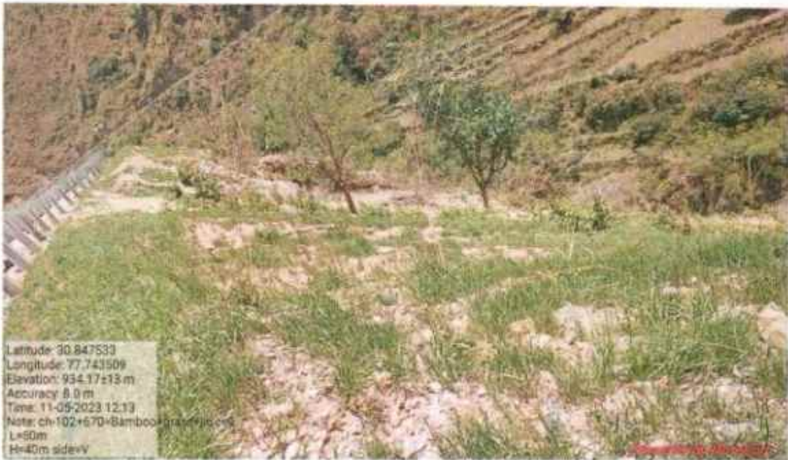
Valley side Geo cell with Hydro seeding and Bamboo plantation work at km 102+670
