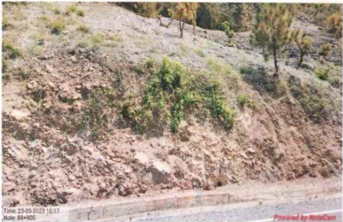
Interlink chain mesh work at km 88+900
