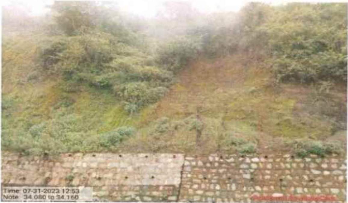
Hydro seeding work at km 34+080 to 34+160
