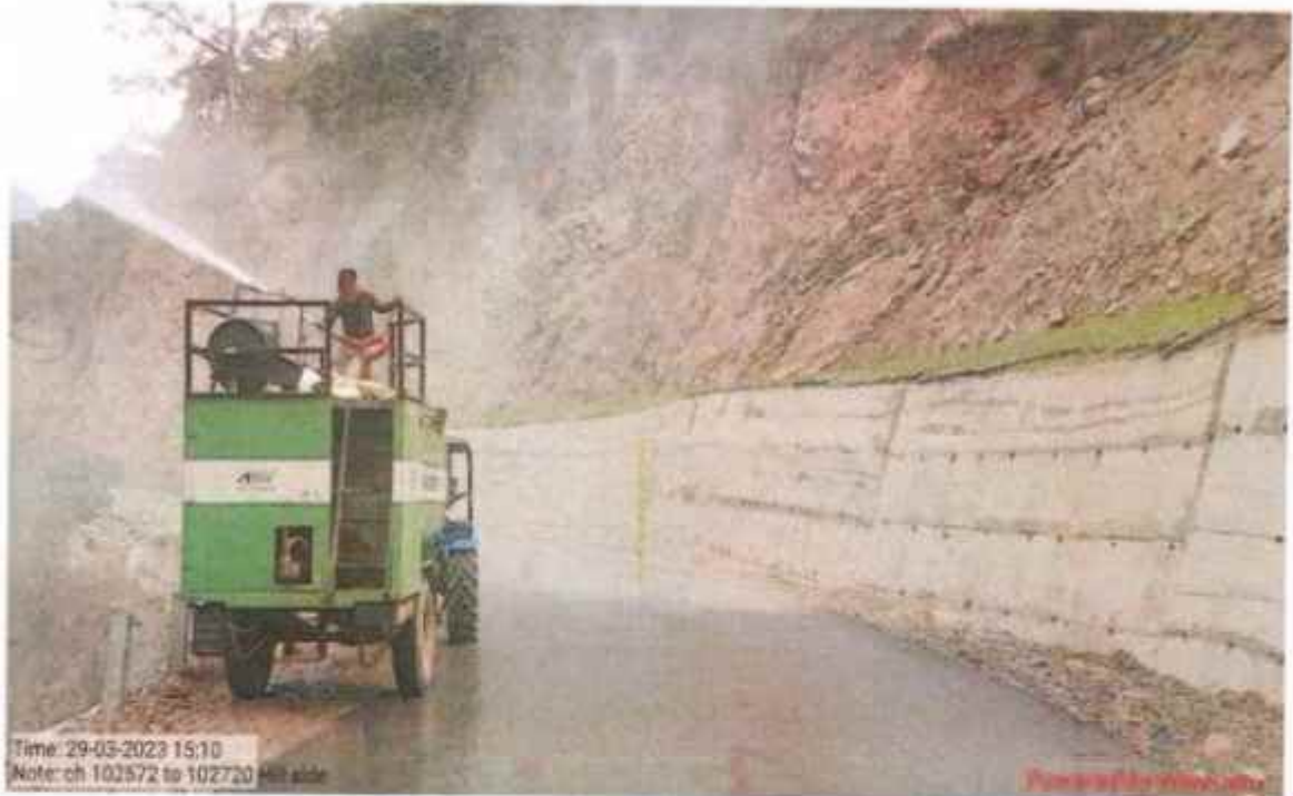
Geo cell with Hydro seeding work at km 102+572 to 102+720
