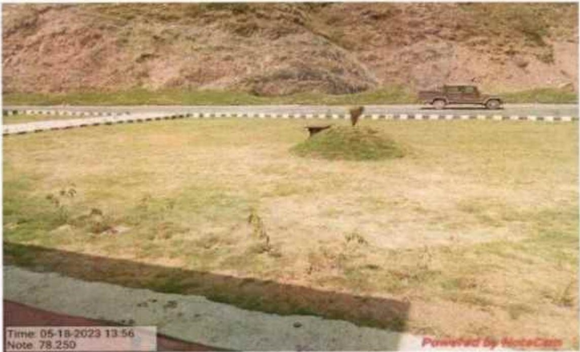
Valley side Bio-Engineering work at km 78+250
