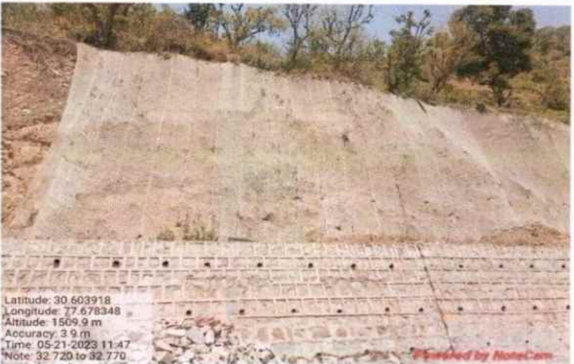
Coco fibre work at km 32+720 to 32+770
