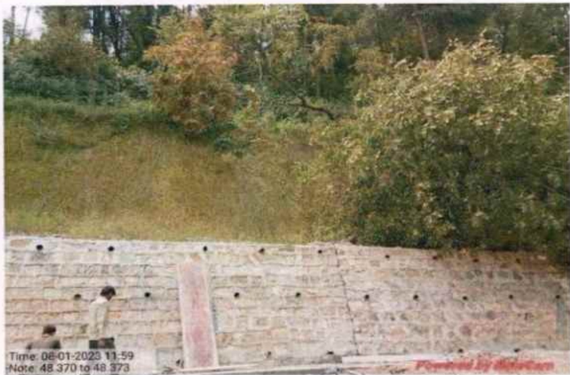
Interlink chain mesh work at km 48+370 to 48.373
