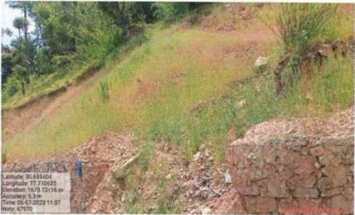
Hydro seeding work at km 67+970
