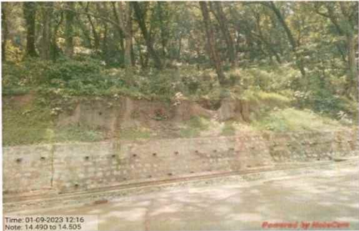
Coco fibre work at km 14+490 to 14.505
