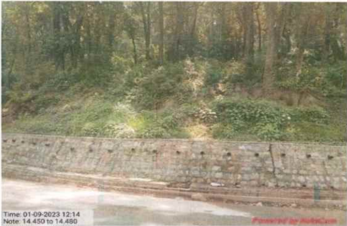
Coco fibre work at km 14.450 to 14.480
