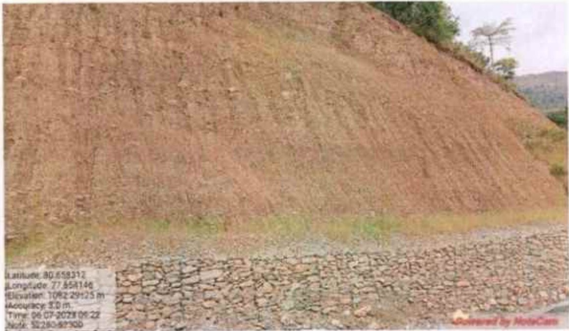
Hydro seeding work at km 52+280 to 52+300
