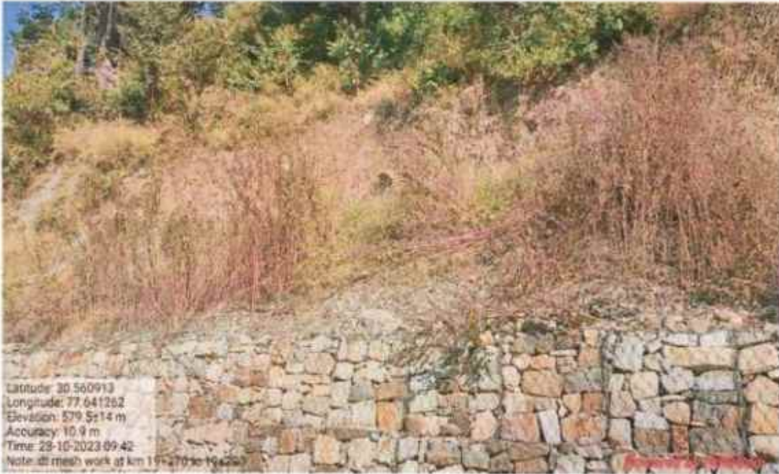
hydro seeding at km 19+270 to 19+290
