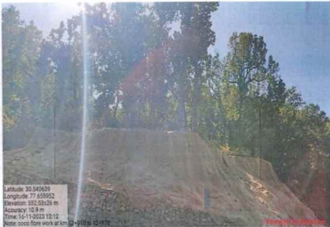
Coco fibre work at km 12+910 to 12+970
