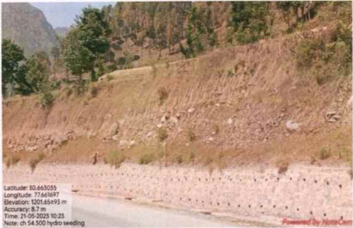
Hydro seeding work at km 54+300
