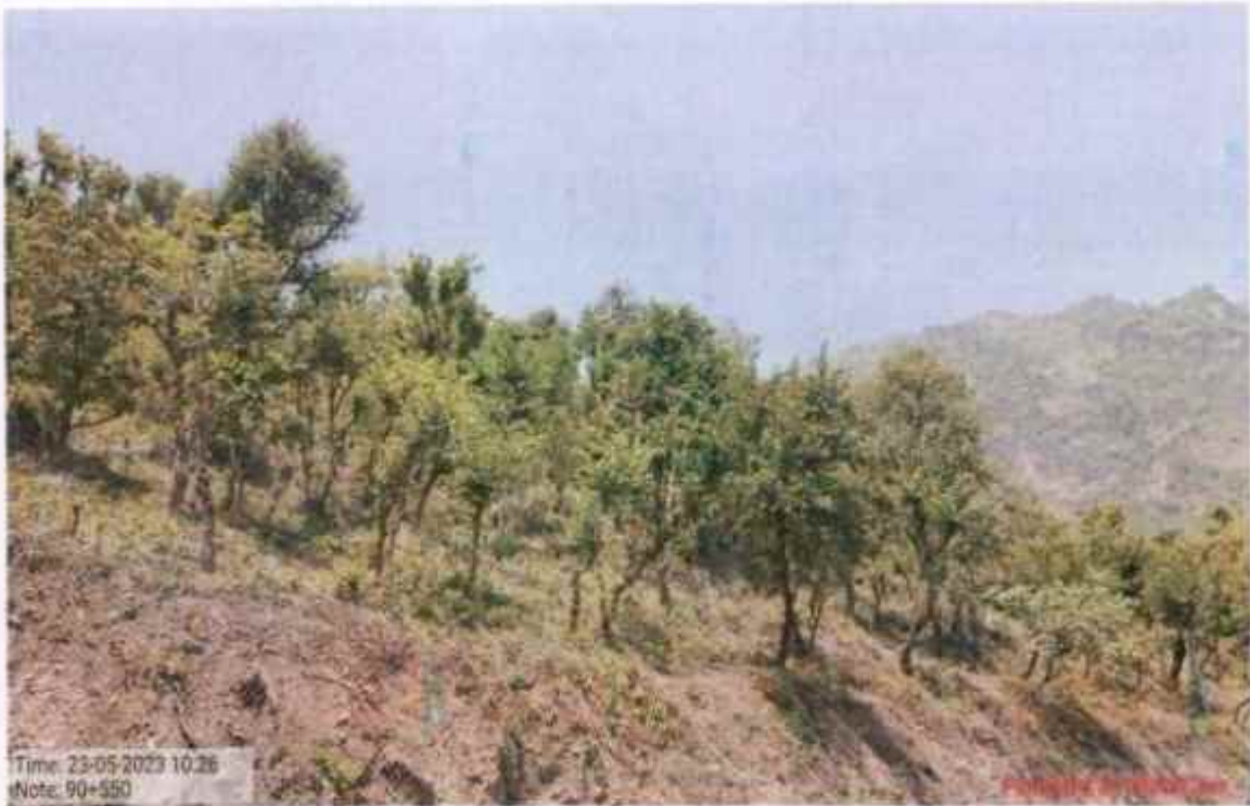
Interlink chain mesh work at km 90+550
