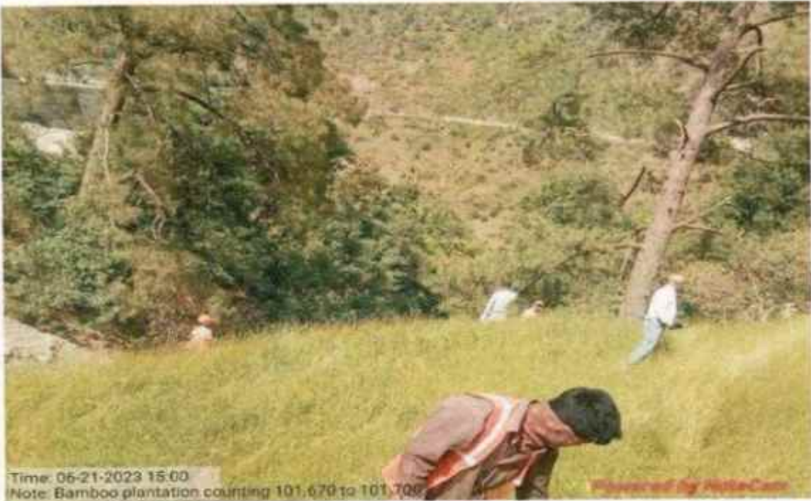
Valley side Geo cell with Hydro seeding and Bamboo plantation work at km 101+670 to 101+700
