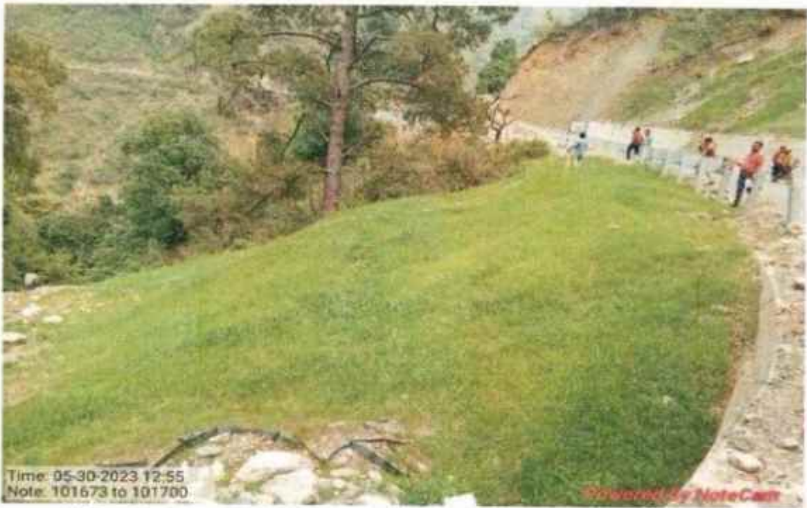
Valley side Geo cell with Hydro seeding and Bamboo plantation work at km 101+673 to 101+700
