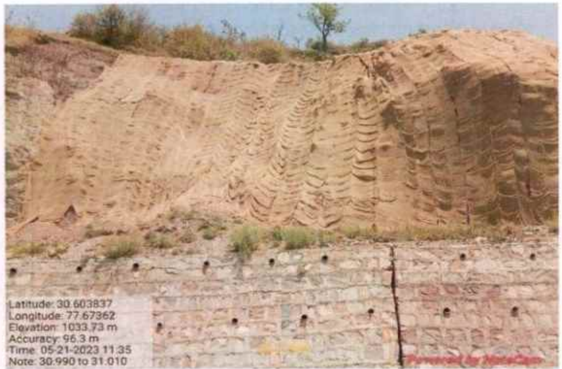
Coco fibre work at km 30+990 to 31+010
