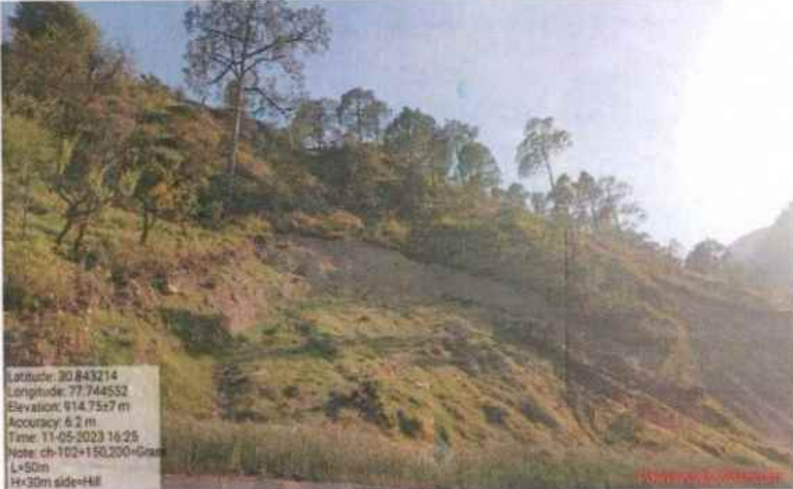
Hydro seeding and Geo cell with Hydro seeding work at km 102+150 to 102+200
