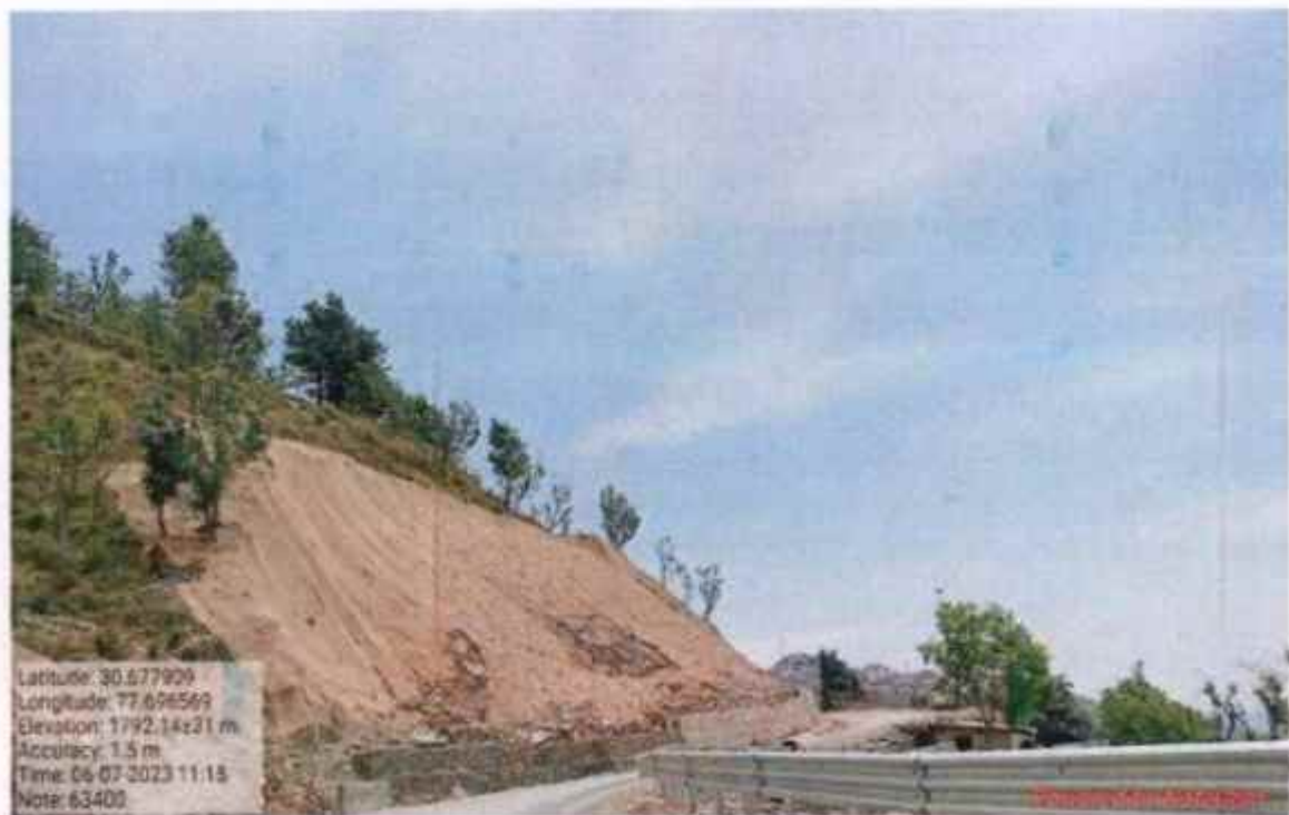
Shotcrete Crib wall work at km 63+400
