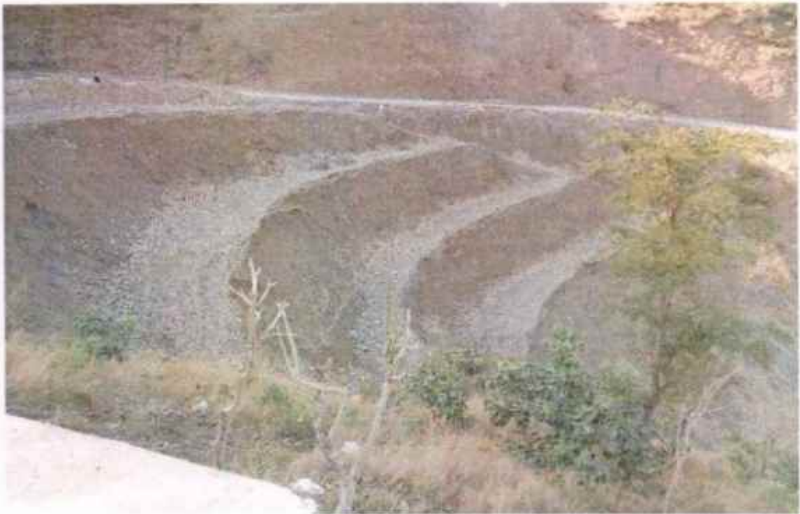
Valley side Bio-Engineering work at km 83+250
