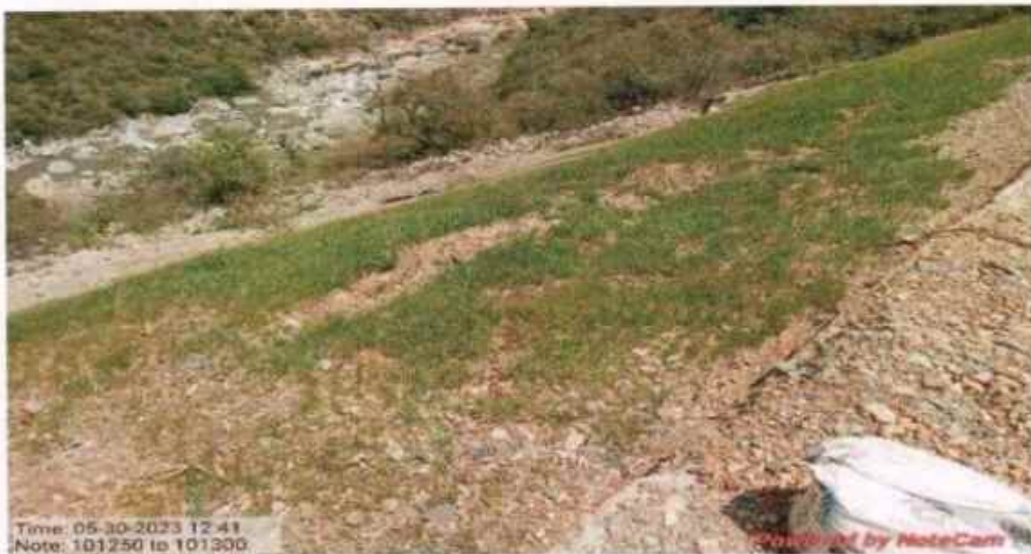
Valley side Geo cell with Hydro seeding and Bamboo plantation work at km 101+250 to 101+300
