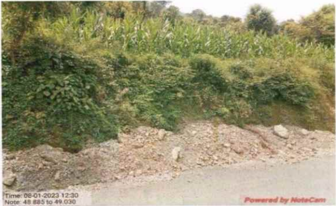
Interlink chain mesh work at km 48+855 to 49+030
