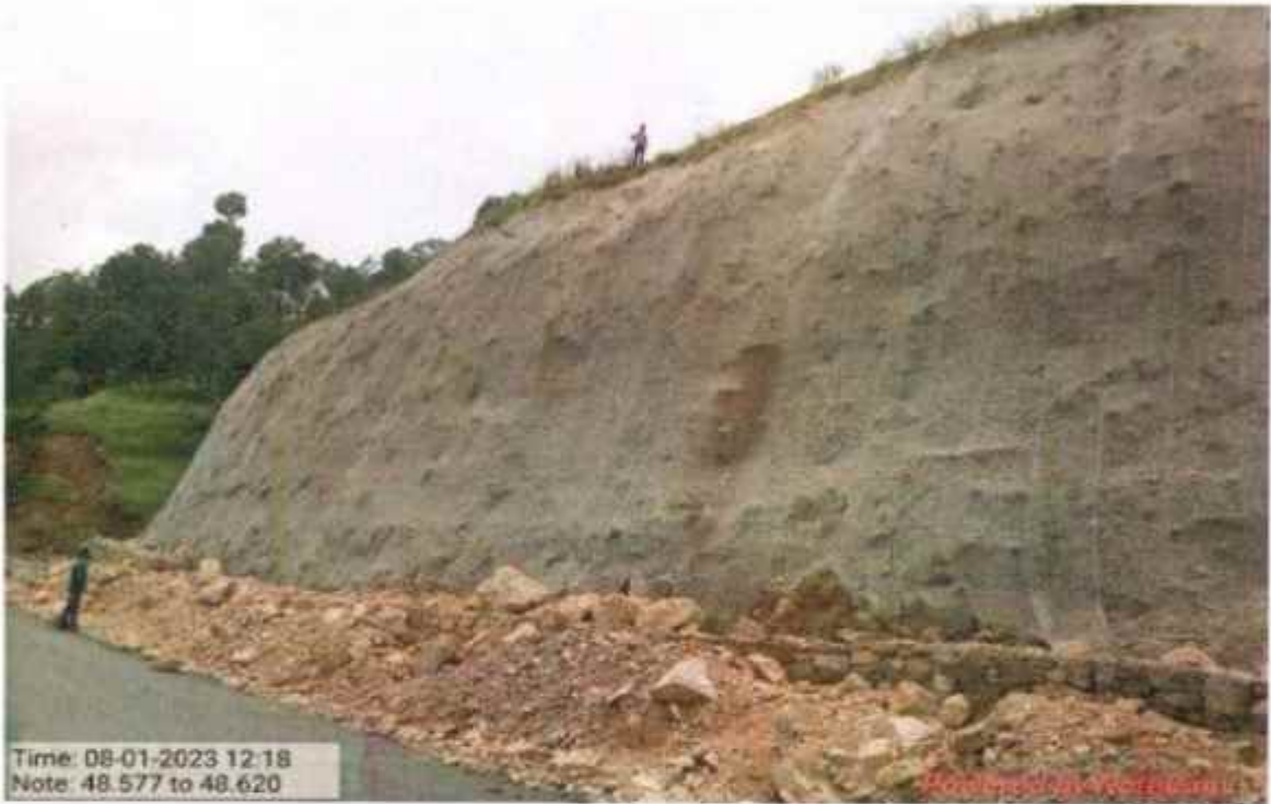
Interlink chain mesh work at km 48+577 to 48+620
