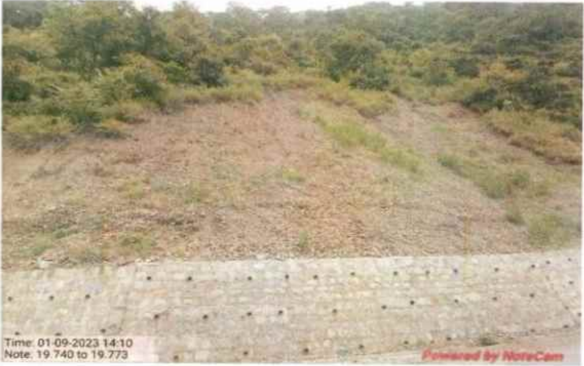
Interlink chain mesh work at km 19+740 to 19+773
