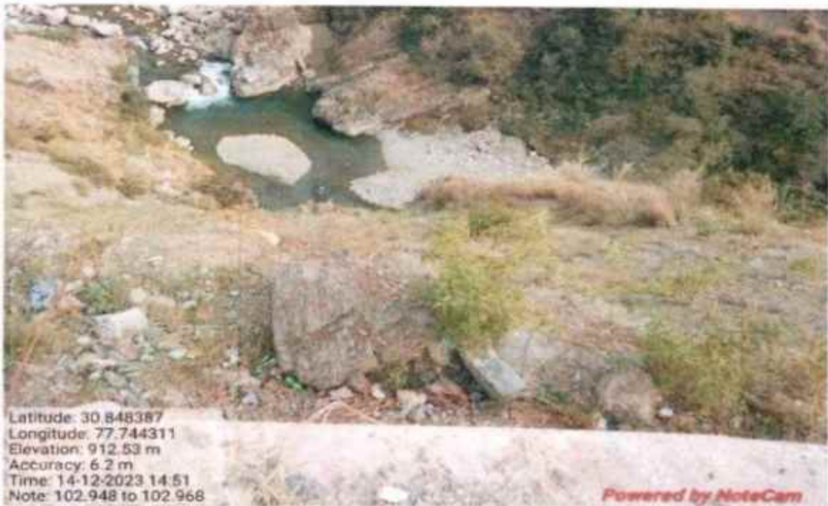
Valley side Bamboo plantation work at km 102+948 to 102+968
