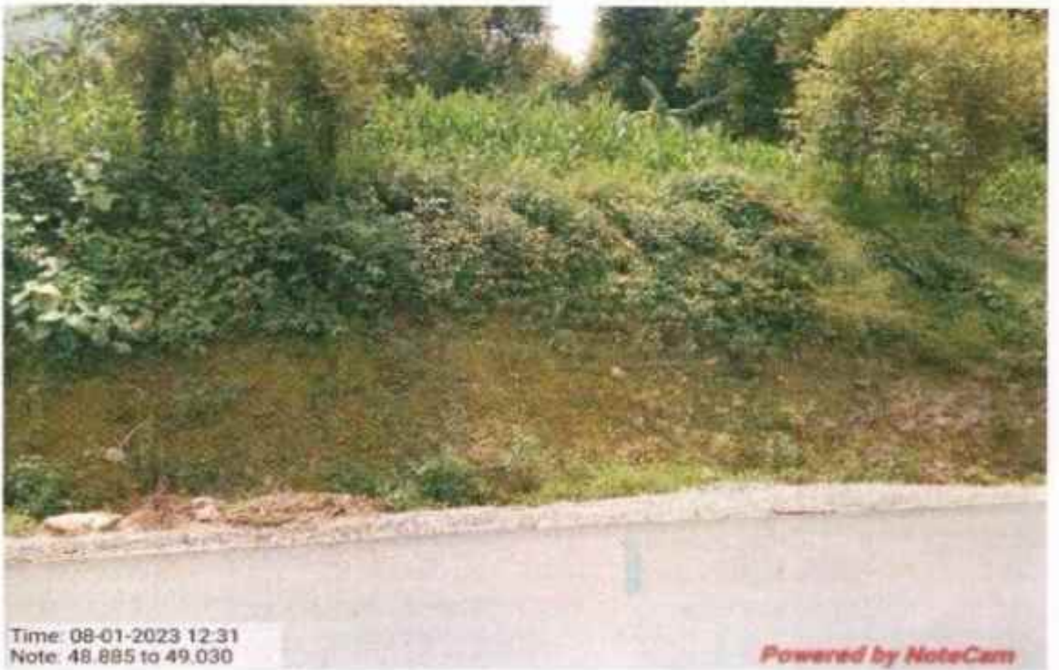
Interlink chain mesh work at km 48+855 to 49+030
