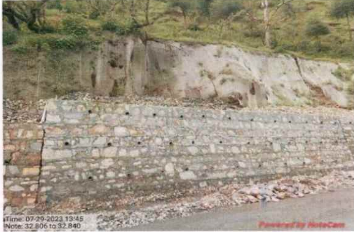
Coco fibre work at km 32+806 to 32+840
