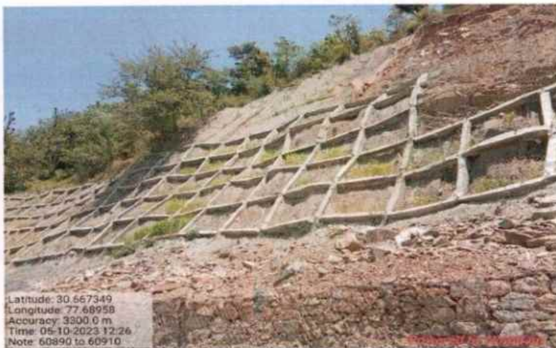
Shotcrete Crib wall work at km 60+910
