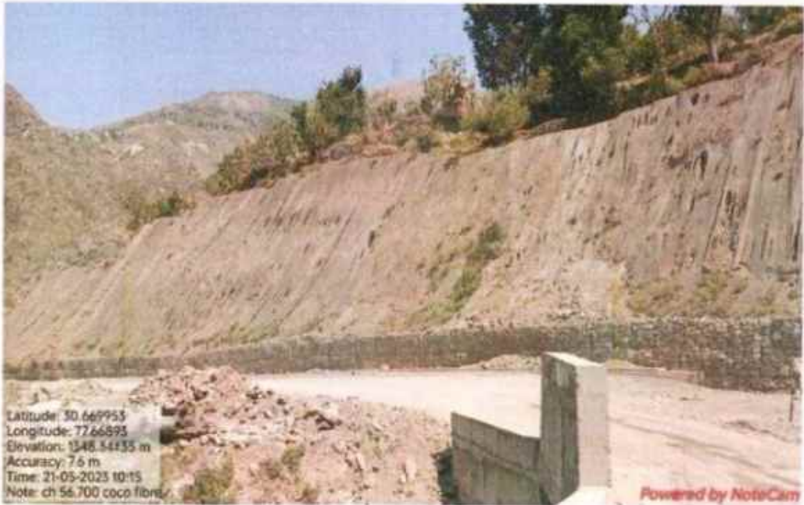
Coco fibre with Grass work at km 56+700
