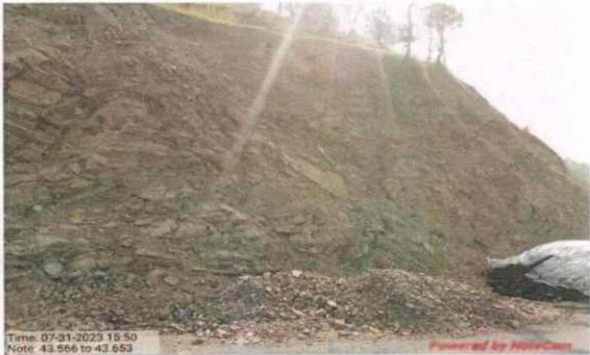
Interlink chain mesh work at km 43+566 to 43+653
