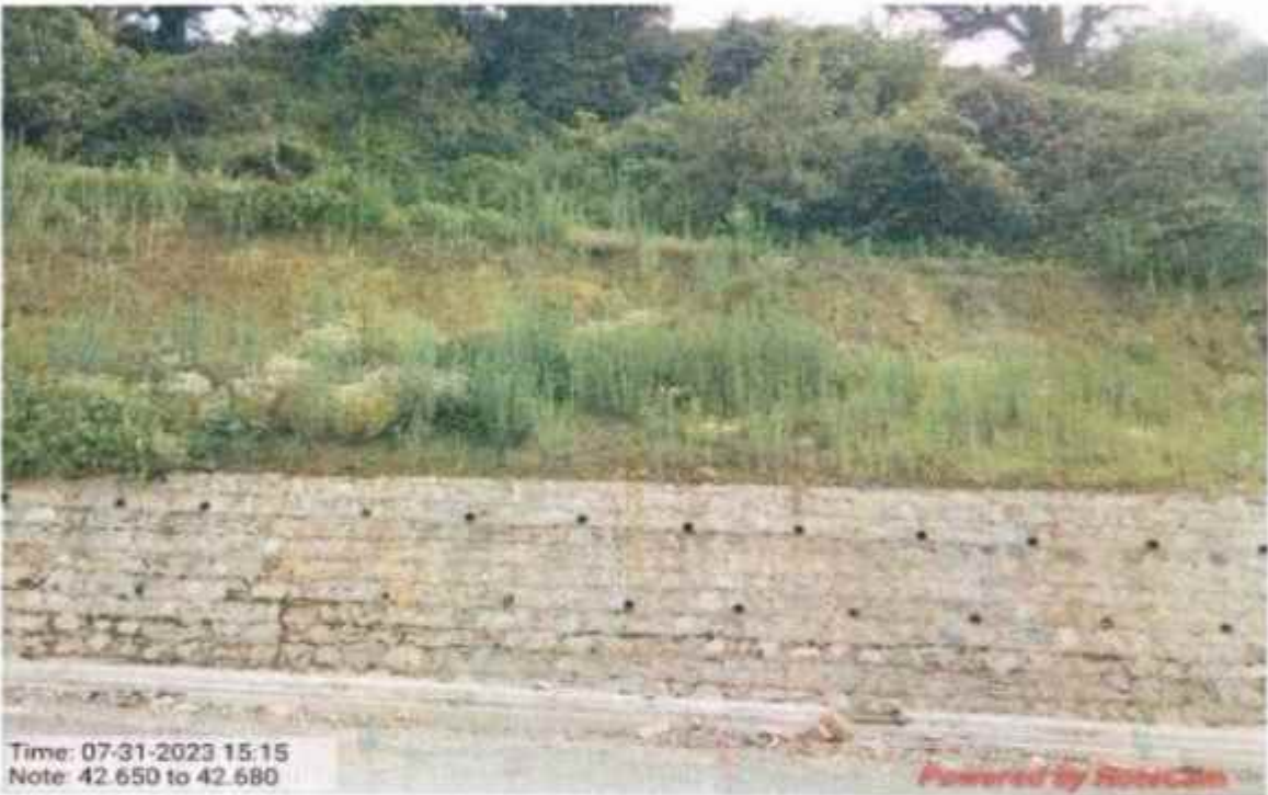
Interlink chain mesh work at km 42+650 to 42+680
