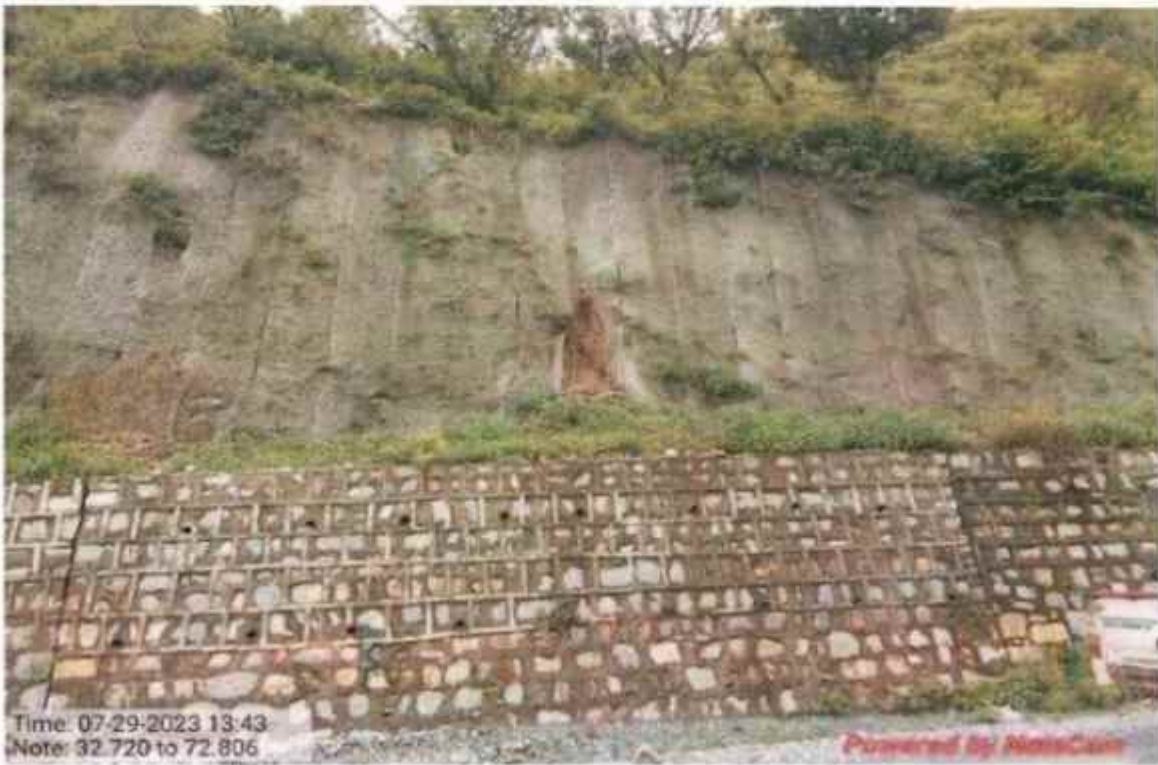
Coco fibre work at km 32+720 to 32+806
