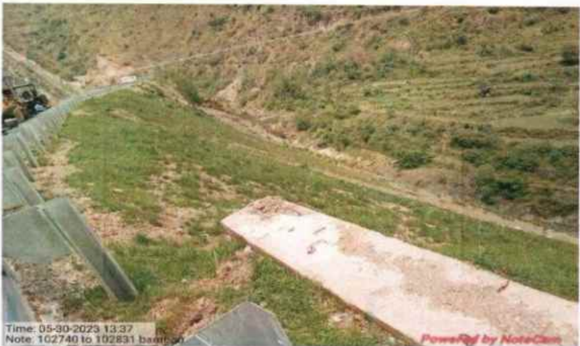
Valley side Geo cell with Hydro seeding and Bamboo plantation work at km 102+740 to 102+831
