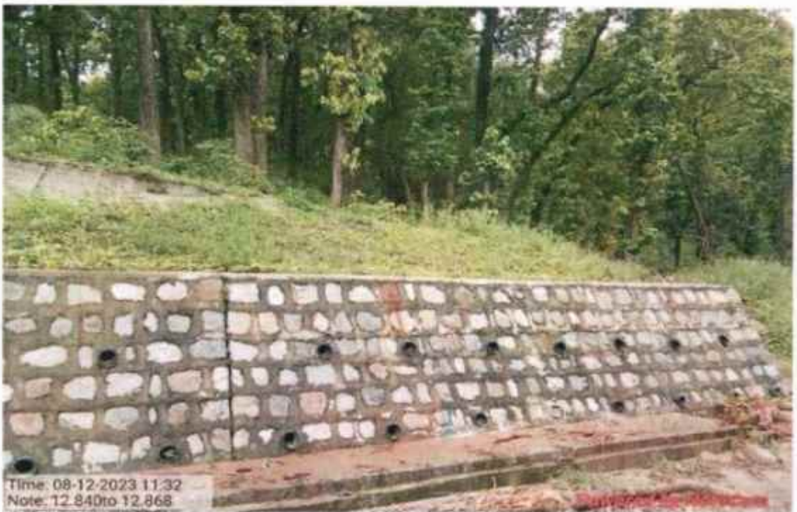
Coco fibre work at km 12+840 to 12+868
