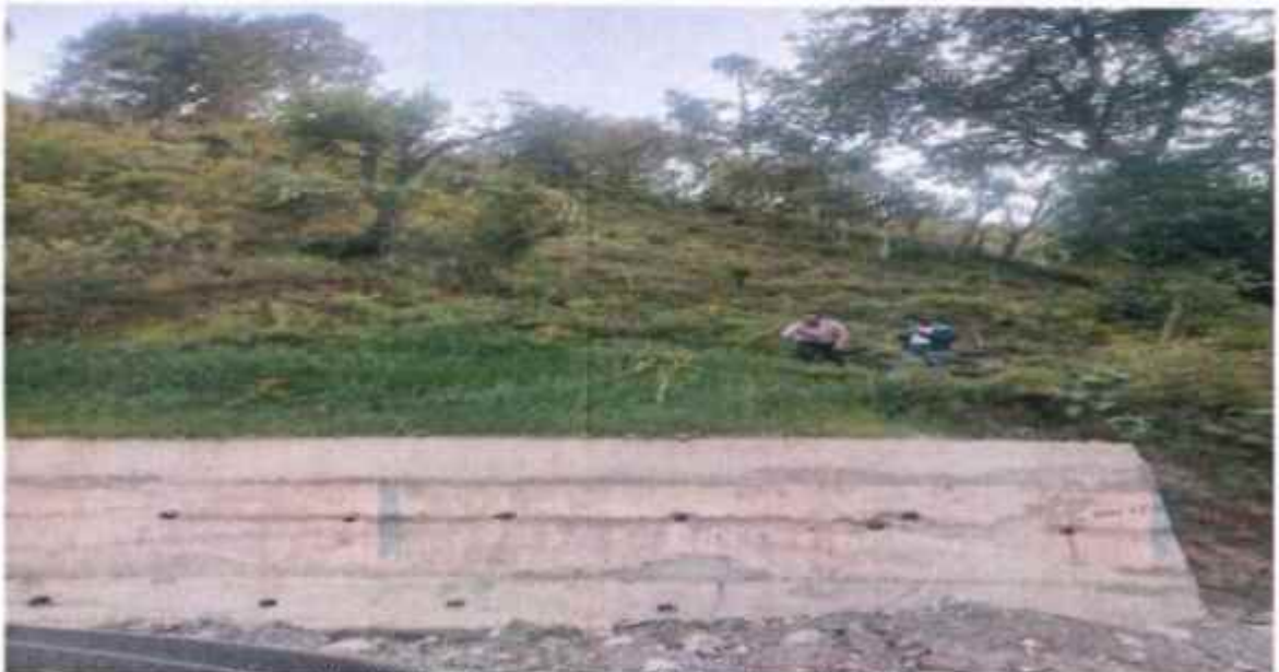
Geo cell with Hydro seeding and Bamboo plantation work
