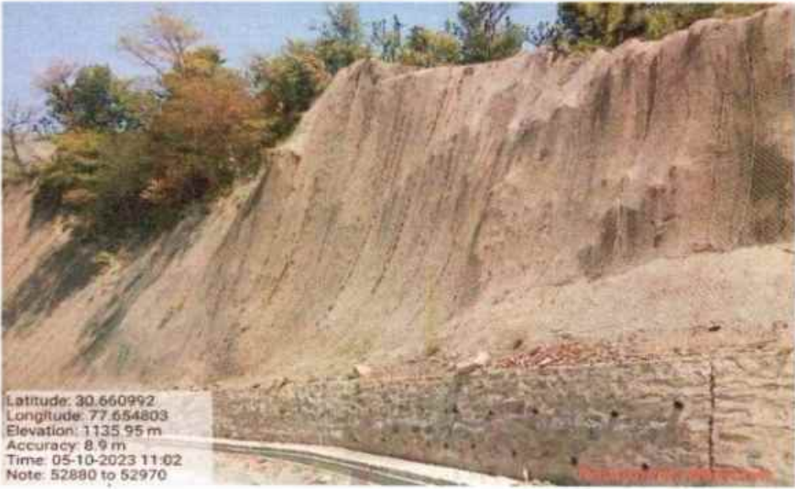
Interlink chain mesh work at km 52+880 to 52+970
