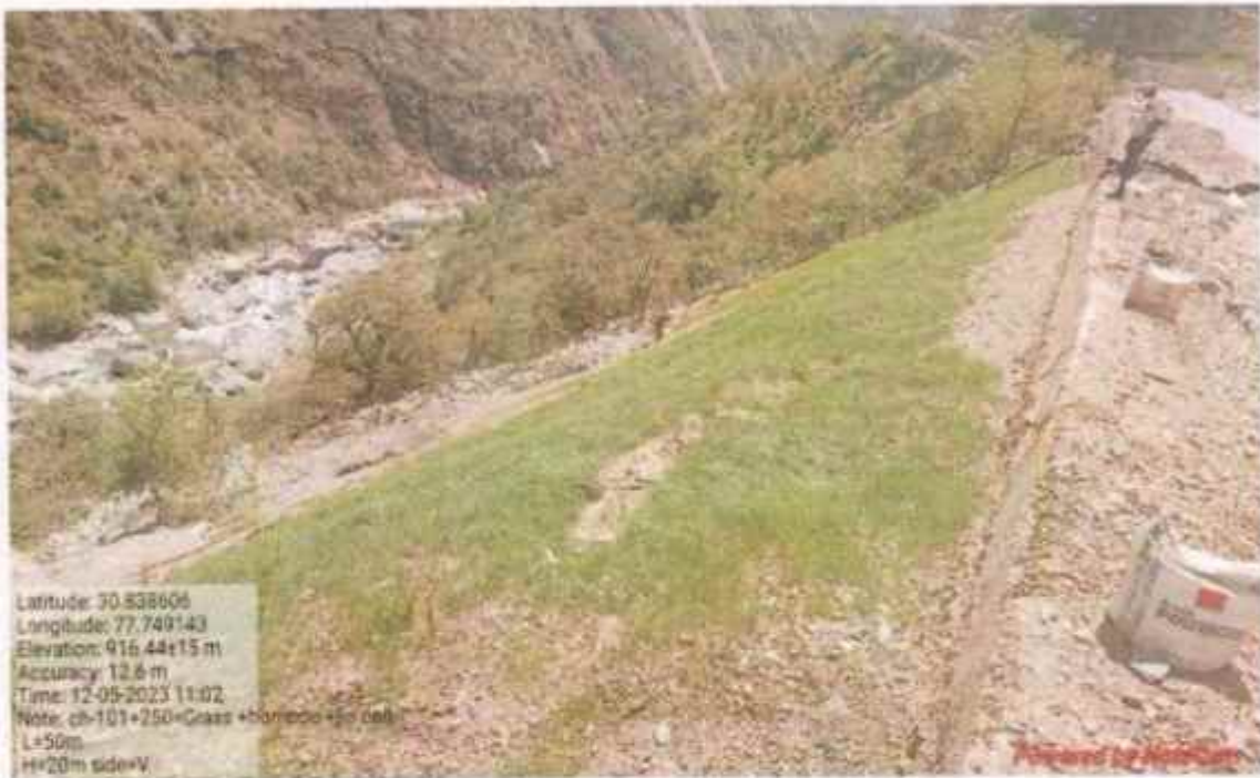
Valley side Geo cell with Hydro seeding and Bamboo plantation work at km 101+250
