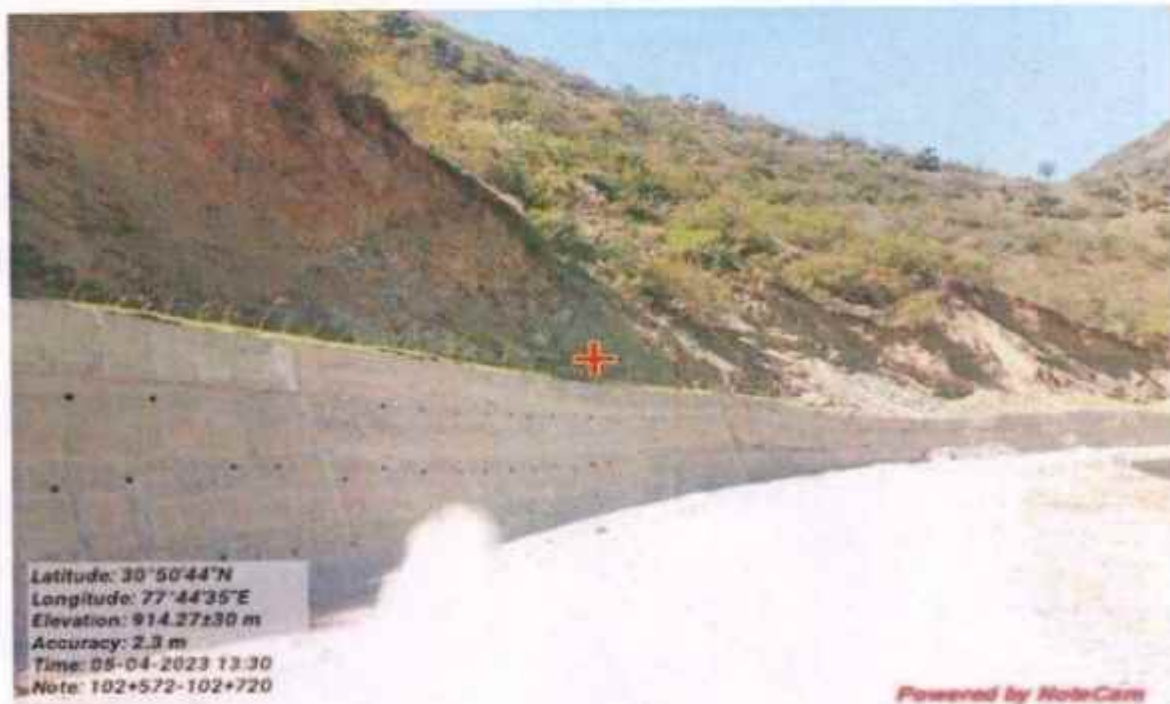
Geocell with Hydroseeding and Bamboo plantation work at km 102+572 to 102+720
