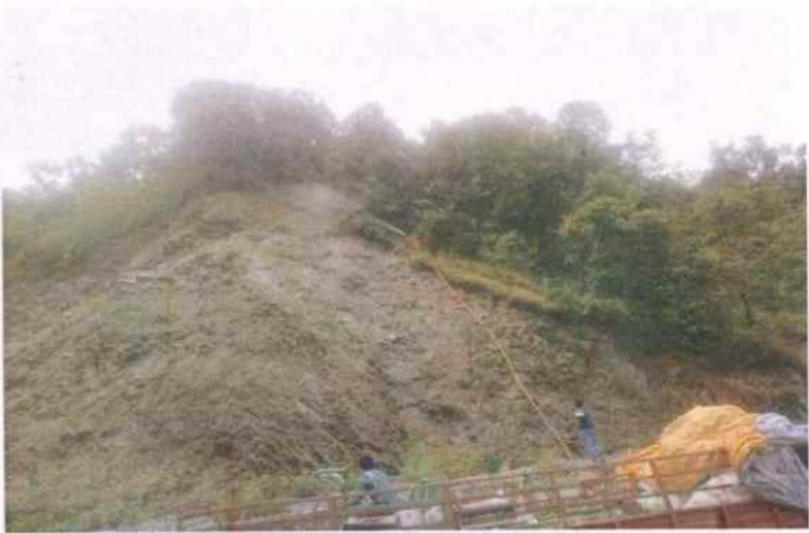
Hydro seeding watering
