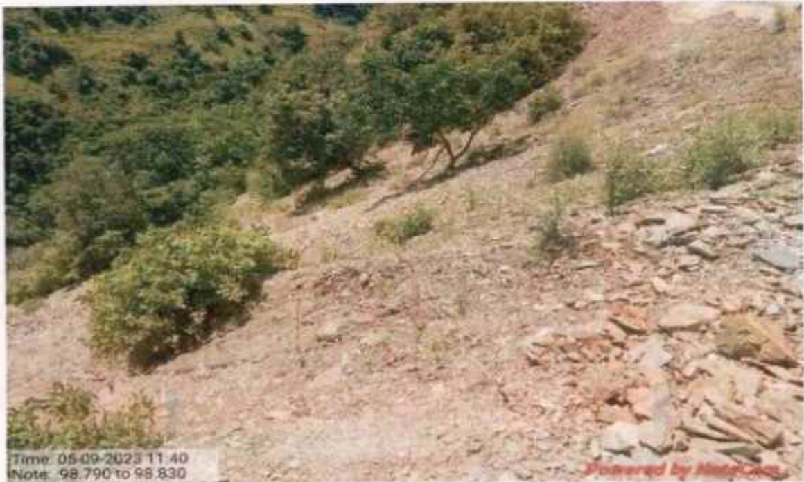
Valley side Bamboo plantation work at km 98+790 to 98+830
