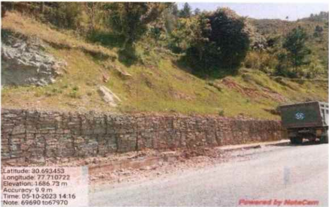
Hydro seeding work at km 69+690 to 69+970
