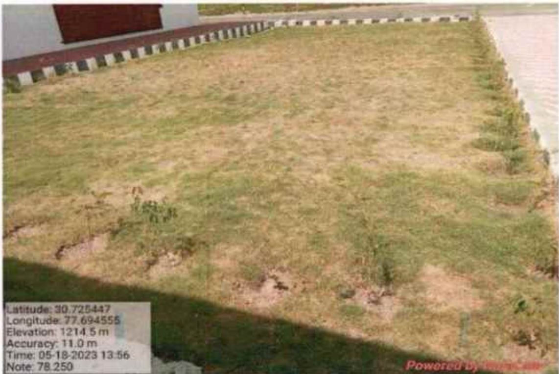
Valley side Bio-Engineering work at km 78+250
