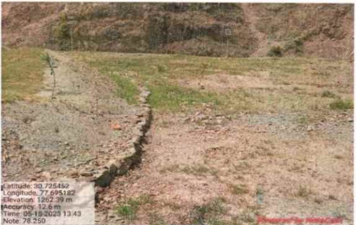
Valley side Bio-Engineering work at km 78+250
