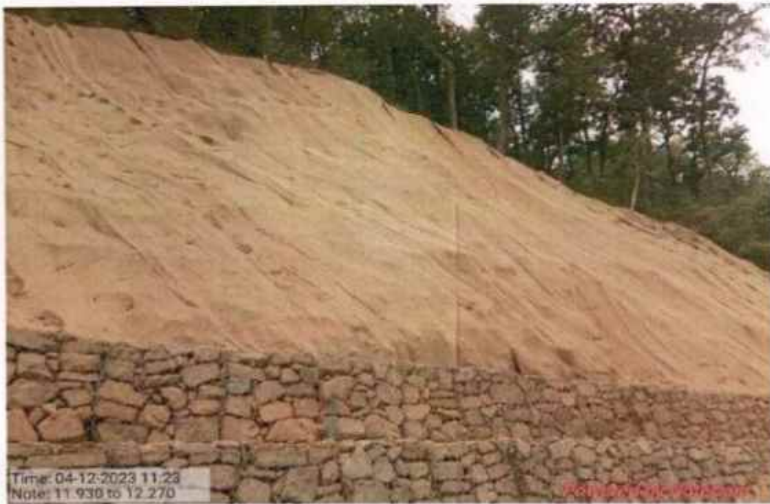
Coco fibre work at km 11+930 to 12+270
