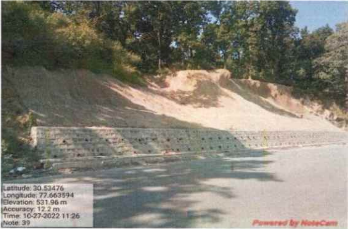
Coco fibre work at km 11+882 to 11+930
