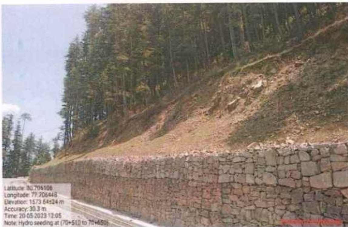
Hydro seeding work at km 70+510 to 70+650
