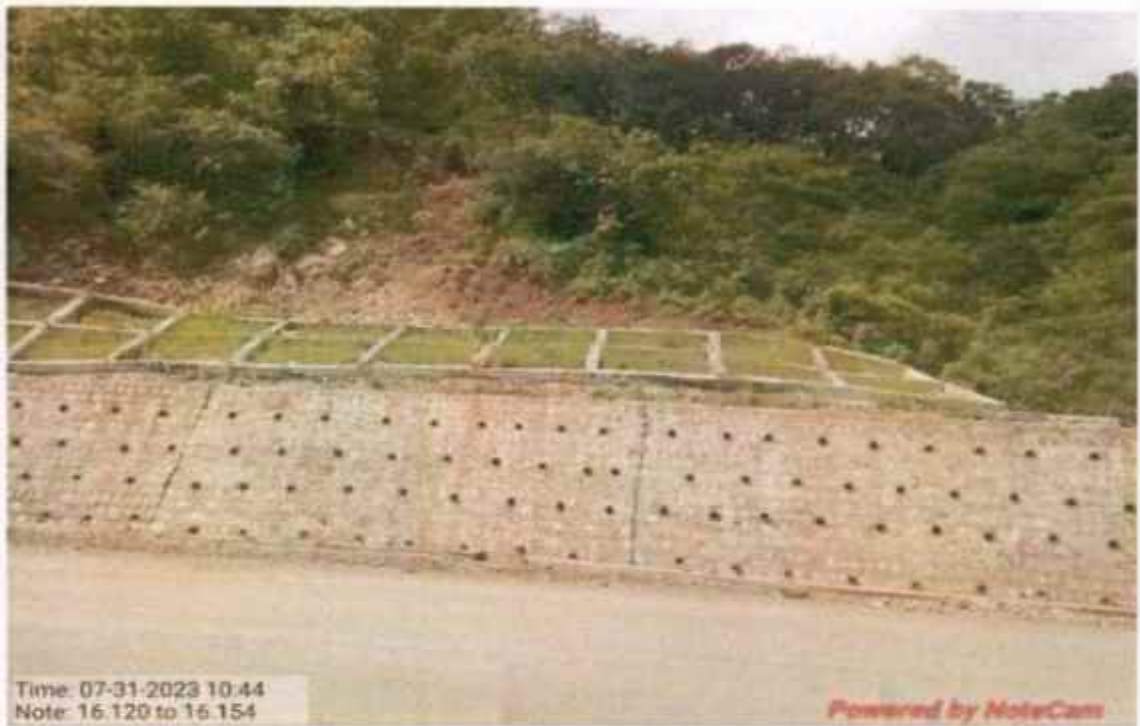
Shotcrete crib wall work at km 16+120 to 16.154
