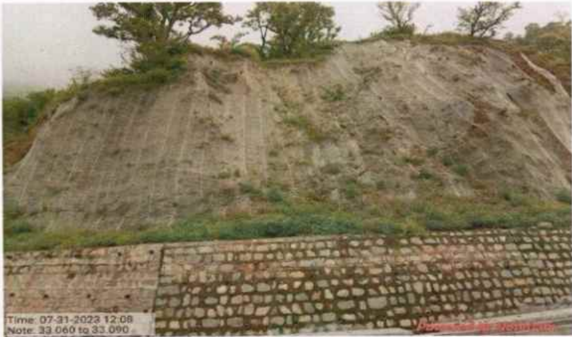
Coco fibre work at km 33+060 to 33+090
