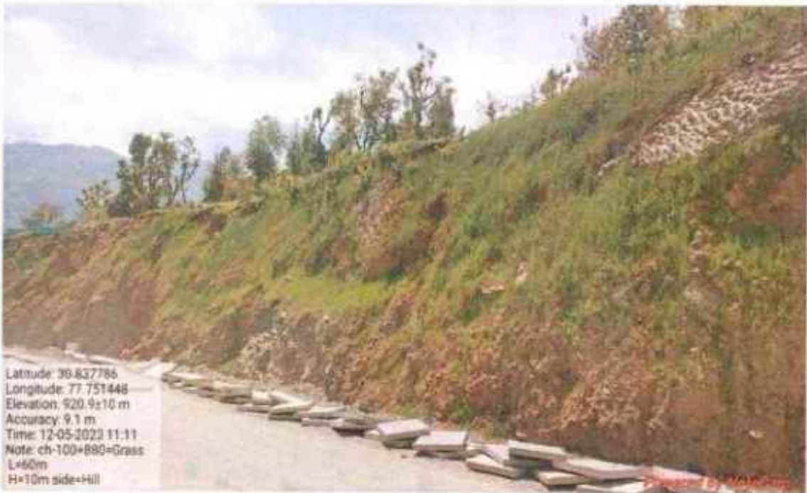
Hydro seeding work at km 100+880
