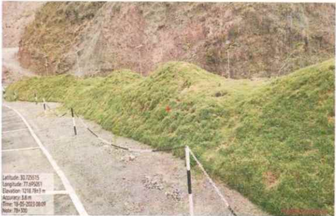
Valley side Bio-Engineering work at km 78+250
