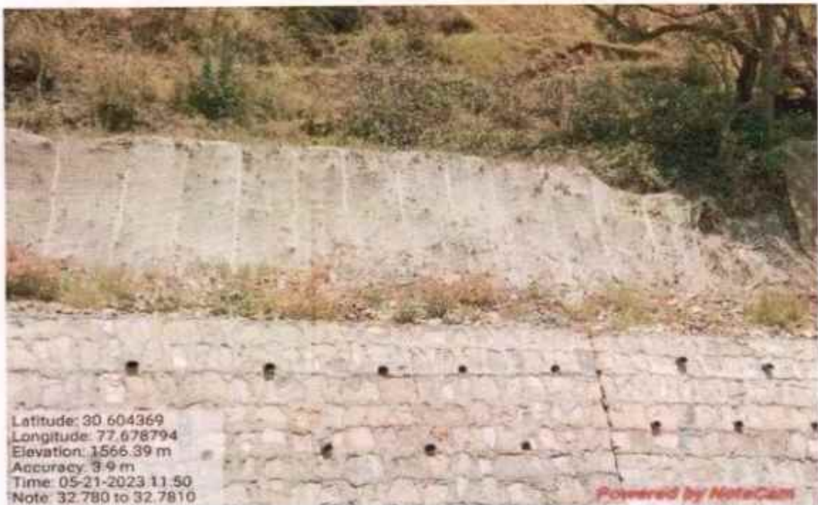
Coco fibre work at km 32+780 to 32+810
