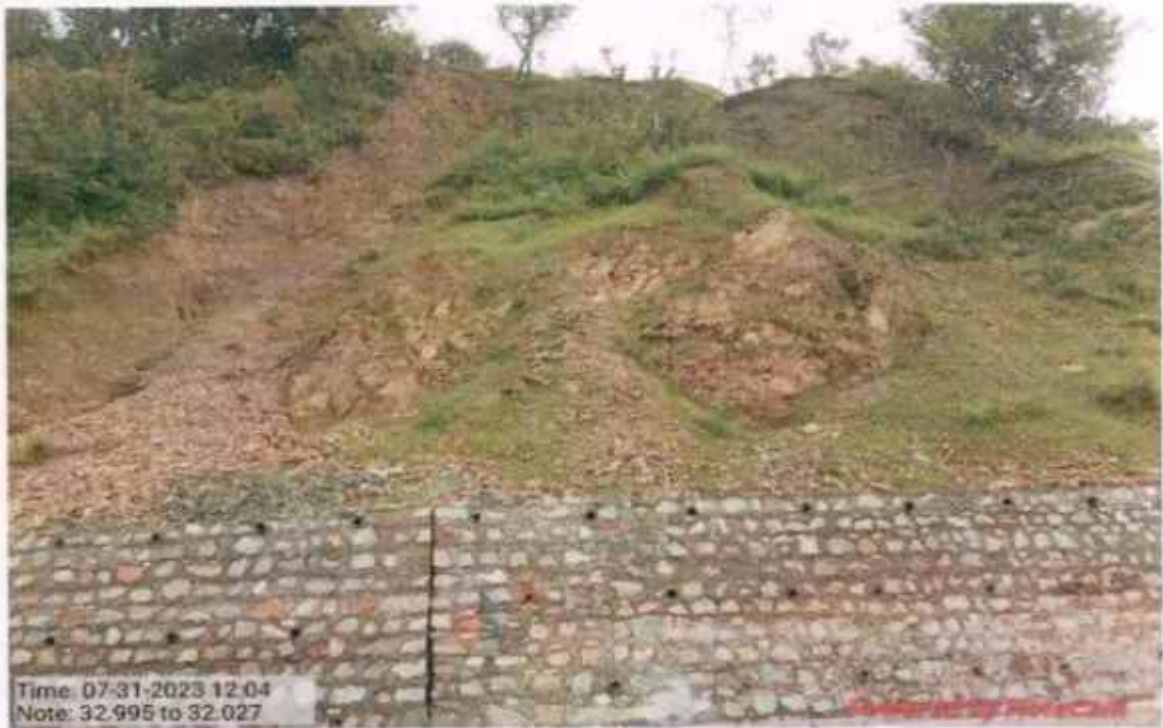
Hydro seeding work at km 32+995 to 32+027
