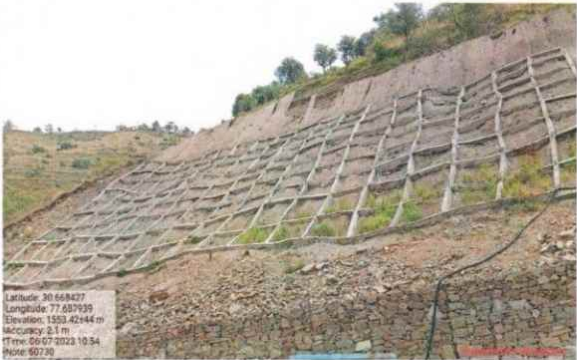
Shotcrete Crib wall work at km 60+730
