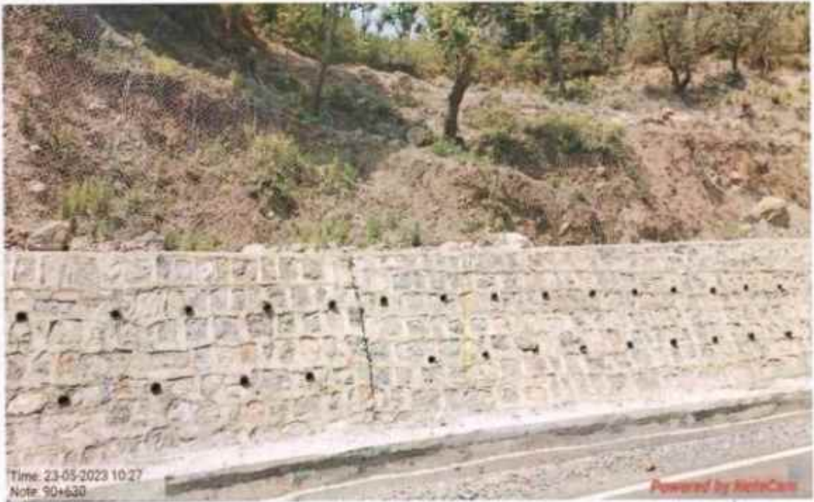
Interlink chain mesh work at km 90+630
