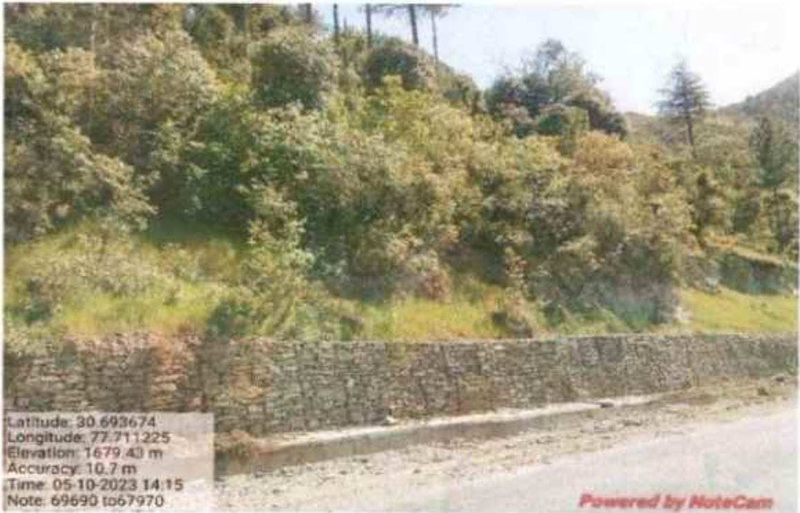
Hydro seeding work at km 69+690 to 69+970
