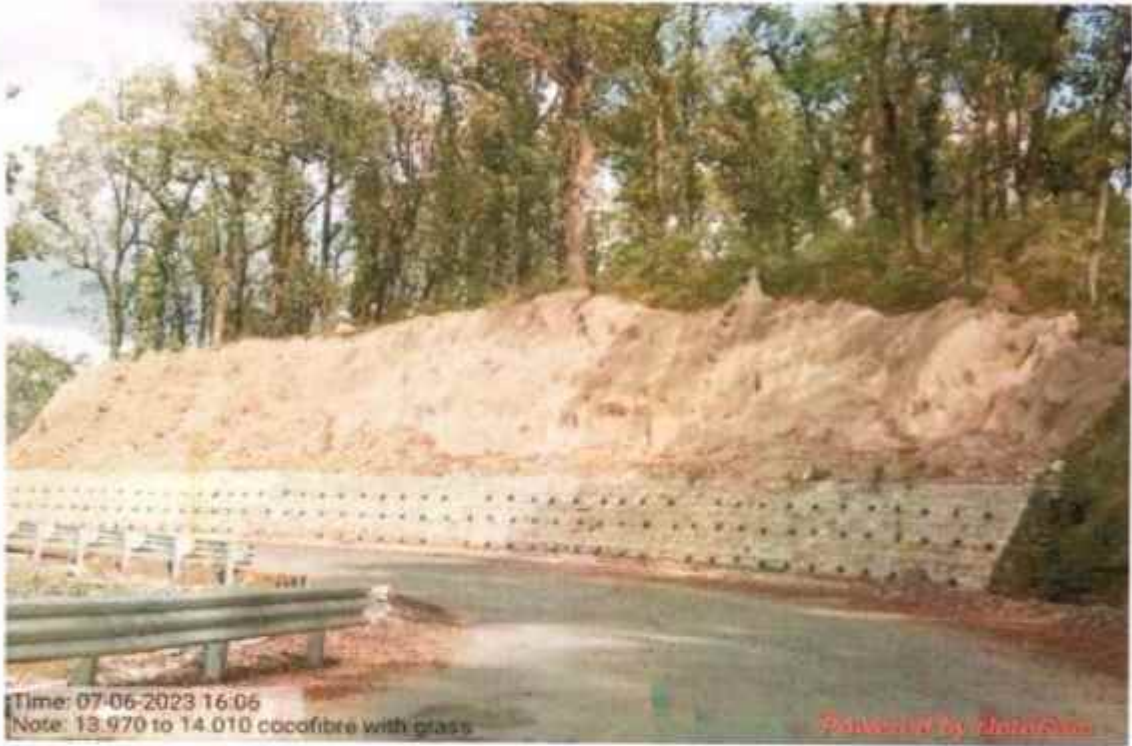
Coco fibre work at km 13+970 to 14.010
