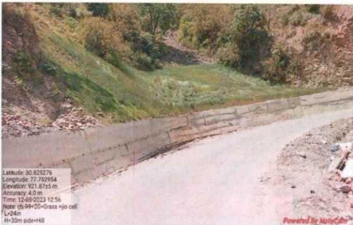
Hydro seeding and Geo cell with Hydro seeding work at km 99+120
