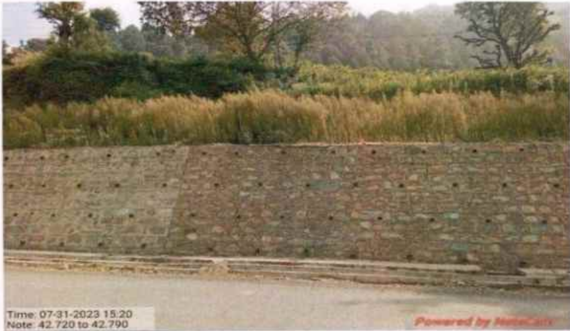
Interlink chain mesh work at km 42+720 to 42+790
