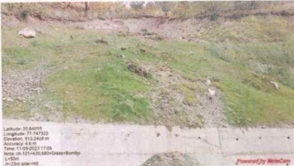
Hydro seeding work at km 101+630 to 101+680
