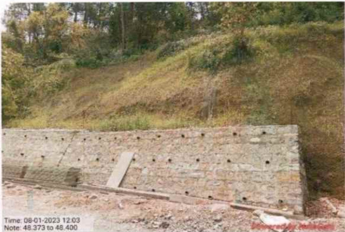
Interlink chain mesh work at km 48+373 to 48+400
