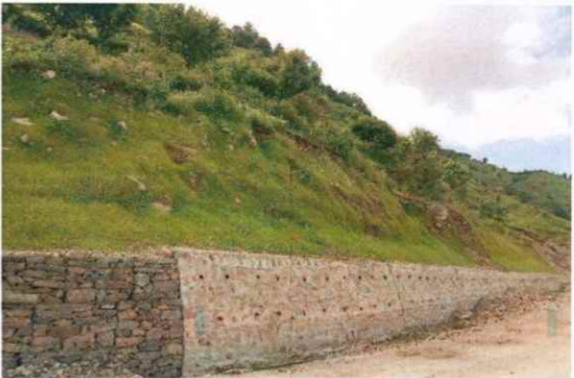
Hydro seeding work
