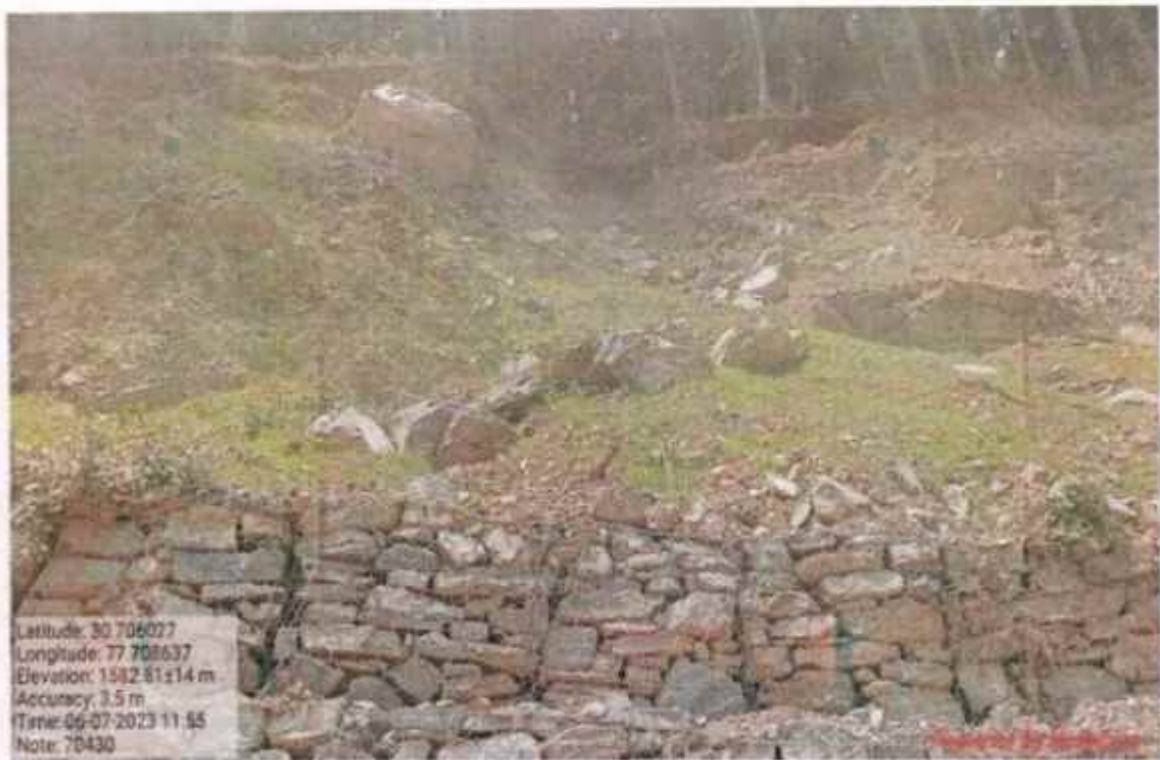
Hydro seeding work at km 70+430
