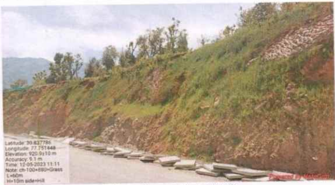
Hydro seeding work at km 100+880
