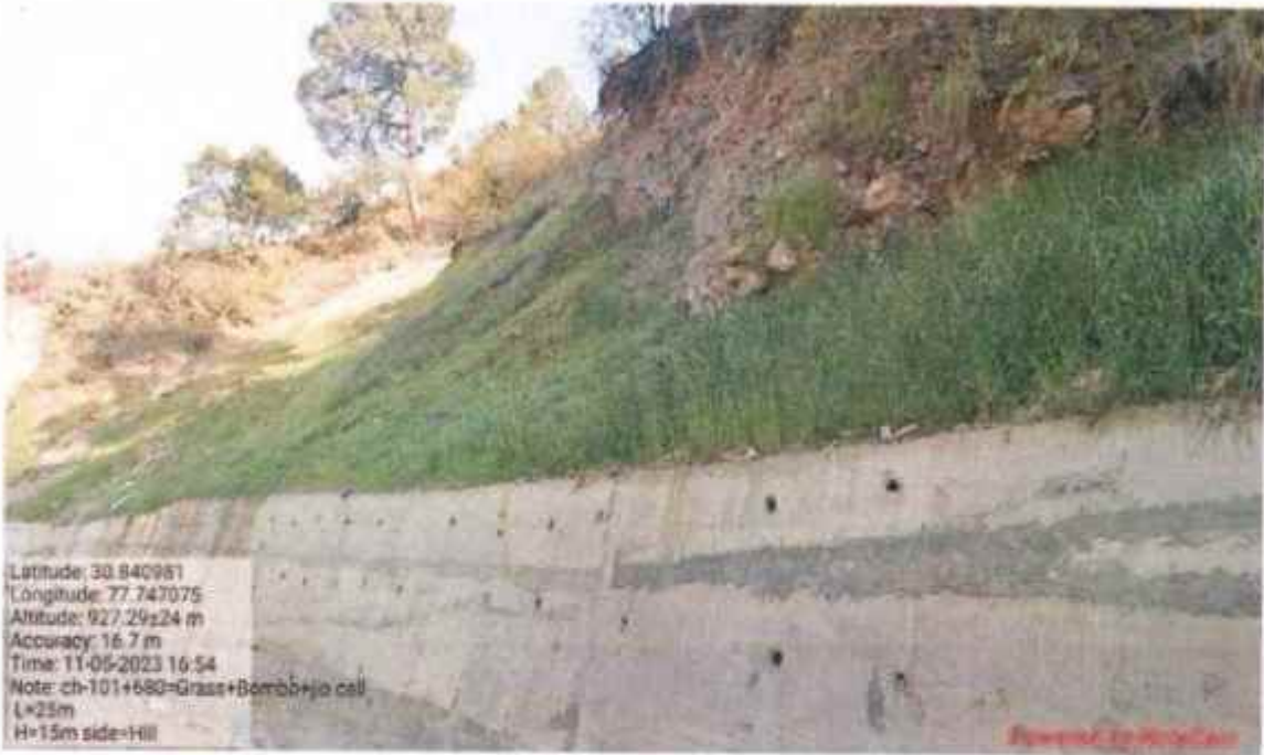
Hydro seeding and Geo cell with Hydro seeding work at km 101+680
