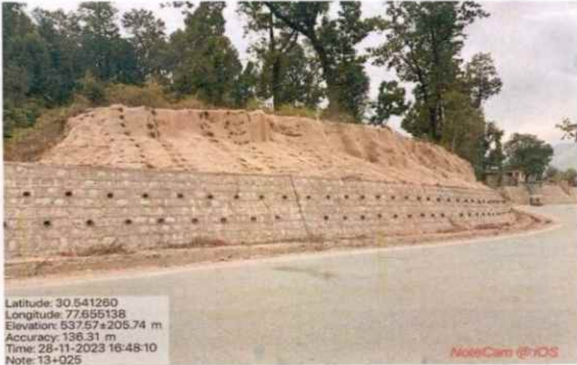
Coco fibre work at km 13+025
