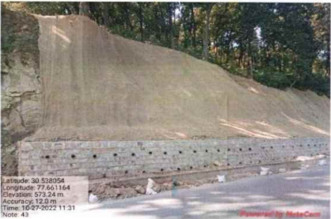
Coco fibre work at km
