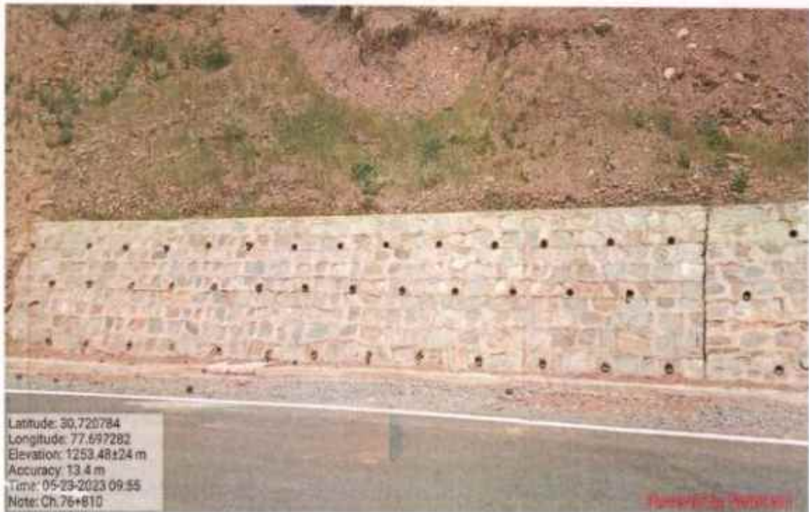
Interlink chain mesh work at km 76+810
