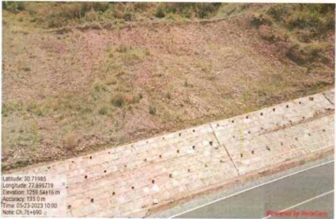
Interlink chain mesh work at km 76+690
