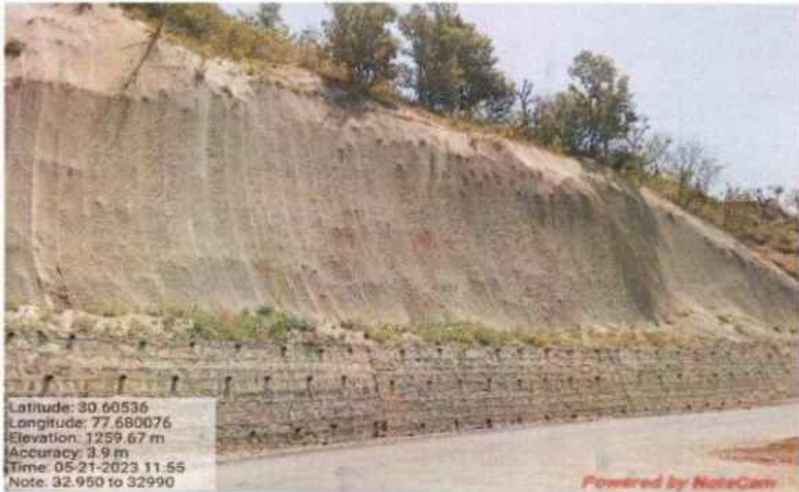
Coco fibre work at km 32+950 to 32+990
