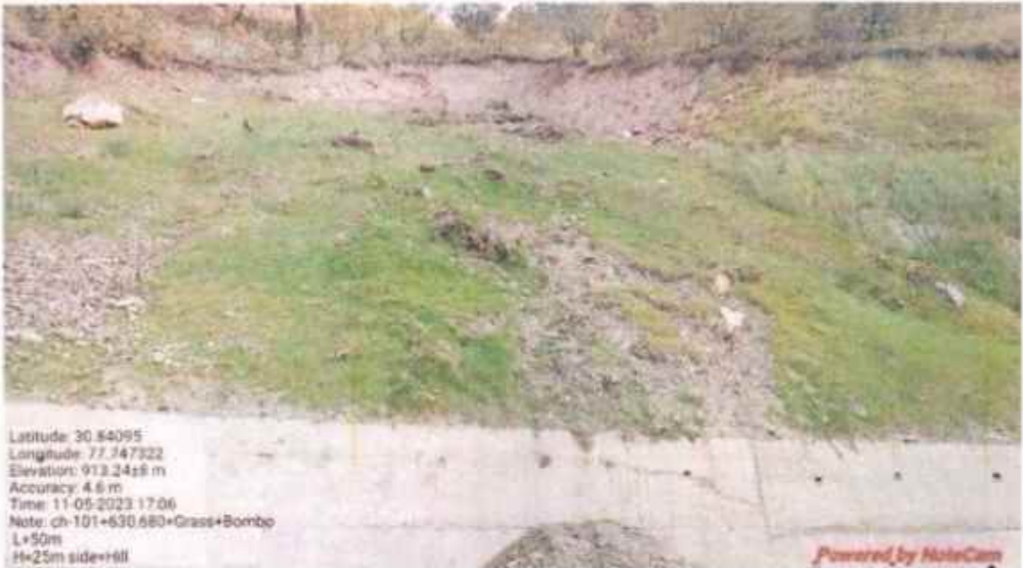
Hydro seeding work at km 101+630 to 101+680
