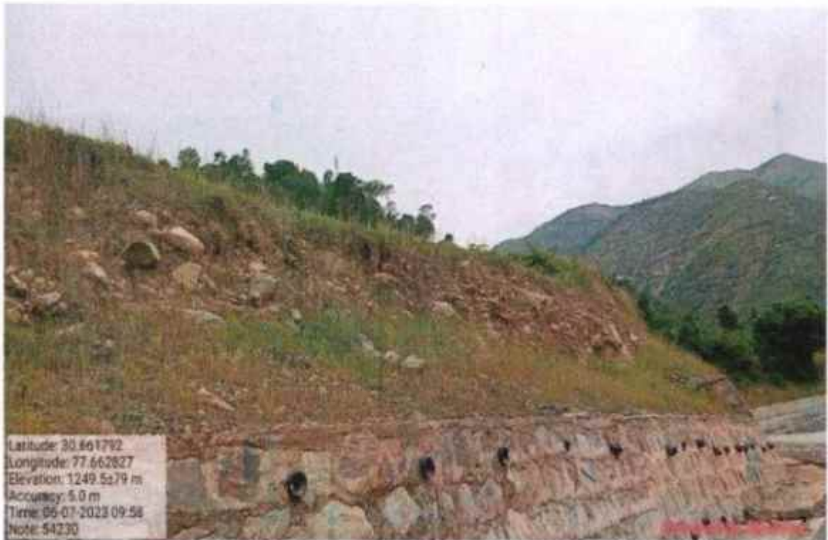
Hydro seeding work at km 54+230
