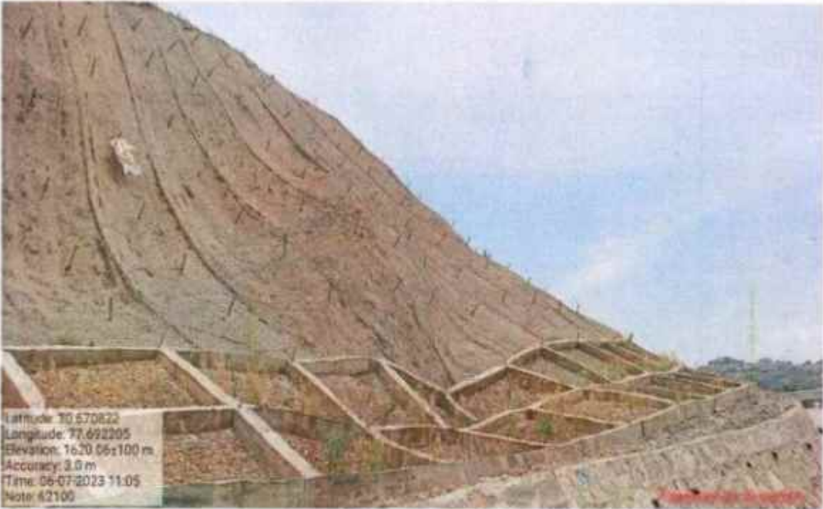
Shotcrete Crib wall work at km 62+100
