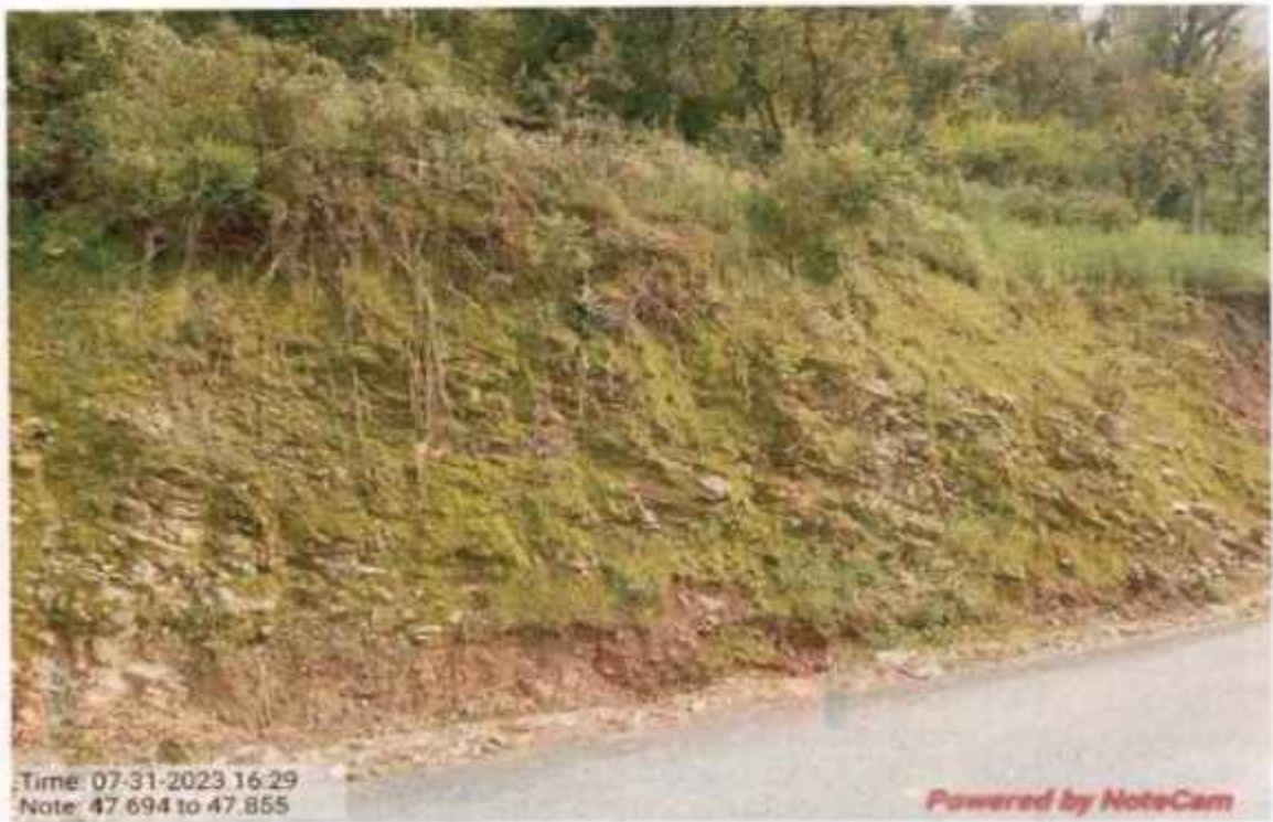
Hydro seeding work at km 47+694 to 47+855
