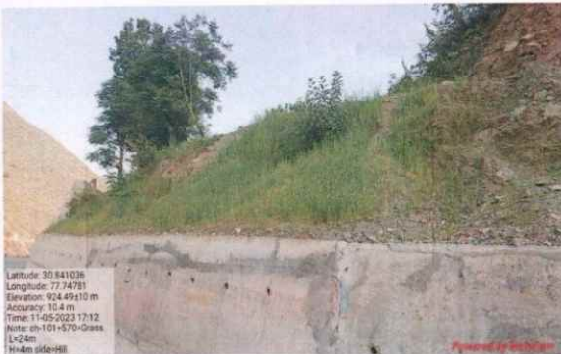
Hydro seeding work at km 101+570
