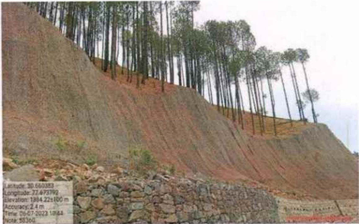
Interlink chain mesh work at km 58+360
