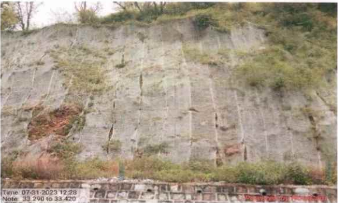
Coco fibre work at km 33+290 to 33+420
