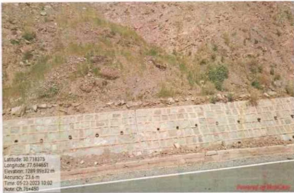
Interlink chain mesh work at km 76+450
