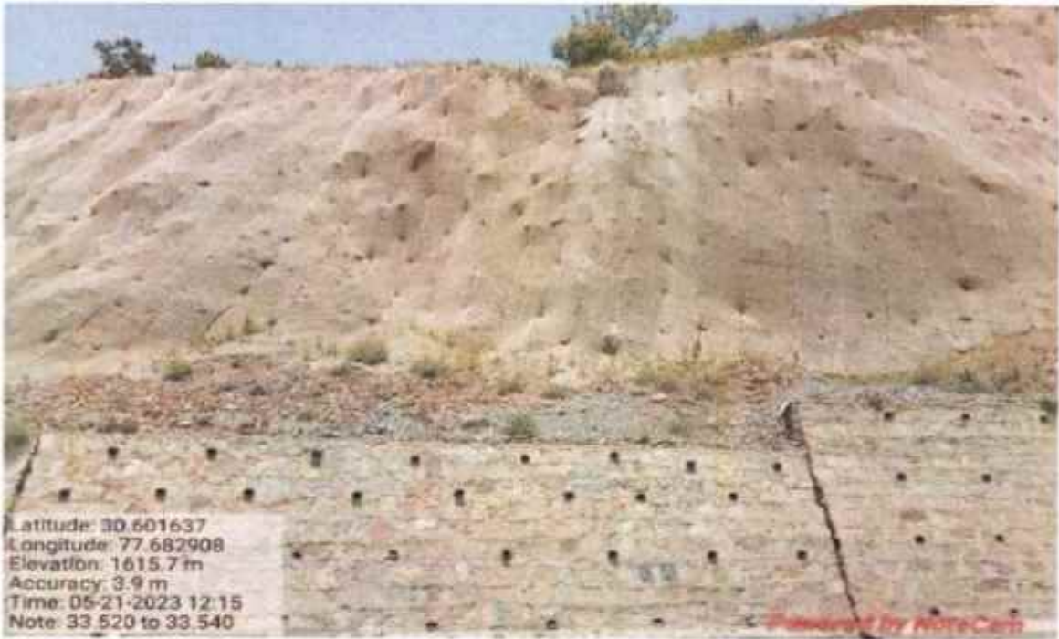
Coco fibre work at km 33+520 to 33+540
