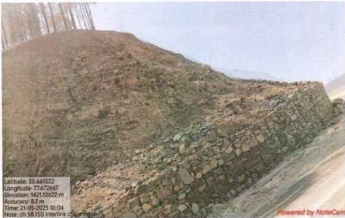
Interlink chain mesh work at km 58+150
