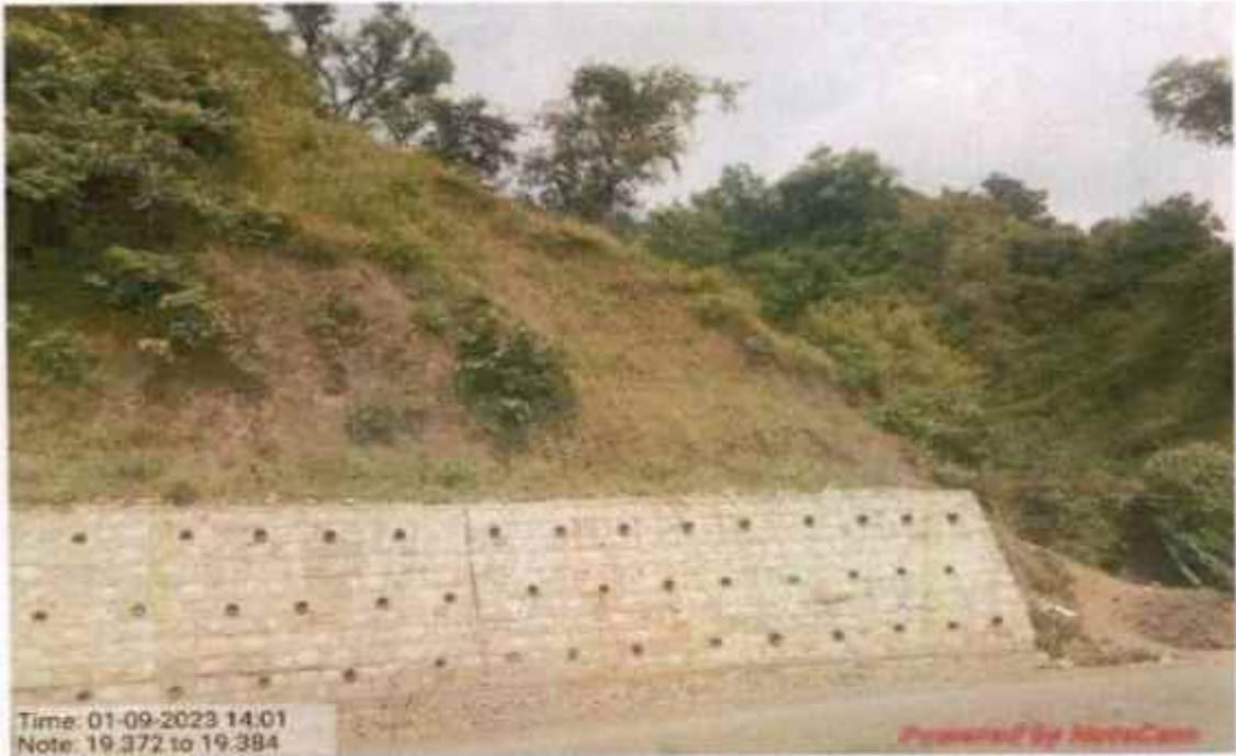
Interlink chain mesh work at km 13+372 to 19+384
