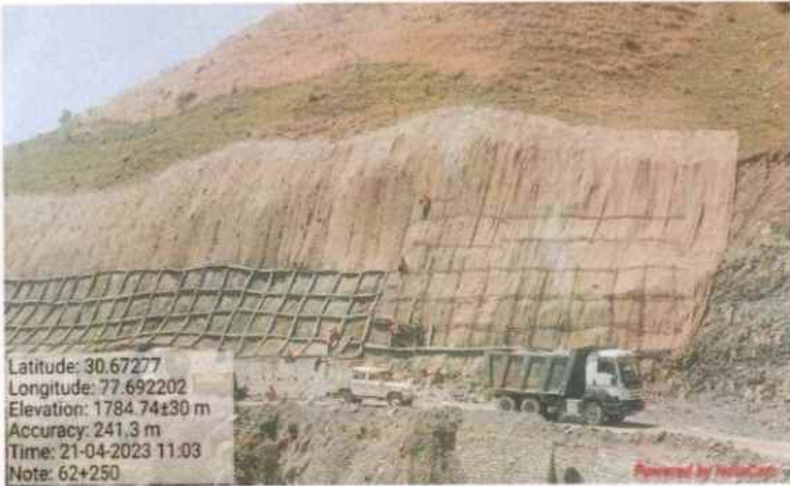
Shotcrete Crib wall work at km 62+250
