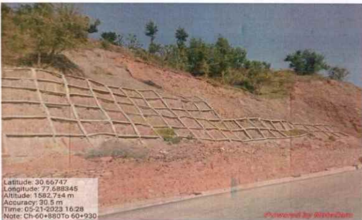
Shotcrete Crib wall work at km 60+880 to 60+930
