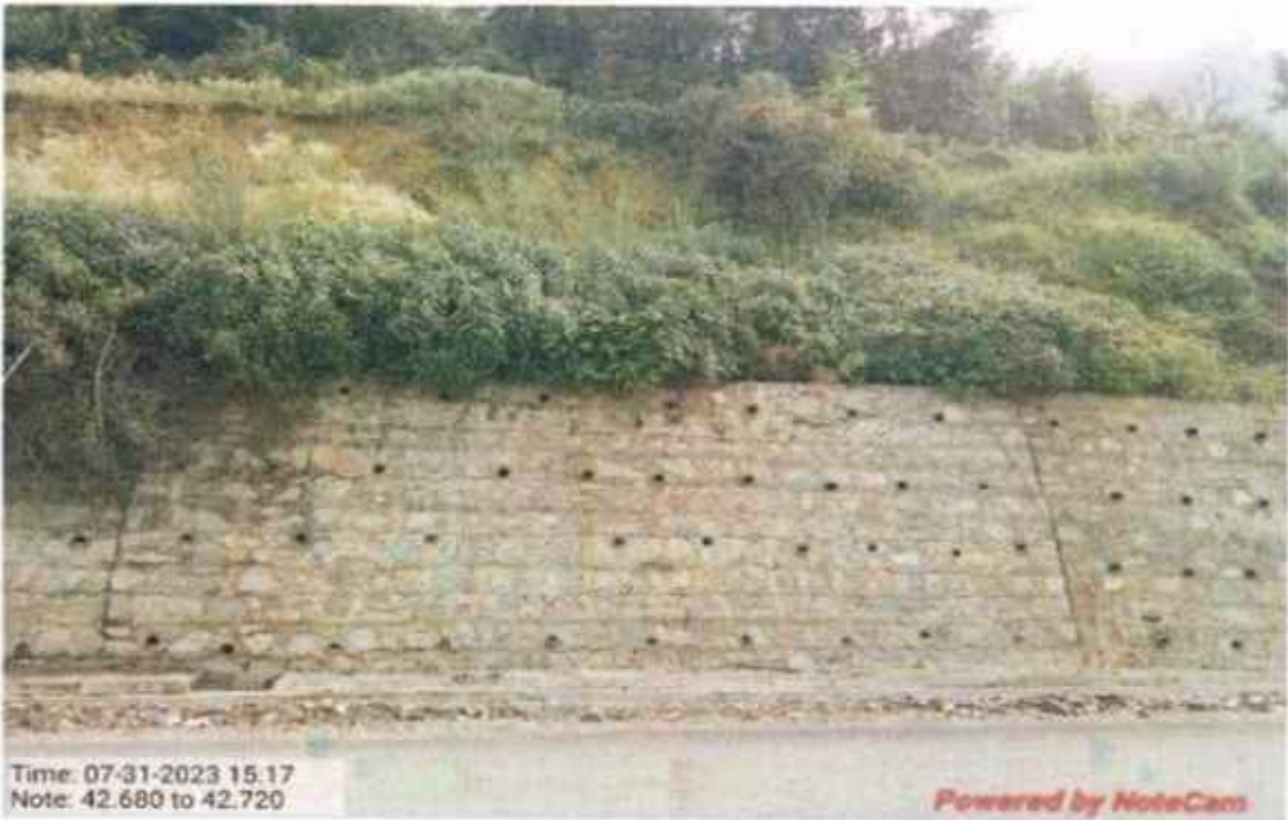
Hydro seeding work at km 42+680 to 42+720
