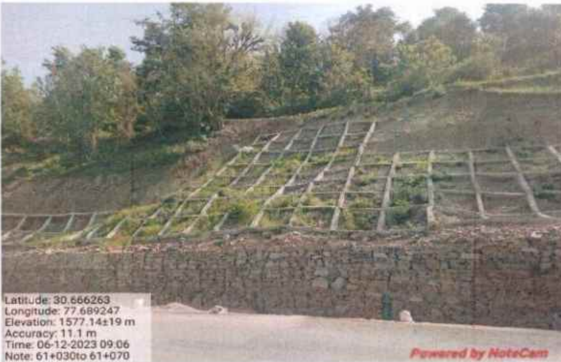
Shotcrete Crib wall work at km 61+030 to 61+070
