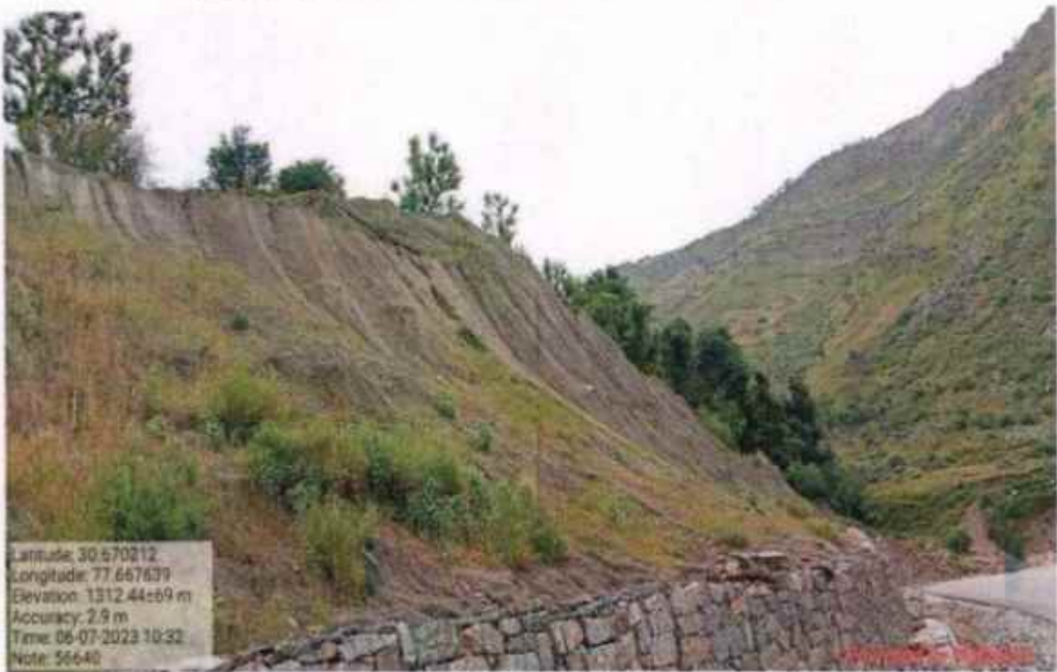
Coco fibre with Grass work at km 56+640
