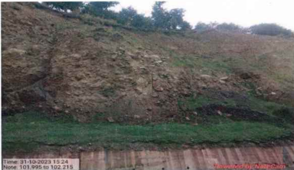
Geo cell with Hydro seeding and Bamboo plantation work at km 101+995 to 102+215
