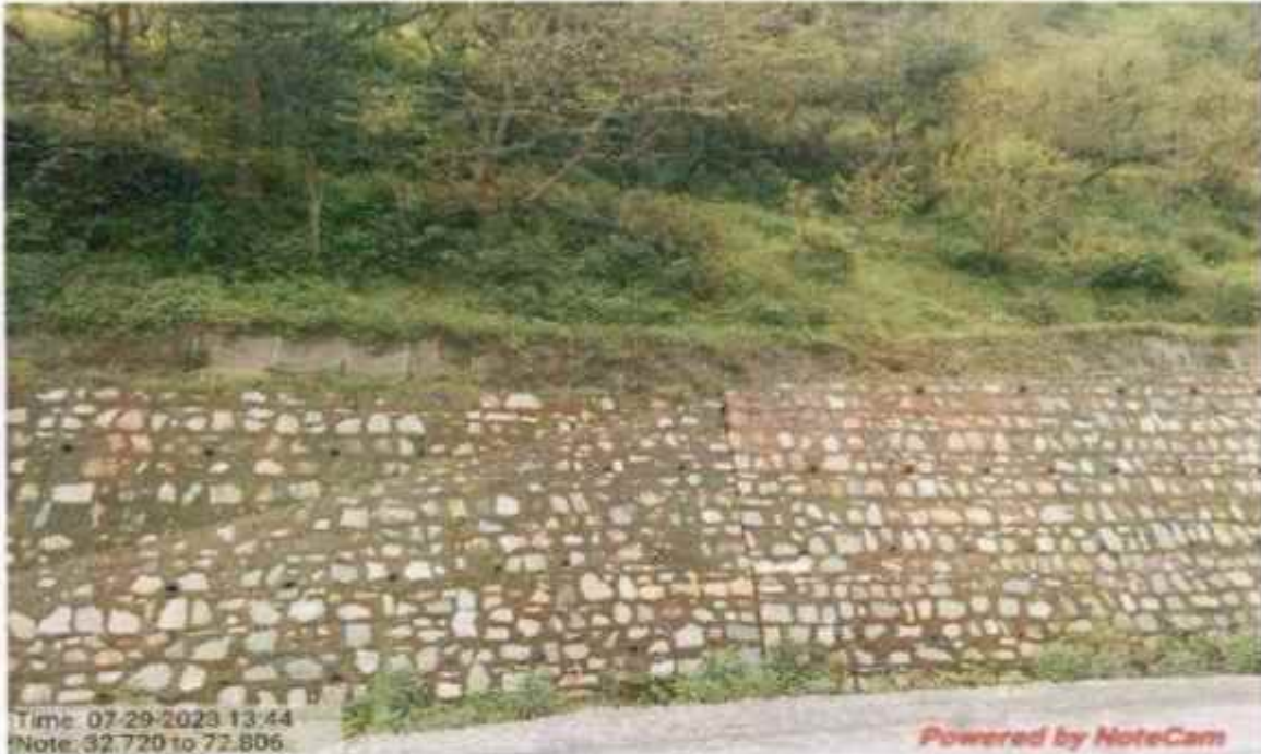
Coco fibre work at km 32+720 to 32+806
