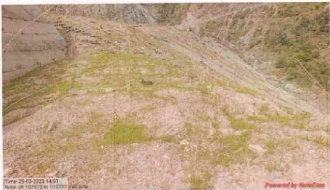
Valley side Bamboo plantation and hydro seeding work at km 102+572 to 102+720
