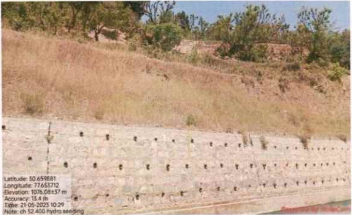
Hydro seeding work at km 52+400
