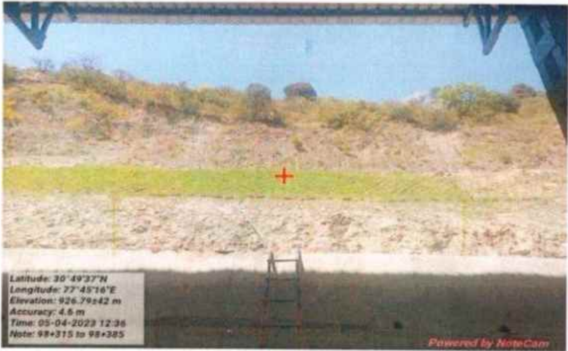
Geo cell with hydro seeding and Bamboo plantation work at km 98+315 to 98+385
