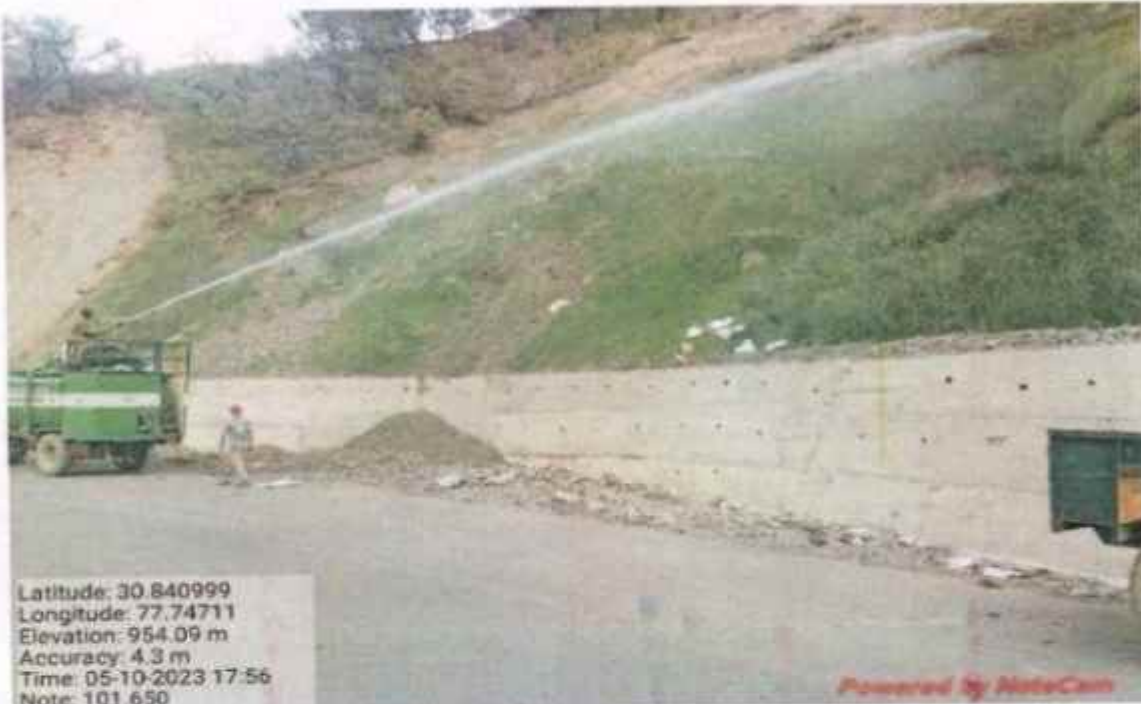
Hydro seeding work at km 101+650
