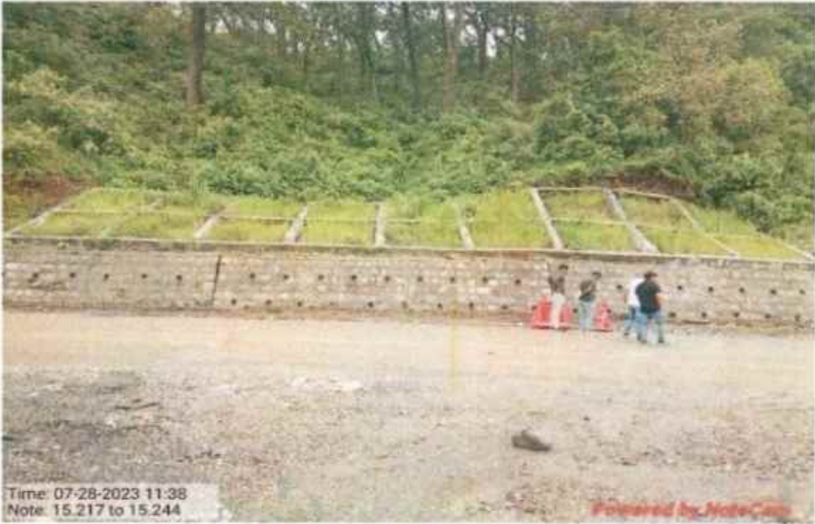
Shotcrete crib wall work at km 15+217 to 15+244
