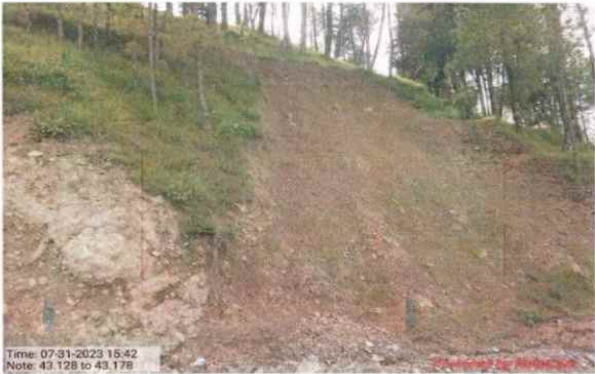
Interlink chain mesh work at km 42+128 to 43+178
