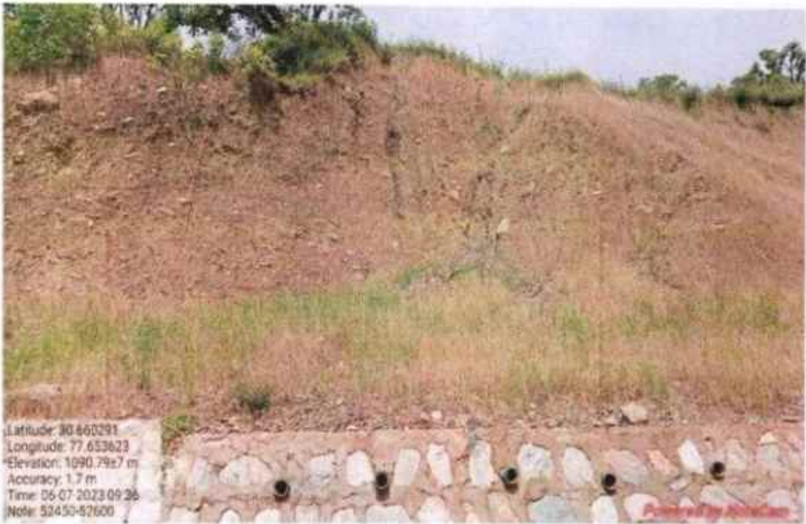
Hydro seeding work at km 52+450 to 52+600
