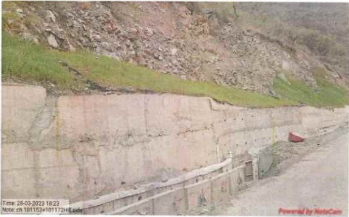
Geo cell with Hydro seeding work at km 101+153 to 101+172
