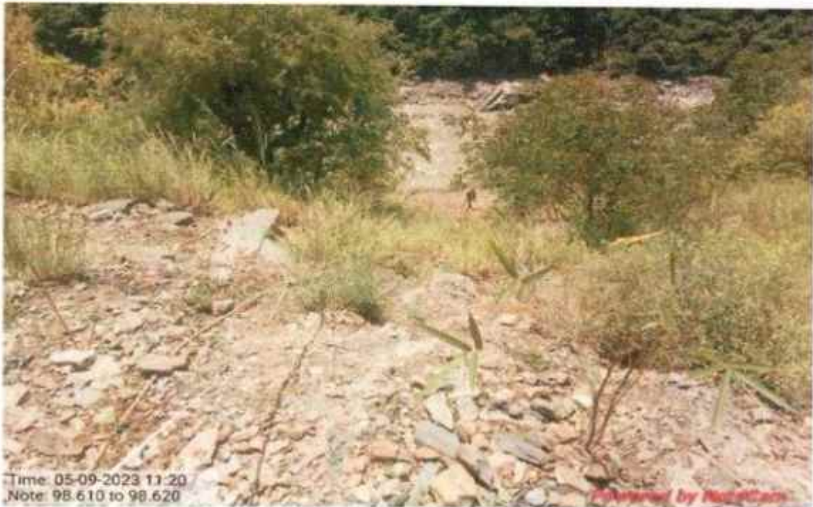
Valley side Bamboo plantation work at km 98+610 to 98+620
