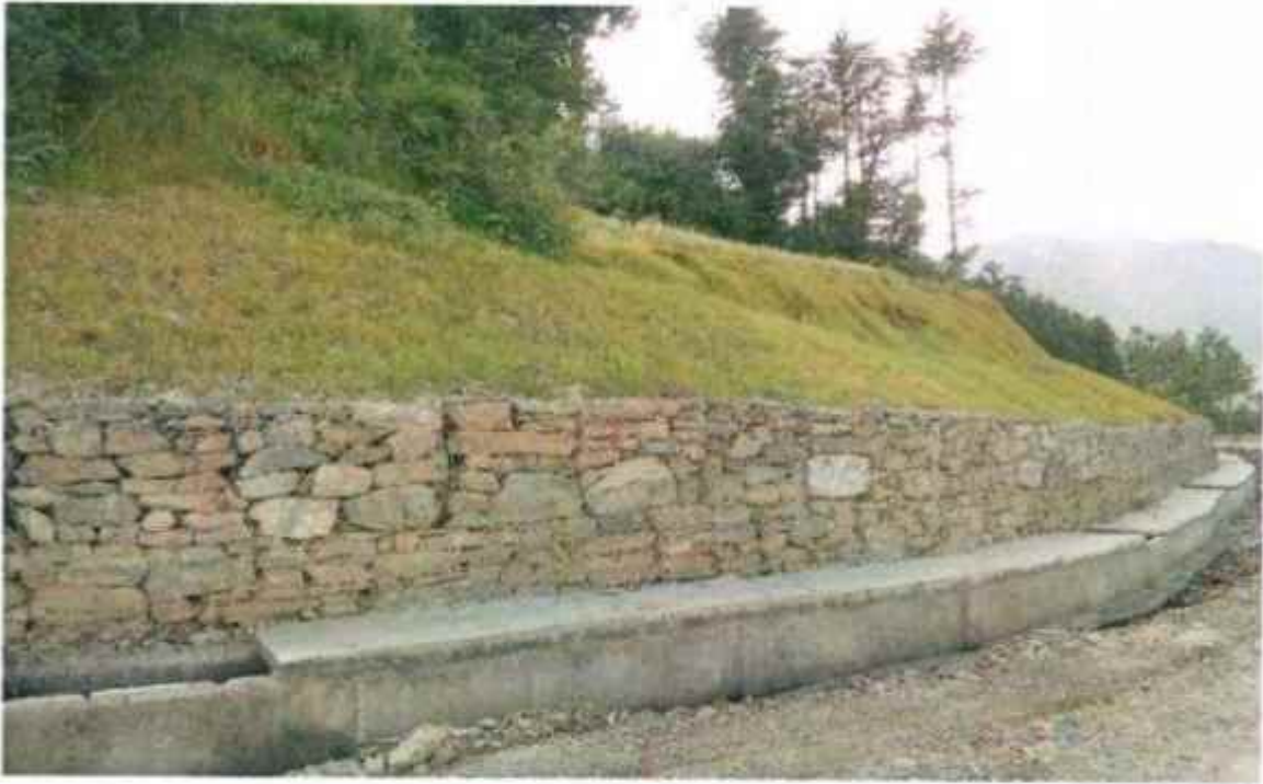
Hydro seeding work at km 70+220
