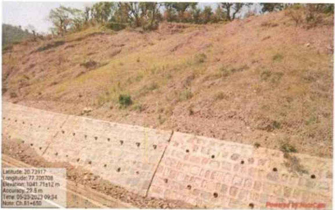
Interlink chain mesh work at km 81+650
