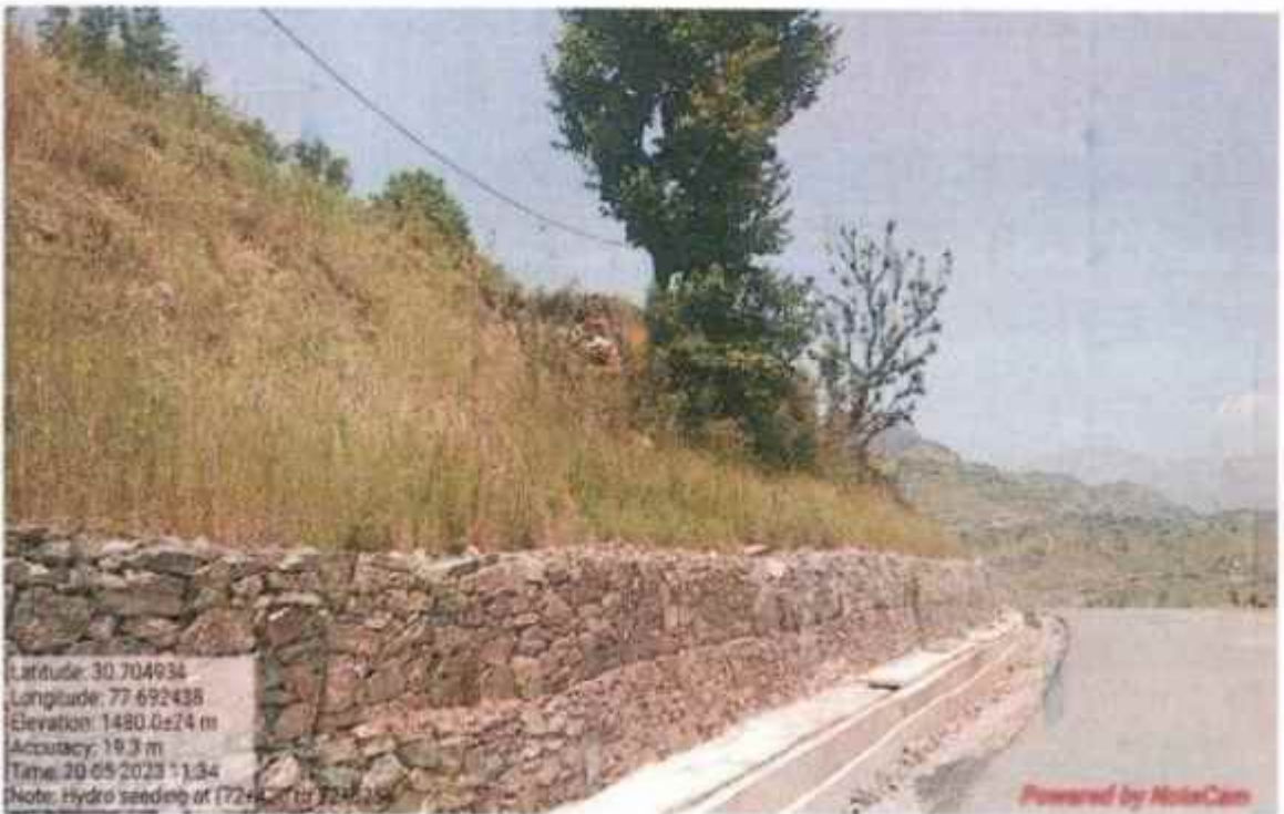
Hydro seeding work at km 72+420 to 72+525
