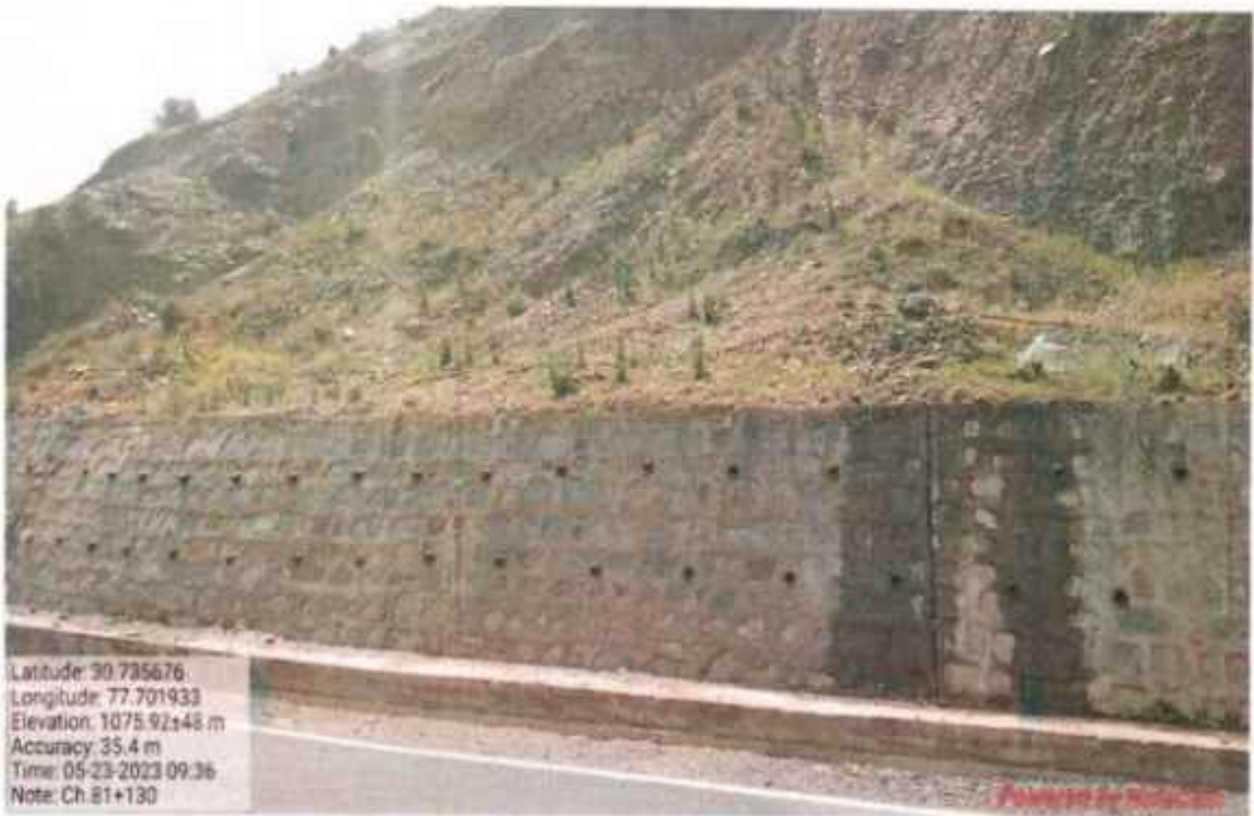
Interlink chain mesh work at km 81+130
