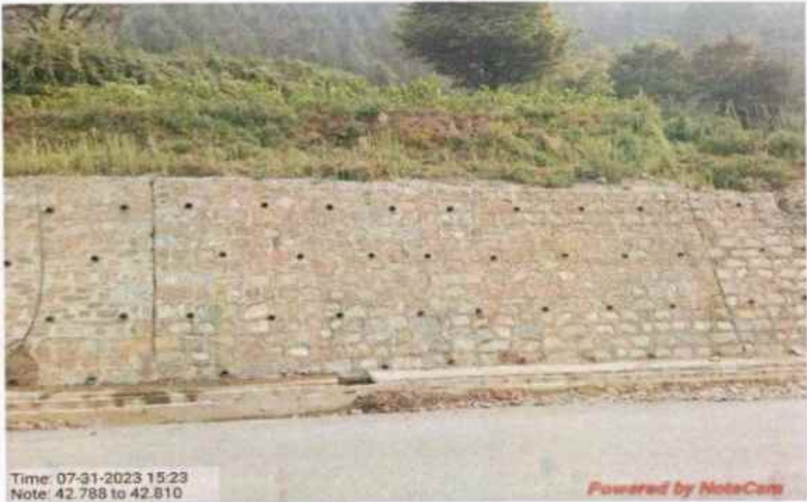
Hydro seeding work at km 42+788 to 42+810
