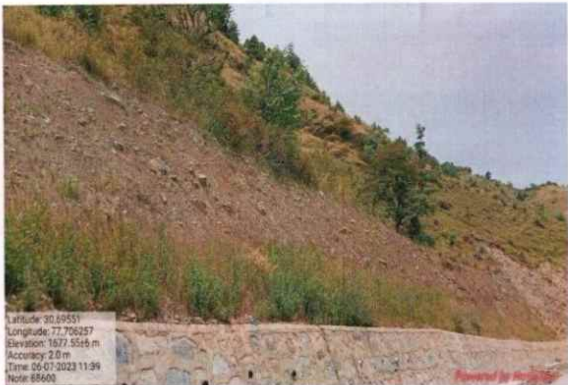
Hydro seeding work at km 68+600
