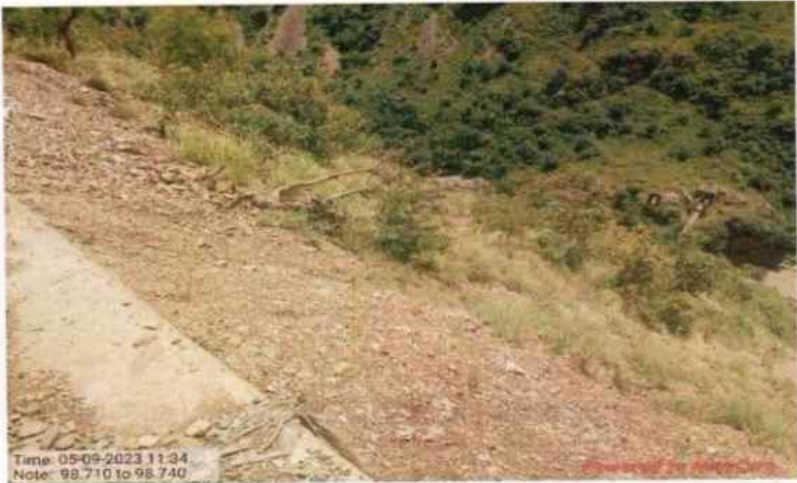
Valley side Bamboo plantation work at km 98+710 to 98+740
