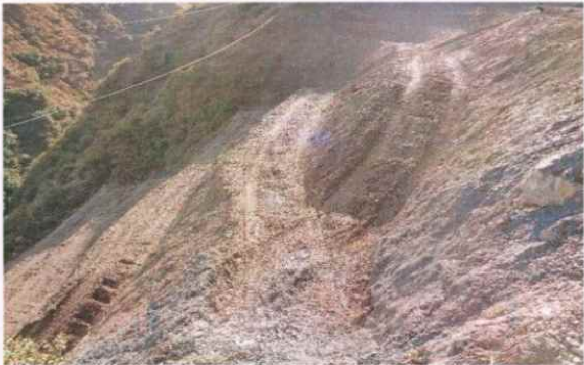
Valley side Bio-Engineering work at km 83+250
