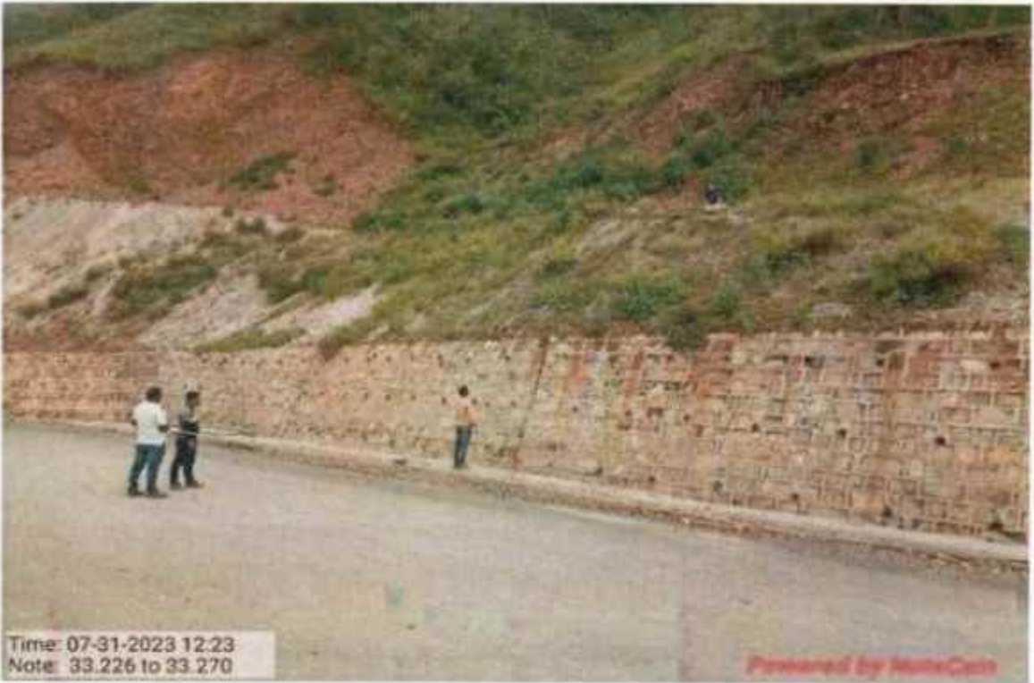
Coco fibre work at km 33+226 to 33+270
