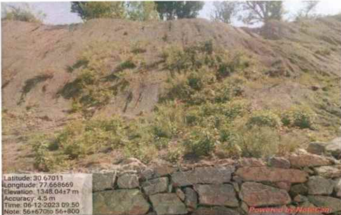
Coco fibre with Grass work at km 56+670 to 56+800
