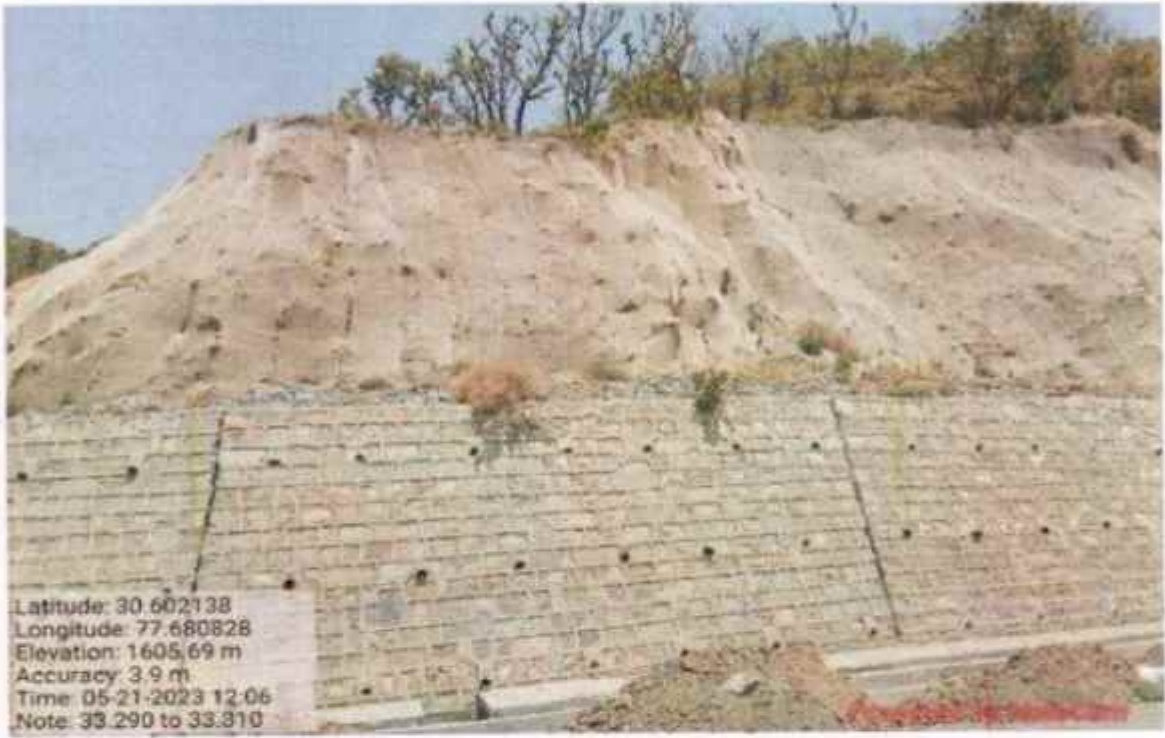
Coco fibre work at km 33+290 to 33+310
