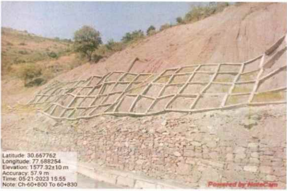
Shotcrete Crib wall work at km 60+800 to 60+830
