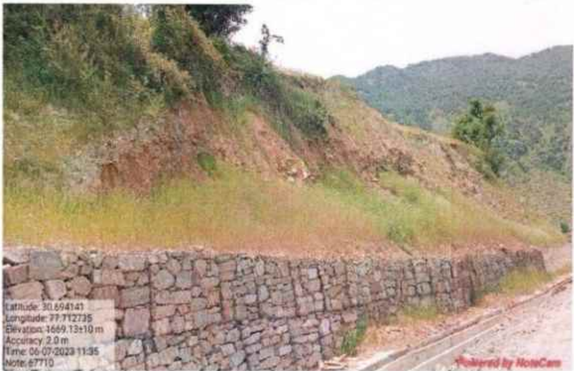
Hydro seeding work at km 67+710
