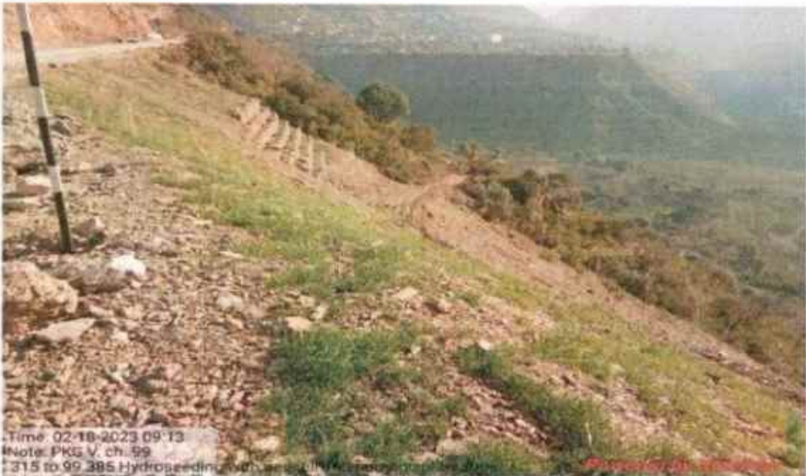
Valley side Geo cell with Hydro seeding and Bamboo plantation work at km 99+315 to 99+385
