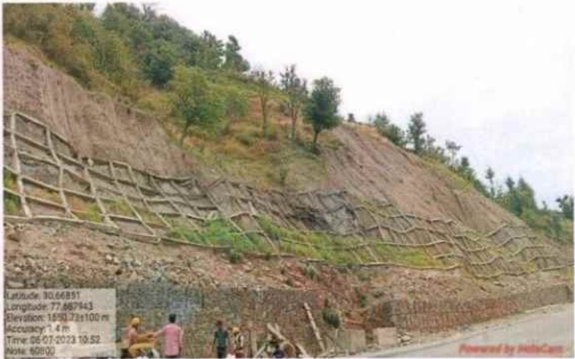
Shotcrete Crib wall work at km 60+800
