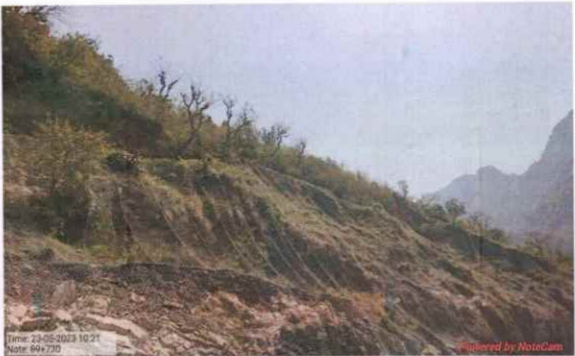
Interlink chain mesh work at km 89+730
