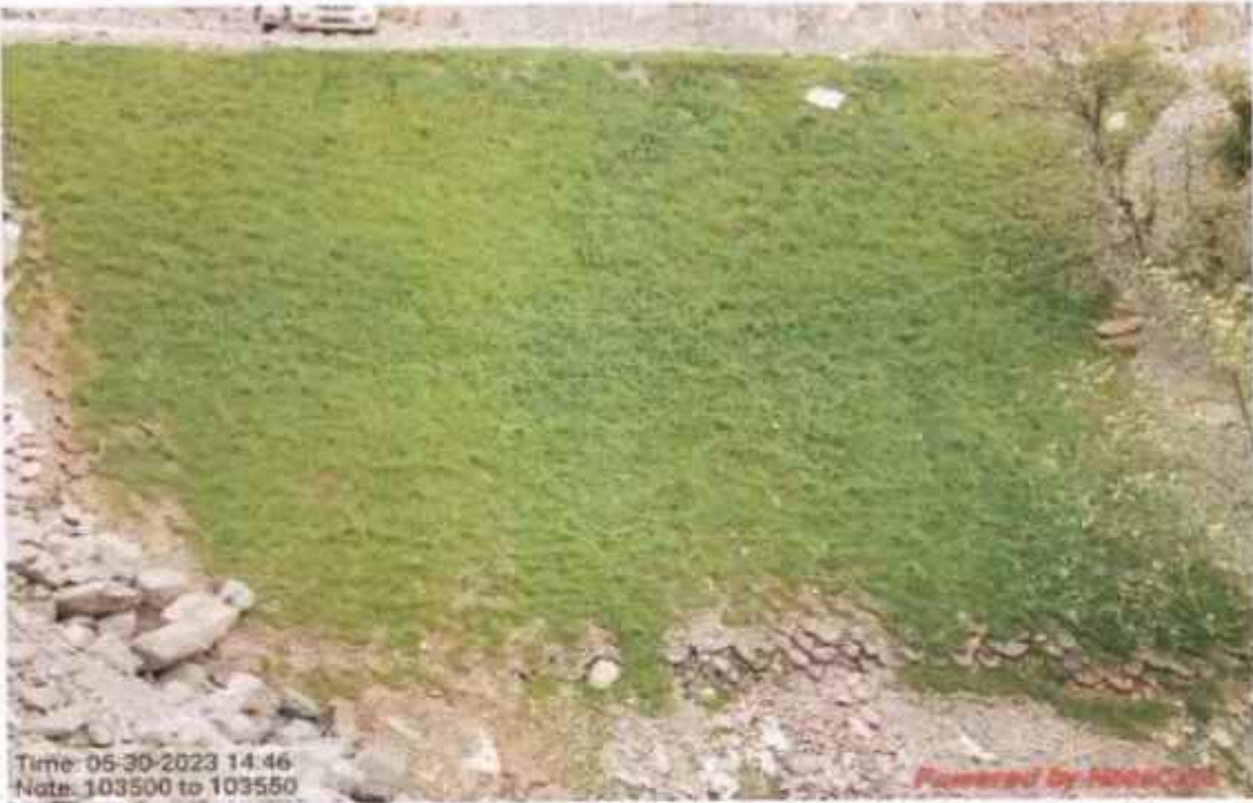
Valley side Geo cell with Hydro seeding and Bamboo plantation at km 103+500 to 103+550
