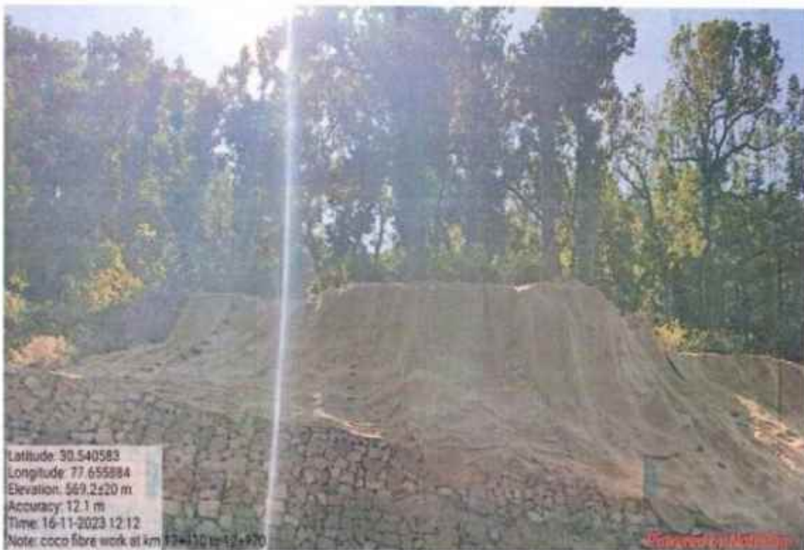
Coco fibre work at km 12+910 to 12+970
