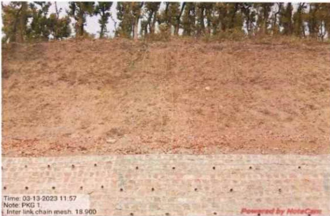
Interlink chain mesh work at km 18+900
