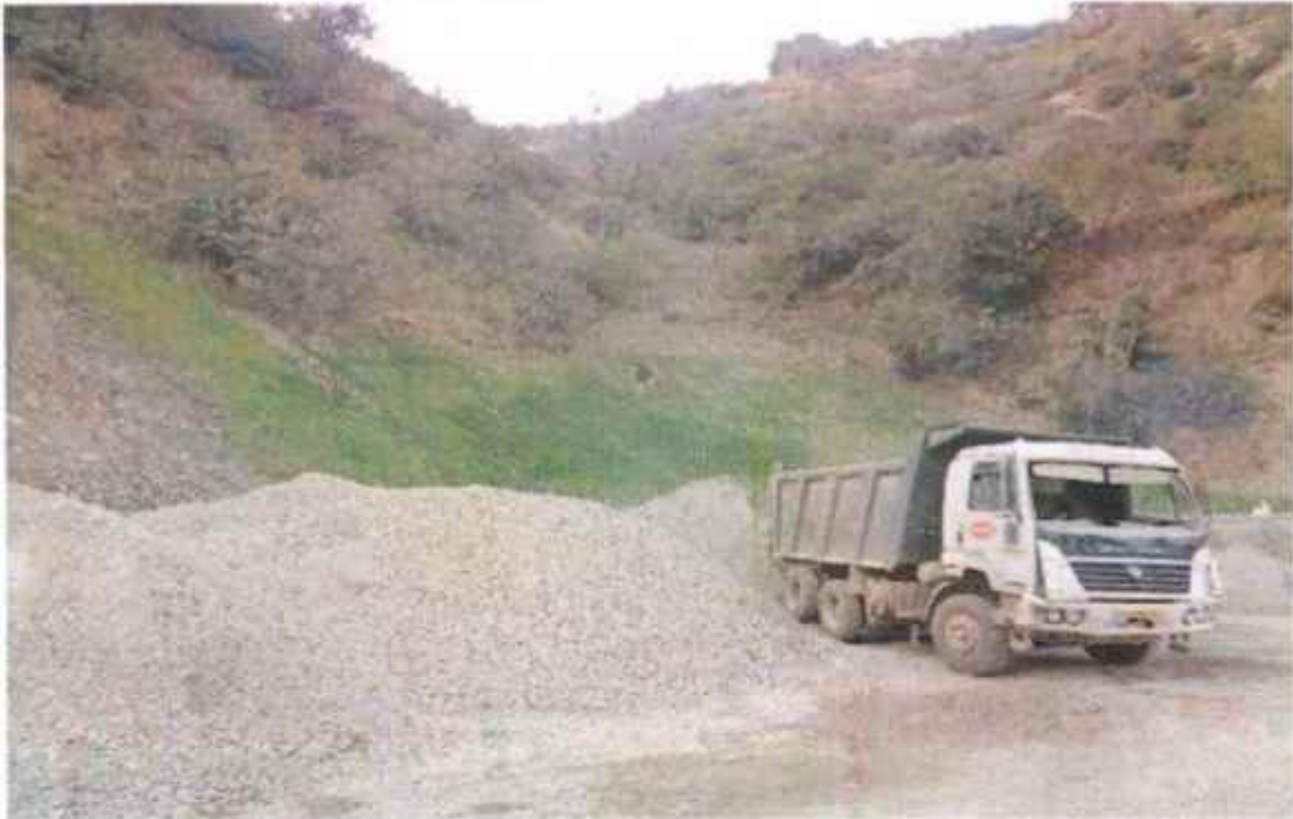
Geo cell with Hydro seeding and Bamboo plantation work
