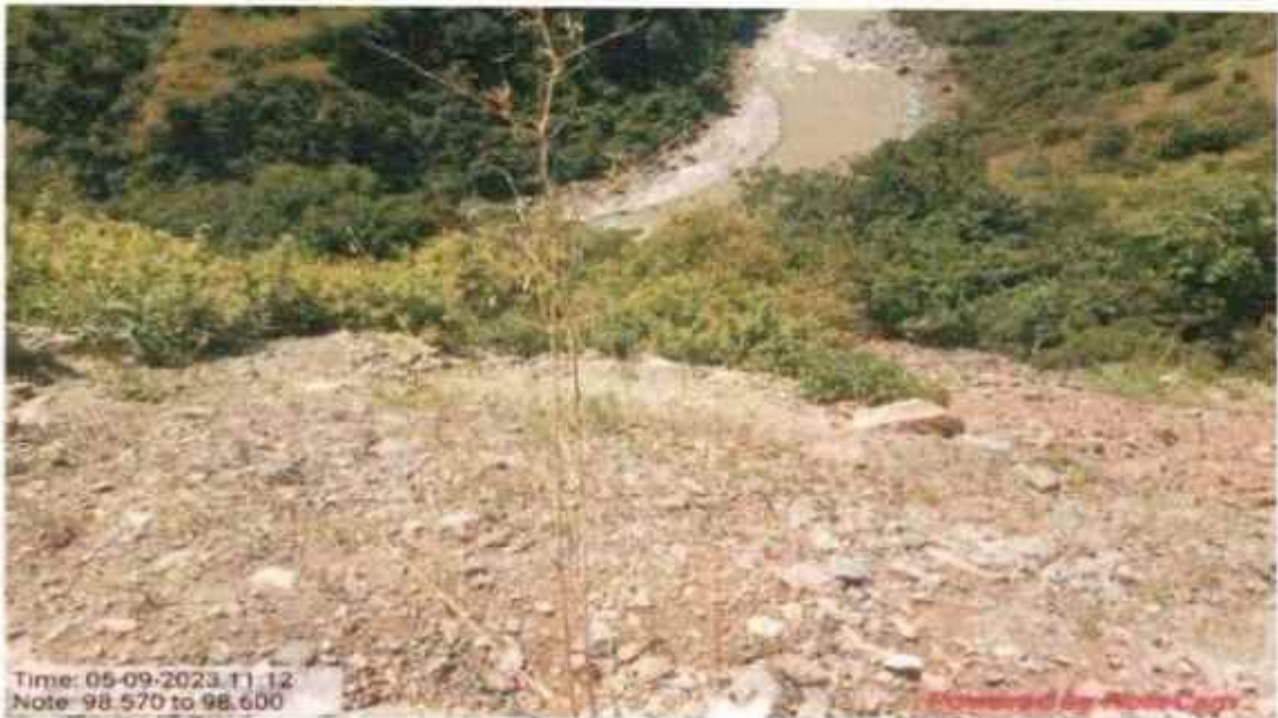
Valley side Bamboo plantation work at km 98+570 to 98+600
