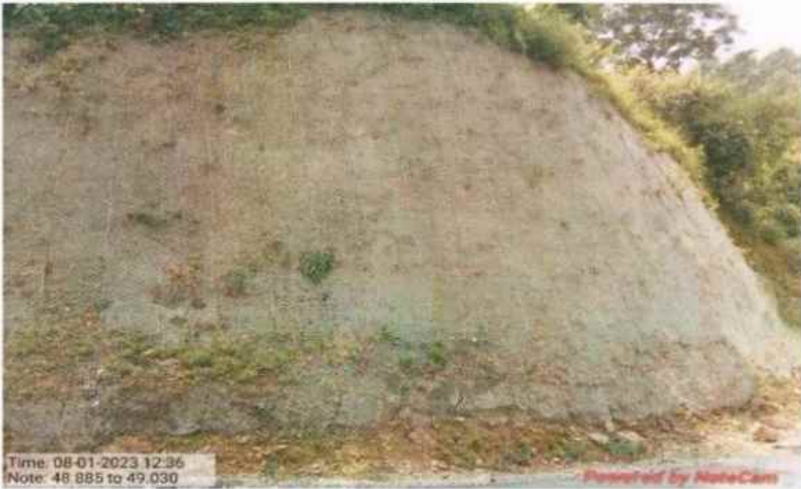
Interlink chain mesh work at km 48+885 to 49+030
