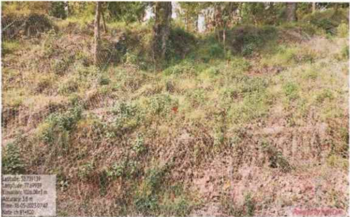
Interlink chain mesh work at km 81+800
