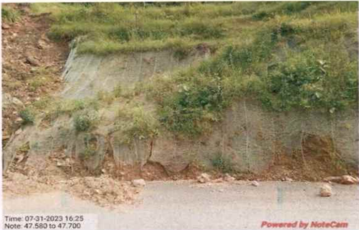
Coco fibre work at km 47+580 to 47+700
