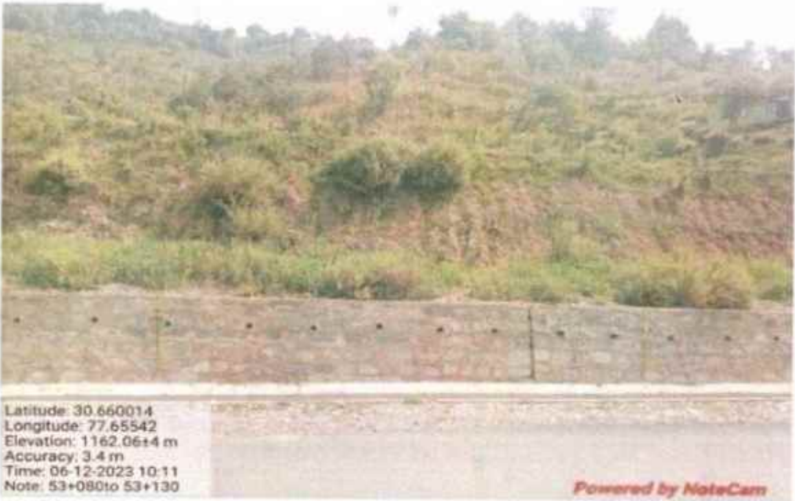
Hydro seeding work at km 53+080 to 53+130
