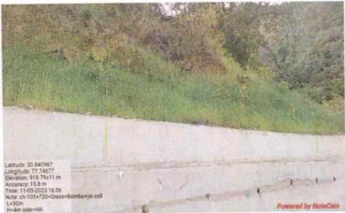
Geo cell with Hydro seeding and Bamboo plantation work at km 101+720
