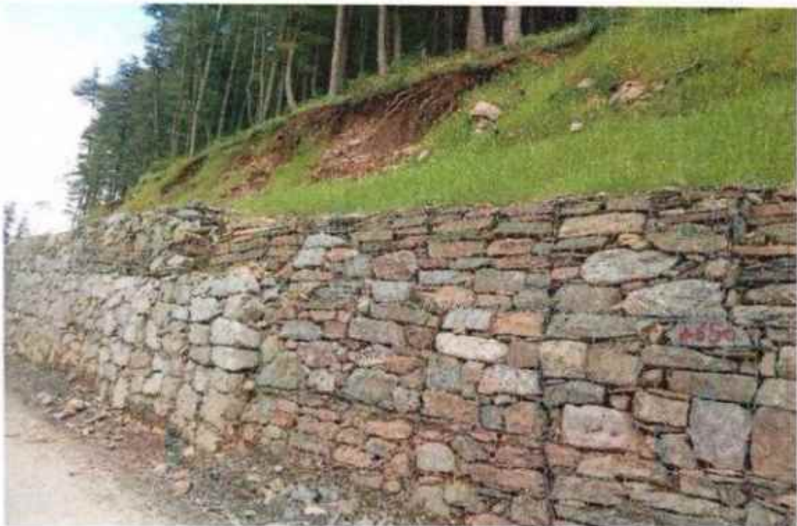
Hydro seeding work at km 70+650
