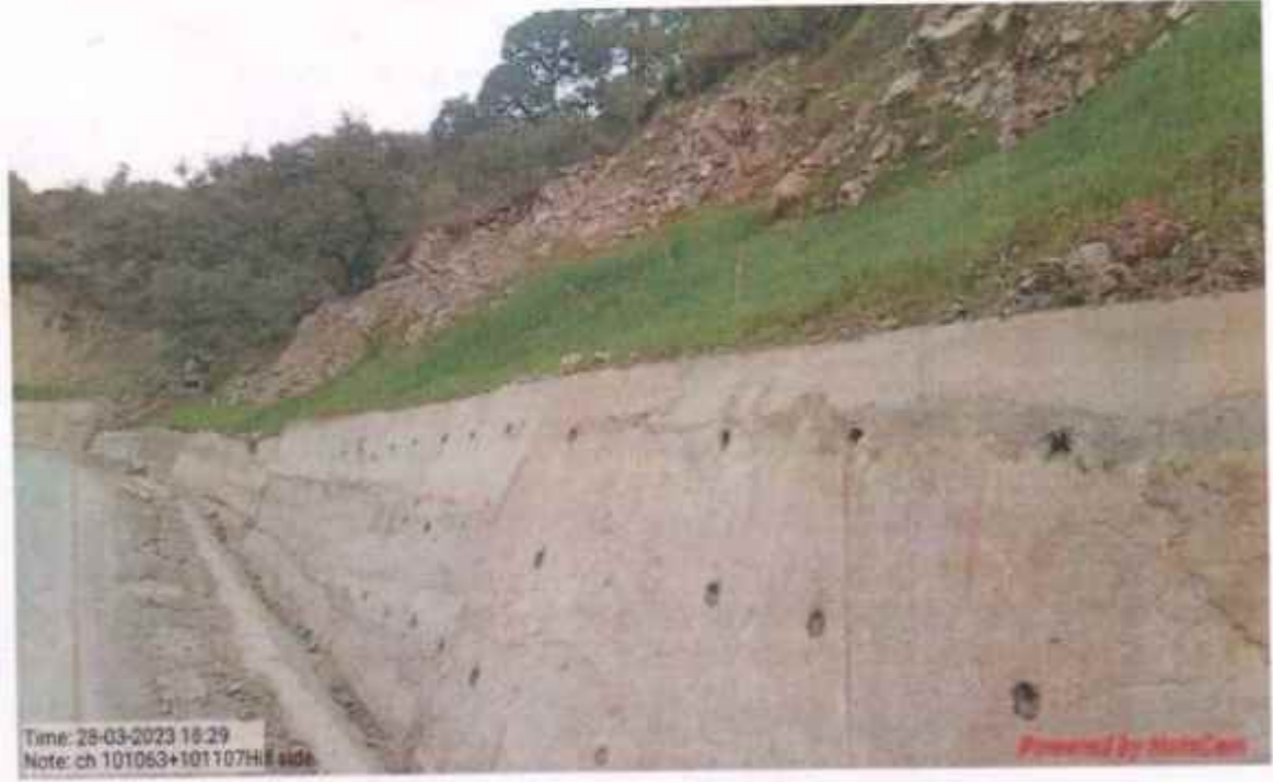
Geo cell with Hydro seeding and Bamboo plantation work at km 101+063 to 101+107
