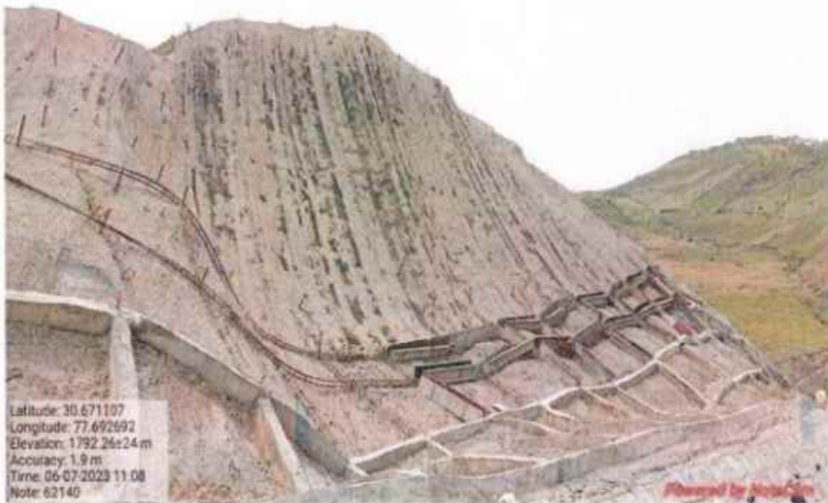
Shotcrete Crib wall work at km 62+140
