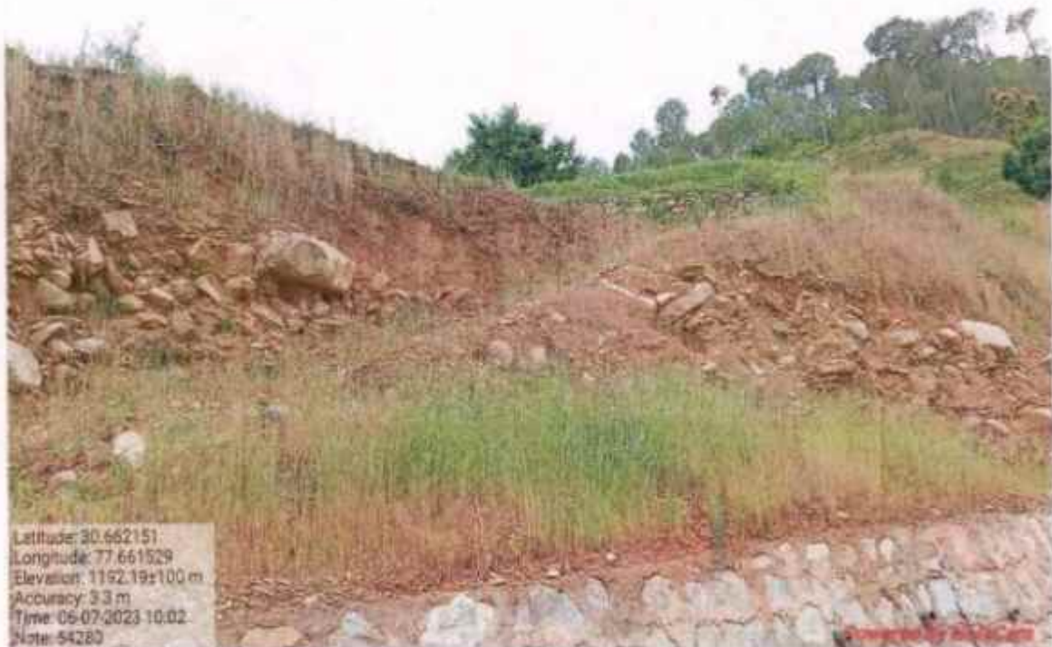
Hydro seeding work at km 54+280
