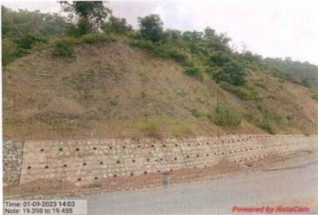
Interlink chain mesh work at Km 19+398 to 19+455
