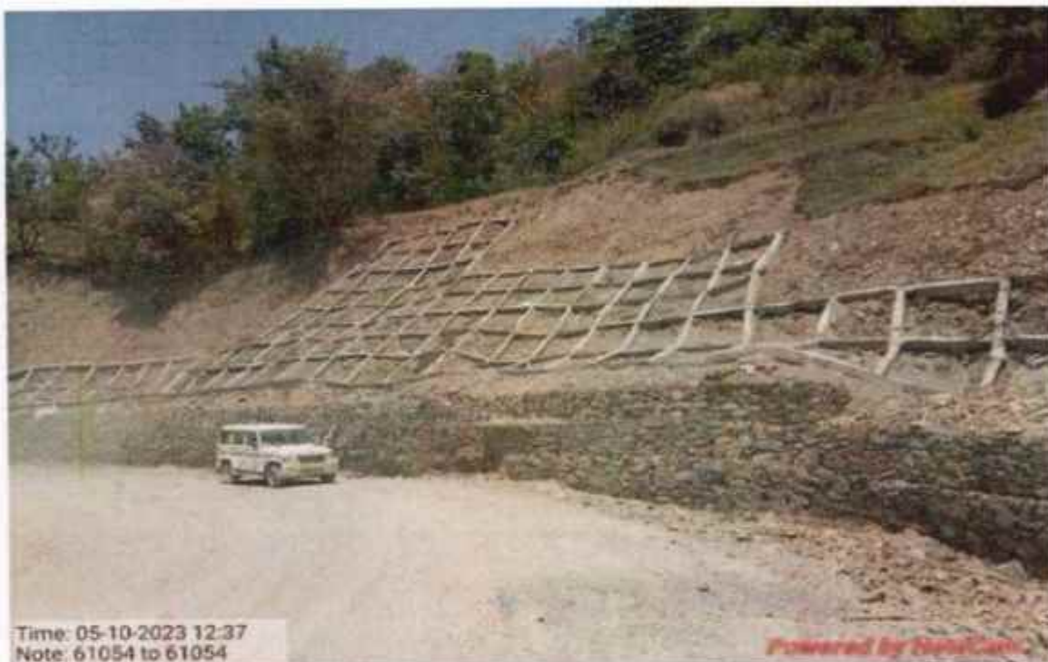
Shotcrete Crib wall work at km 61+054
