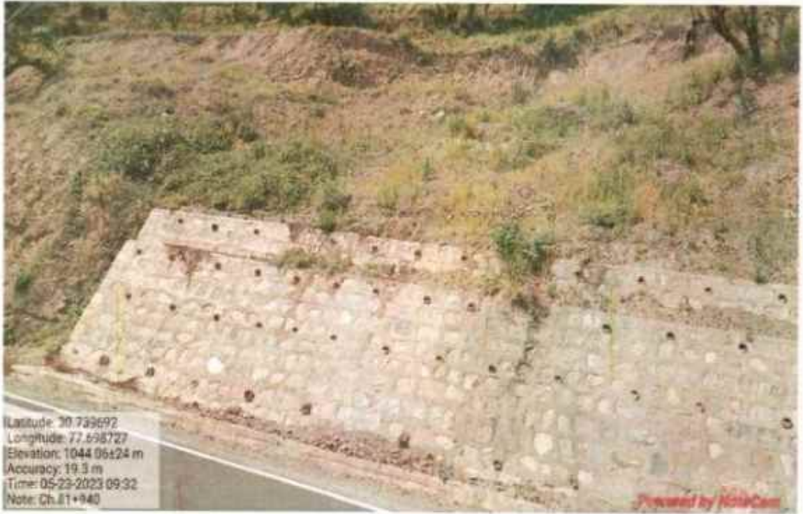
Interlink chain mesh work at km 81+940
