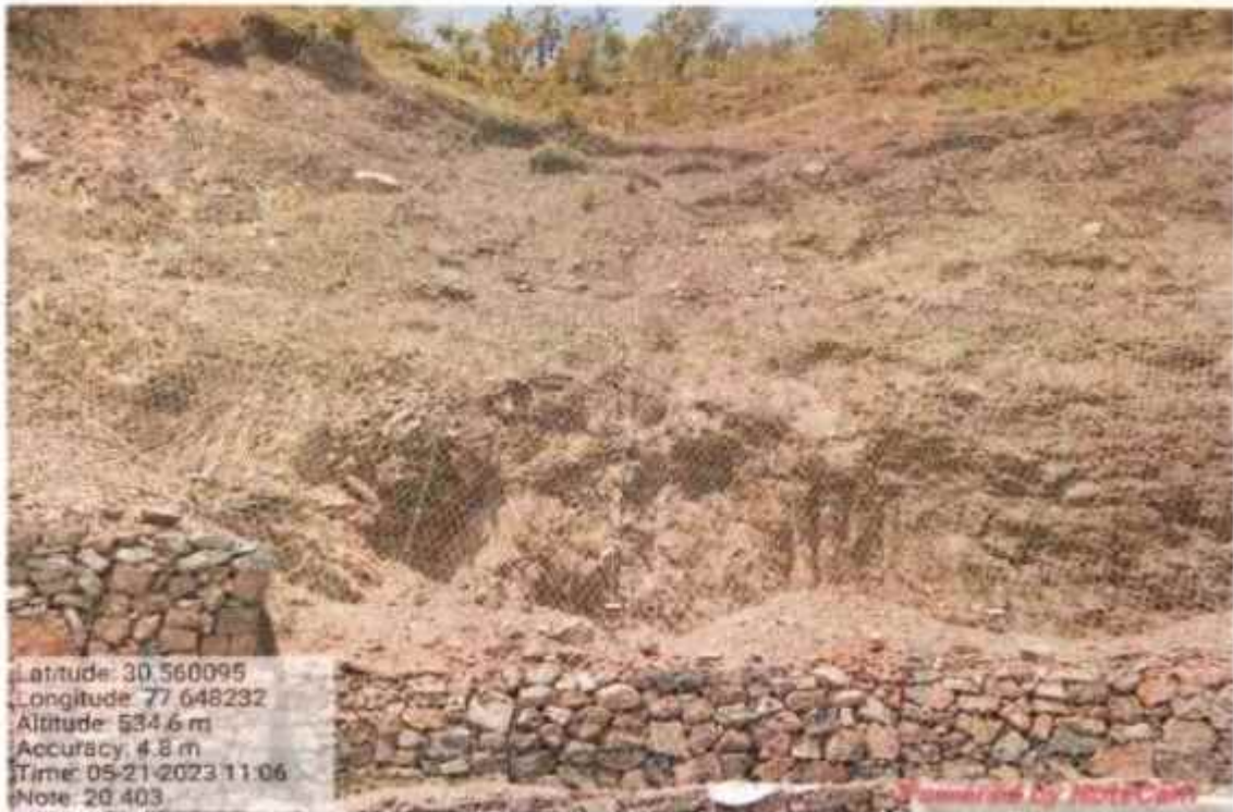
Interlink chain mesh work at Km 20+403
