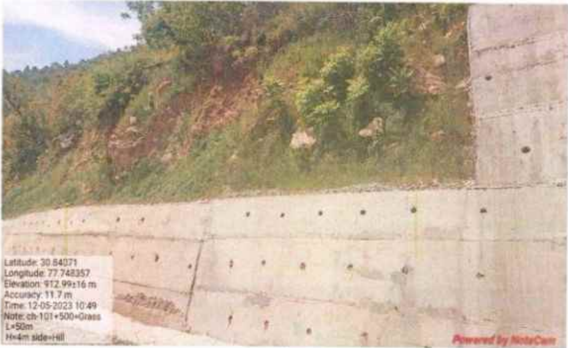
Hydro seeding work at km 101+500
