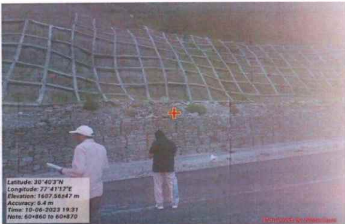
Shotcrete Crib wall work at km 60+860 to 60+870
