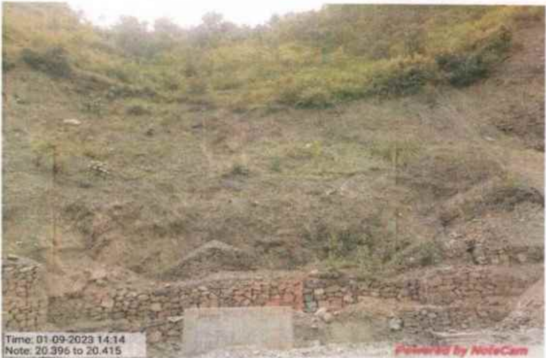
Interlink chain mesh work at Km 20+396 to 20+415
