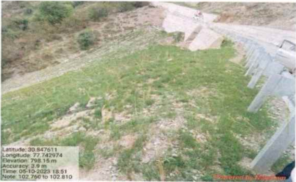
Valley side Geo cell with Hydro seeding and Bamboo plantation work at km 102+760 to 102+810
