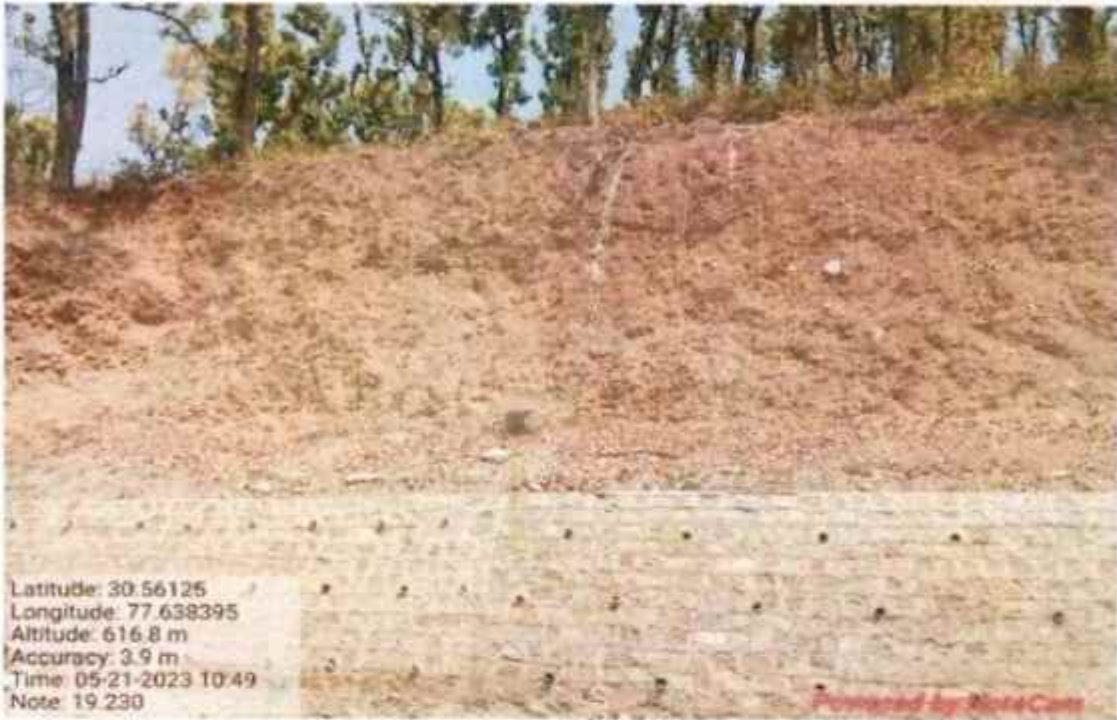
Interlink chain mesh work at km 19+230
