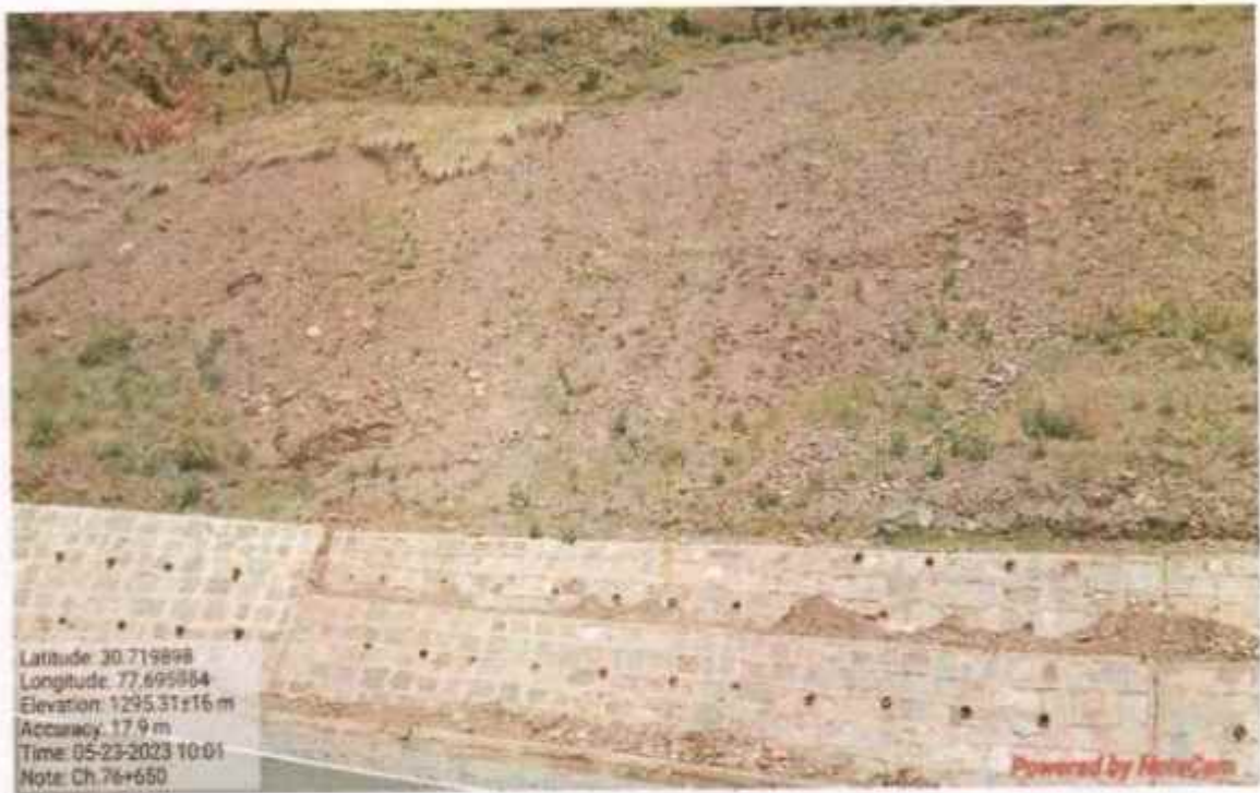
Interlink chain mesh work at km 76+650
