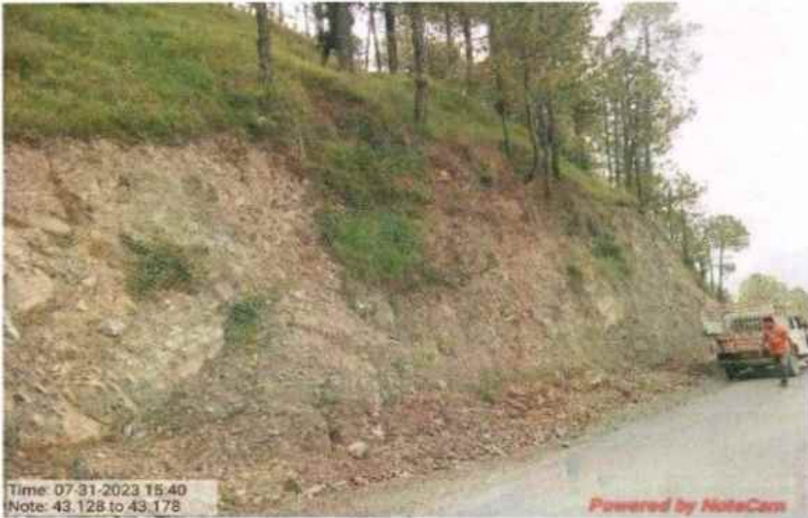
Interlink chain mesh work at km 43+128 to 43+178
