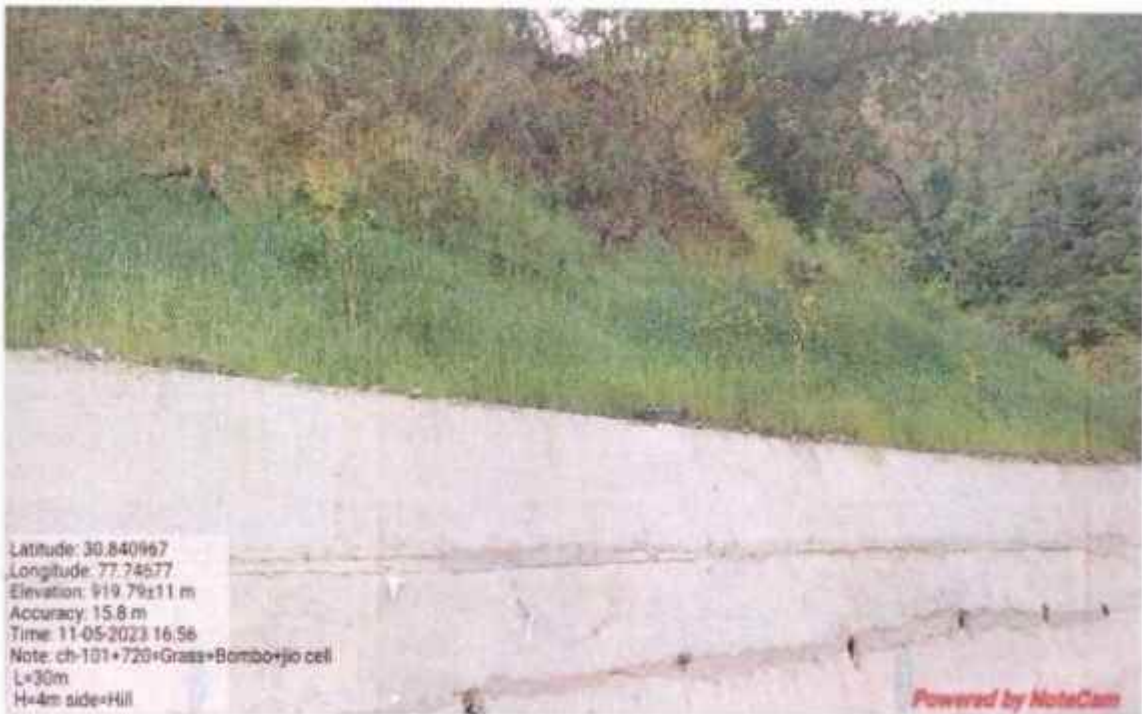
Hydro seeding and Geo cell with Hydro seeding work at km 101+720
