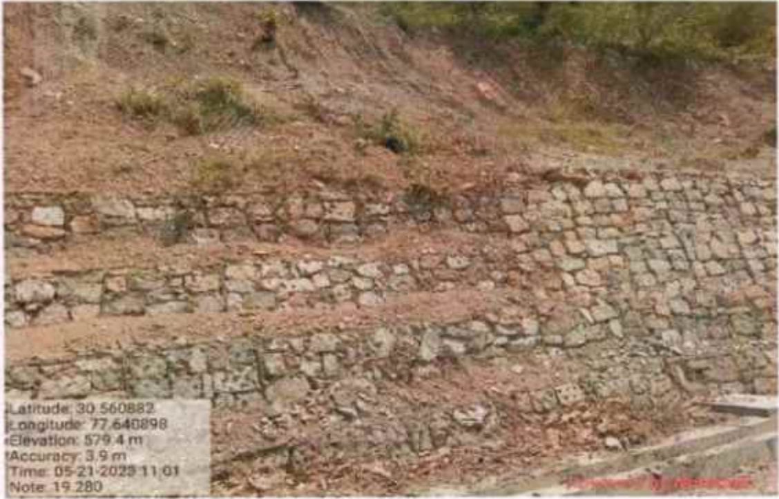
Interlink chain mesh work at Km 19.280
