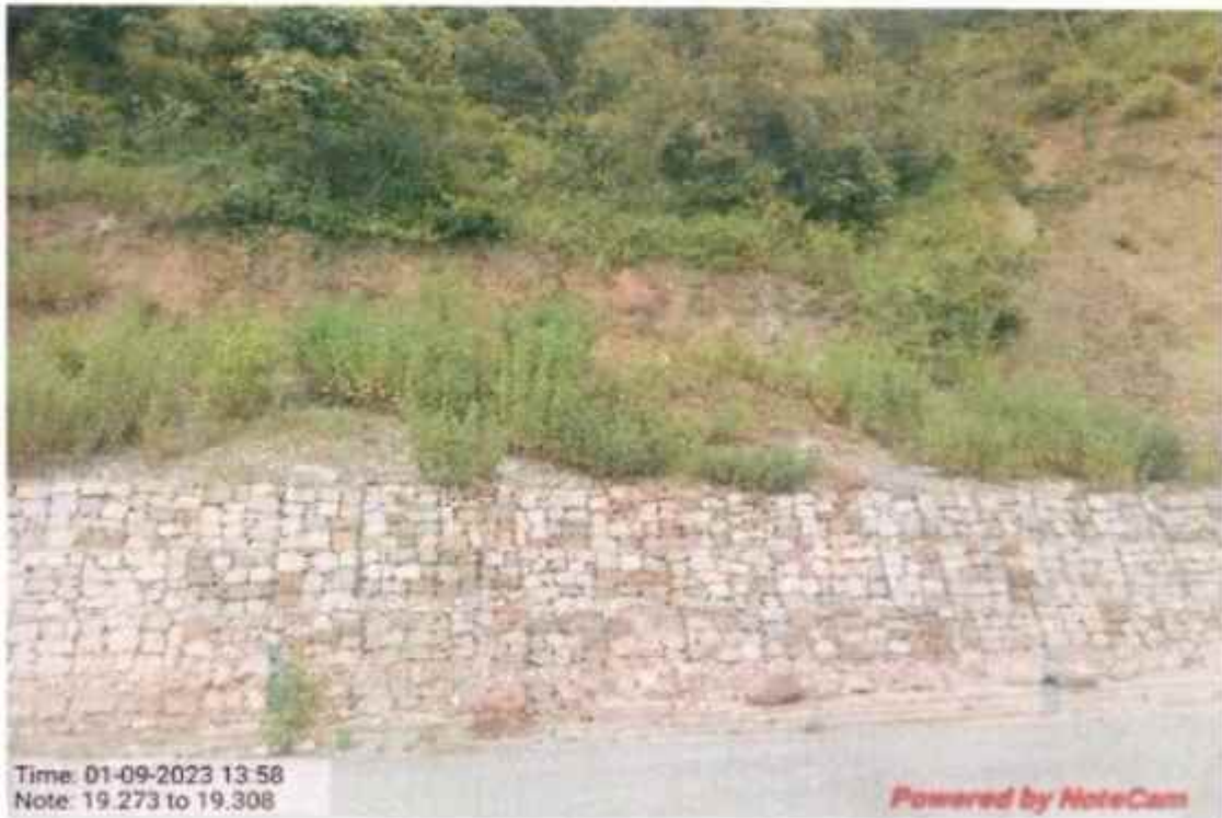
Interlink chain mesh work at km 19+273 to 19+308
