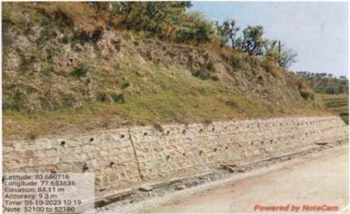
Hydro seeding work at km 52+100 to 52+180
