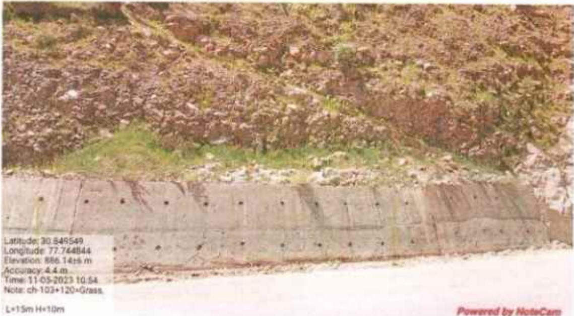
Hydro seeding work at km 103+120
