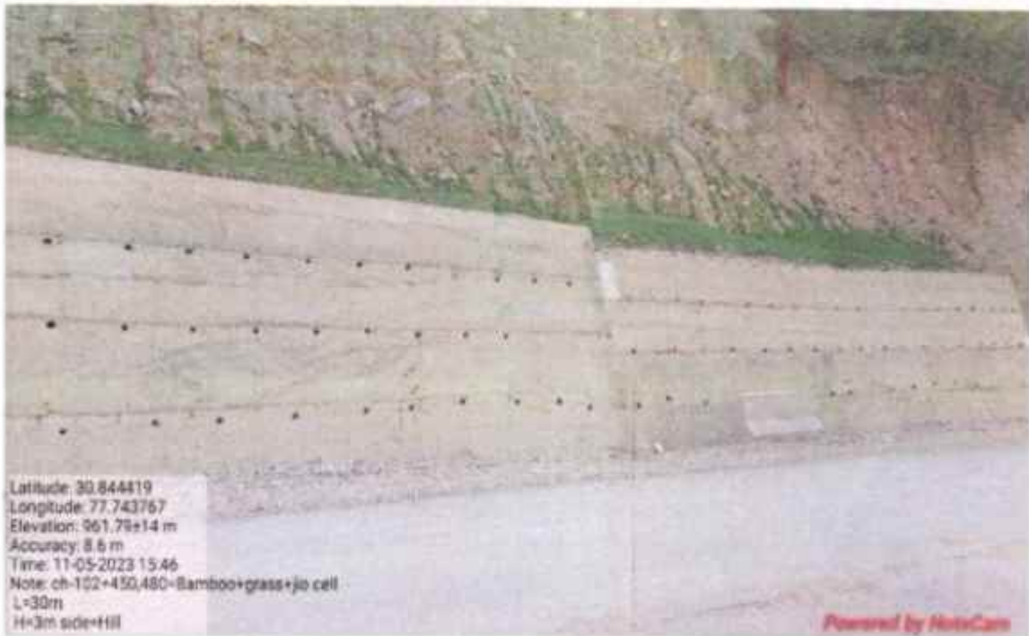
Geo cell with Hydro seeding work at km 102+450 to 102+480
