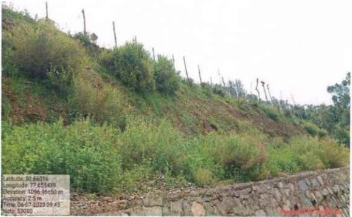
Hydro seeding work at km 53+080
