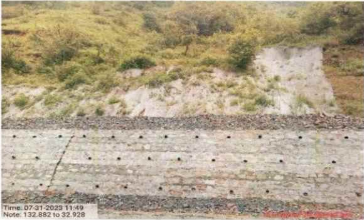
Coco fibre work at km 32+882 to 32+928
