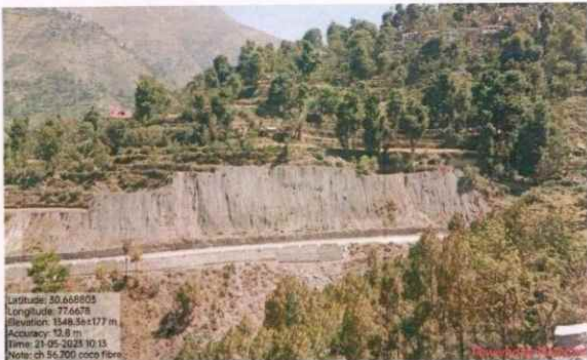
Coco fibre with Grass work at km 56+700
