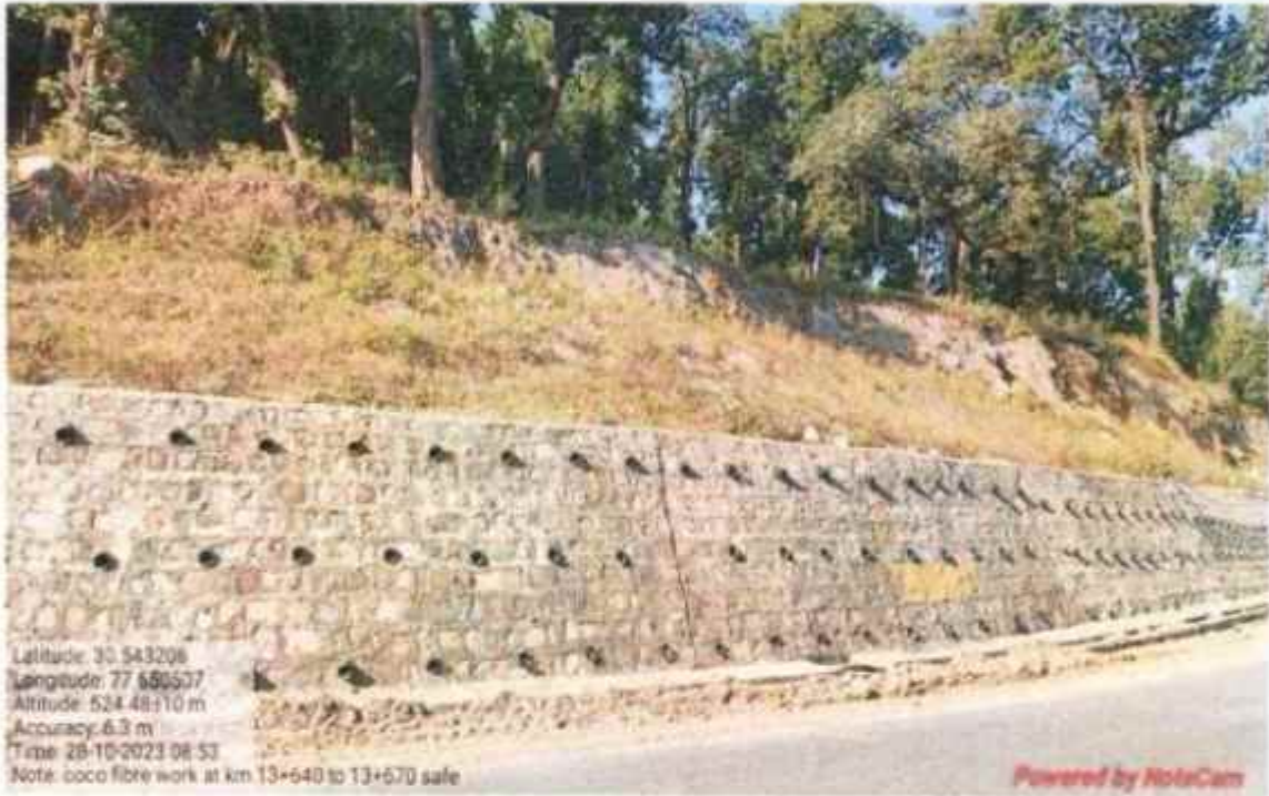
Coco fibre work at km 13+640 to 13+670
