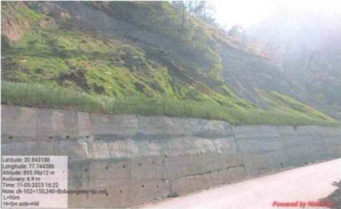
Hydro seeding and Geo cell with Hydro seeding work at km 102+150 to 102+240
