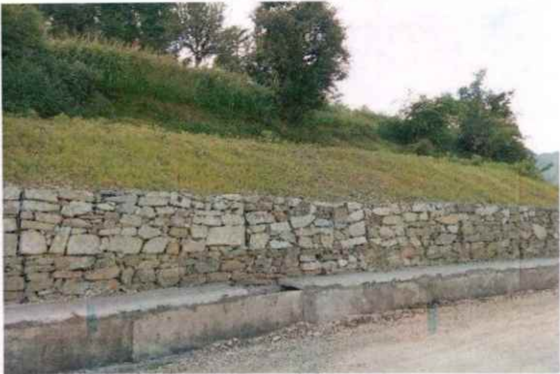
Hydro seeding work at km 70+170
