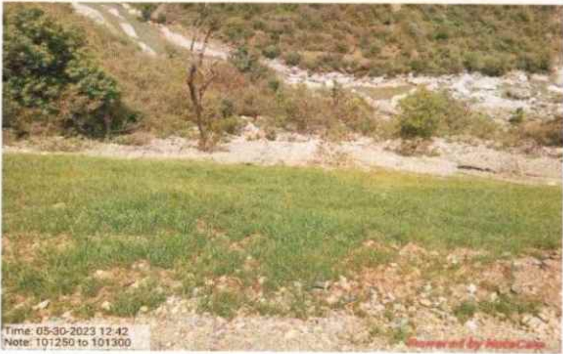
Valley side Geo cell with Hydro seeding and Bamboo plantation work at km 101.250 to 101.300
