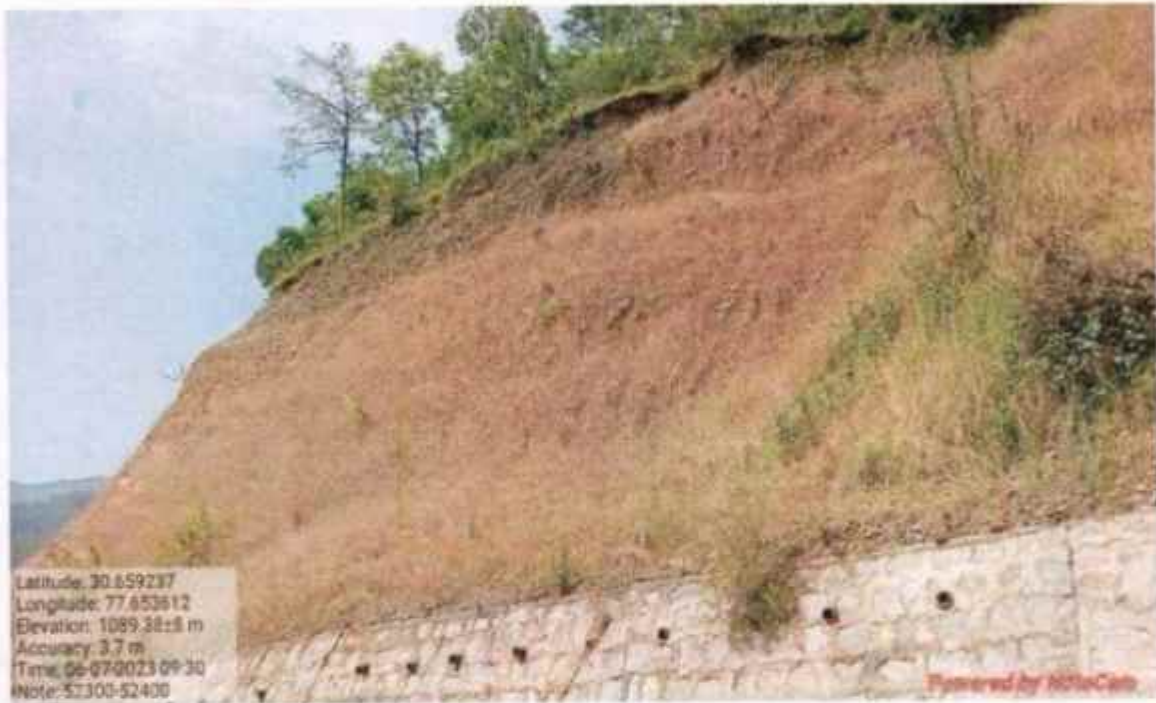
Hydro seeding work at km 52+300 to 52+400
