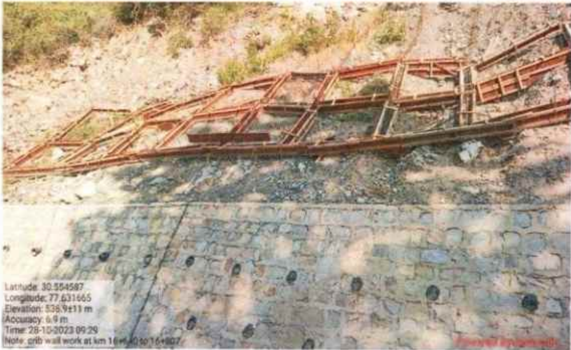
Shotcrete crib wall work at km 16+640 to 16+807
