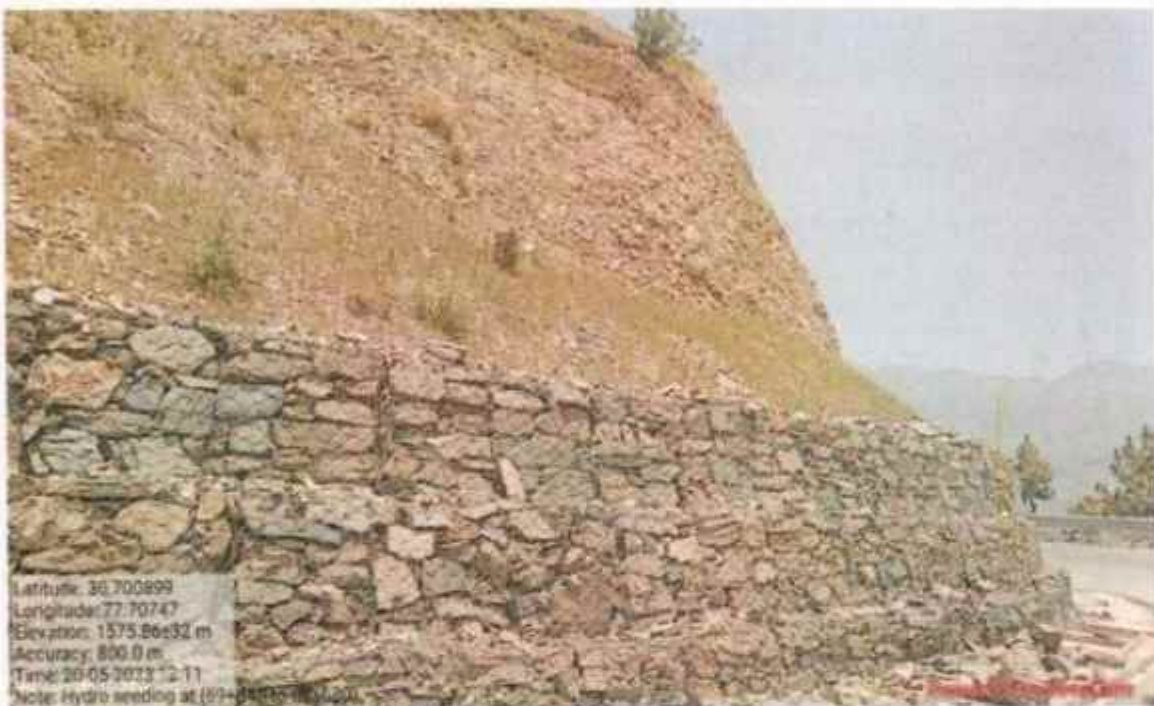
Hydro seeding work at km 69+640 to 69+680
