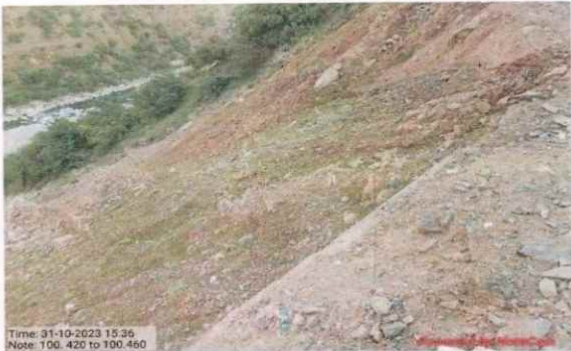
Valley side Bamboo plantation work at km 100+420 to 100+460
