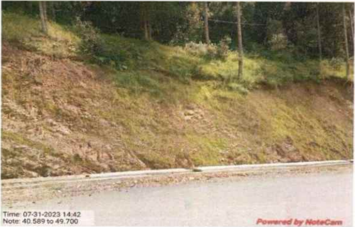
Hydro seeding at km 40+589 to 40+700
