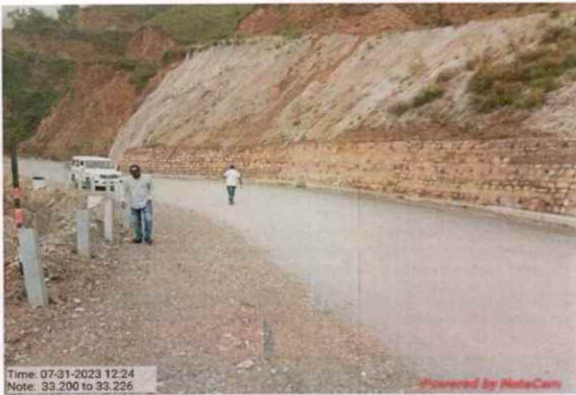
Coco fibre work at km 33+200 to 33+226
