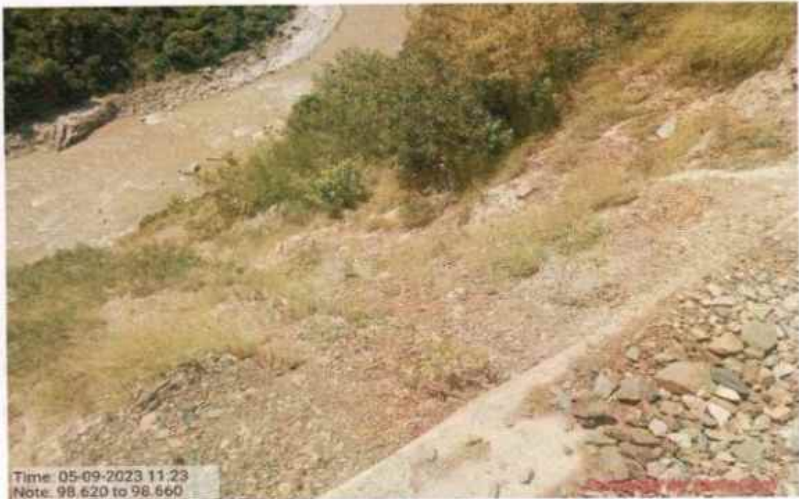
Valley side Bamboo plantation work at km 98+620 to 98+660
