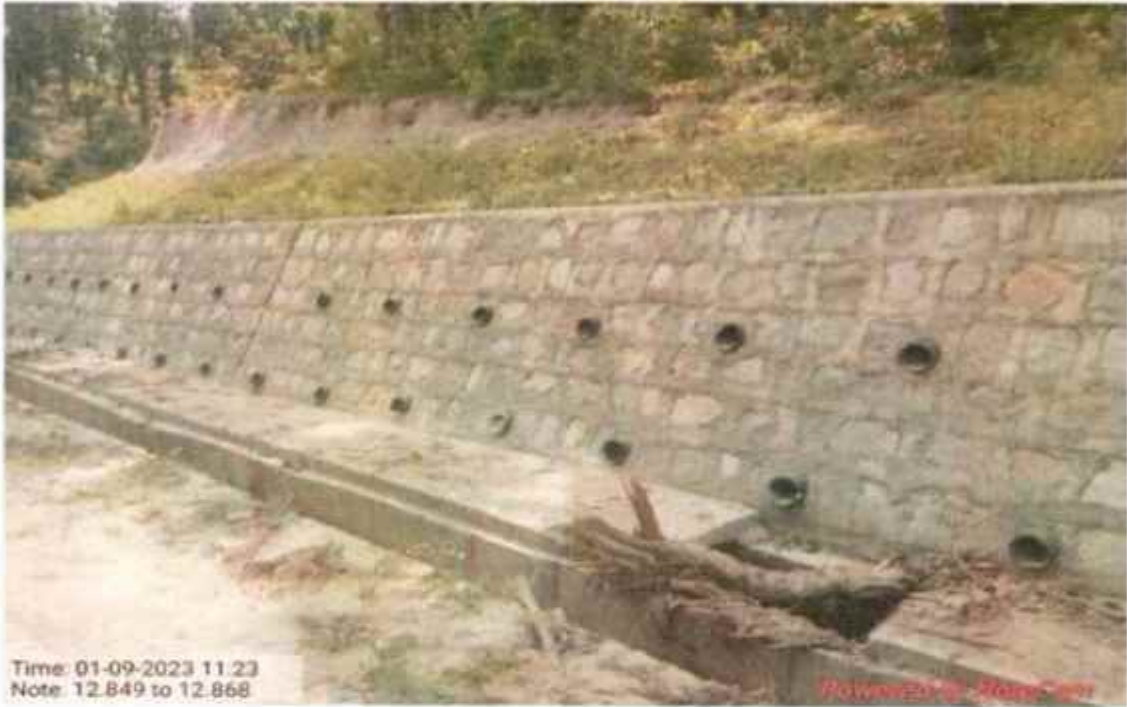
Coco fibre work at km 12+849 to 12+868
