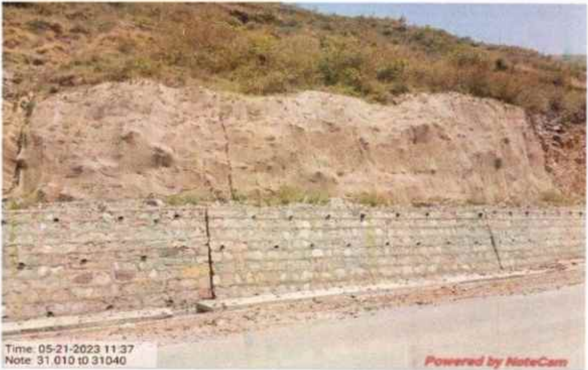
Coco fibre work at km 31+010 to 31+040
