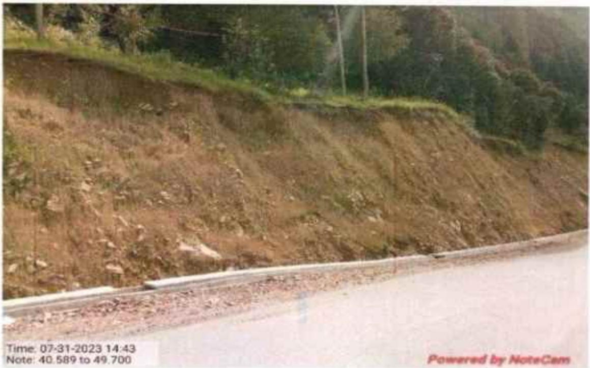
Hydro seeding at km 40+589 to 40+700
