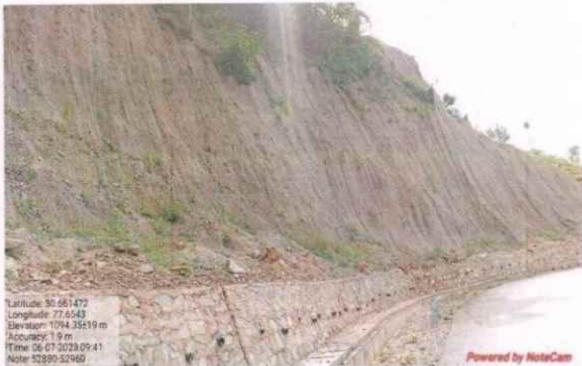
Interlink chain mesh work at km 52+880 to 52+960
