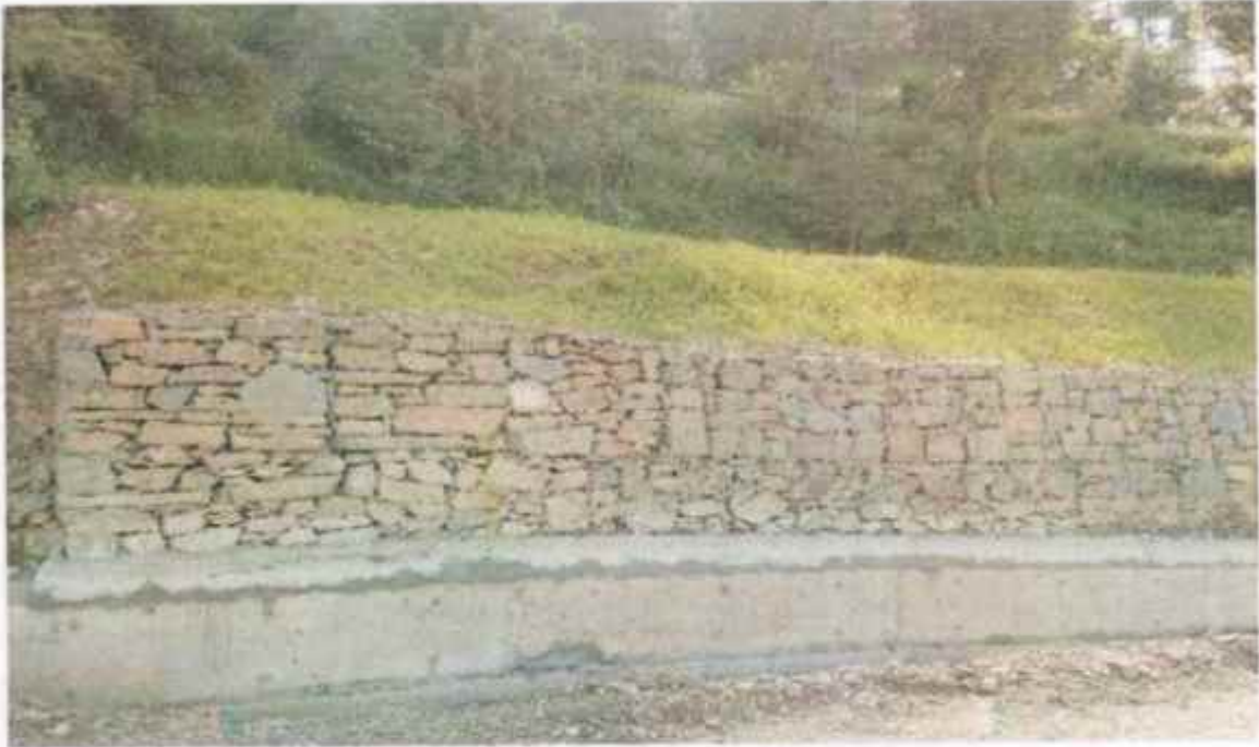
Hydro seeding work at km 70+840
