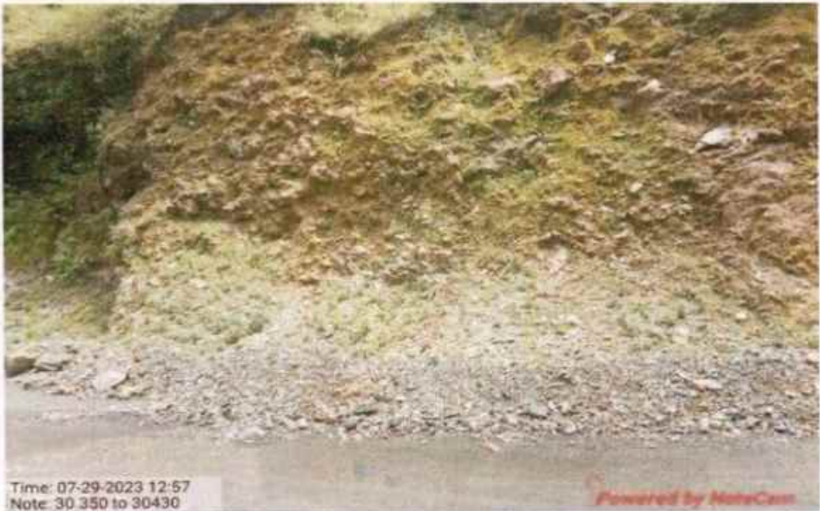
Hydro seeding work at km 30+350 to 30+430
