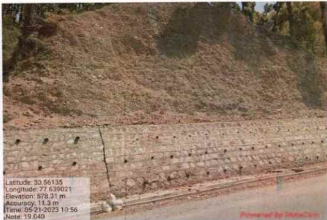
Interlink chain mesh work at Km 19+040
