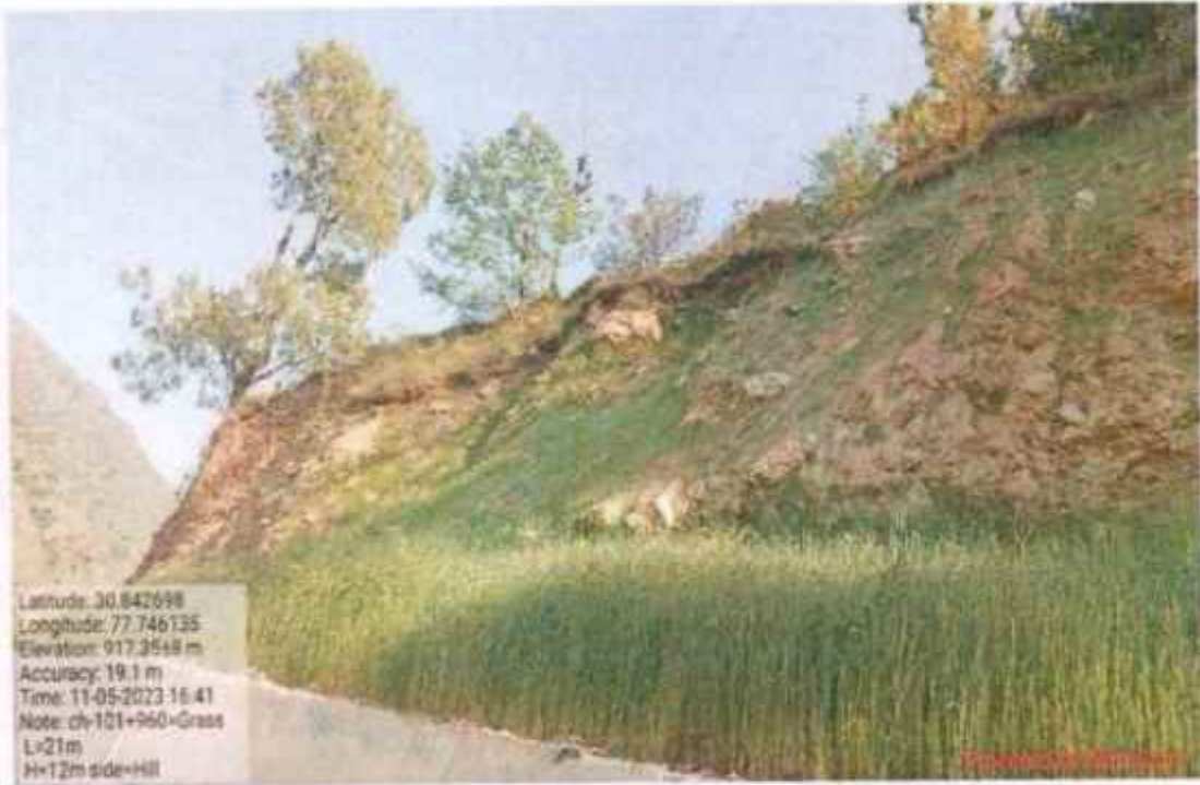
Hydro seeding and Geo cell with hydro seeding work at km 101+960
