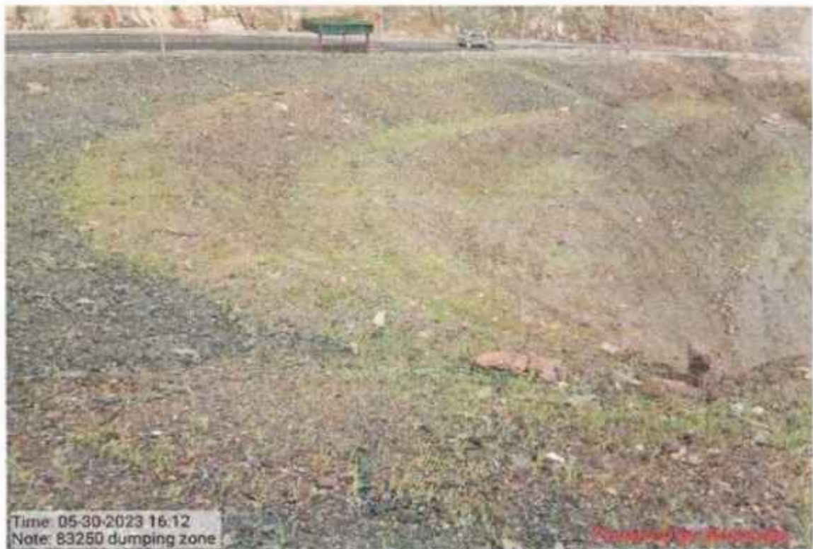
Valley side Bio-Engineering work at km 83+250
