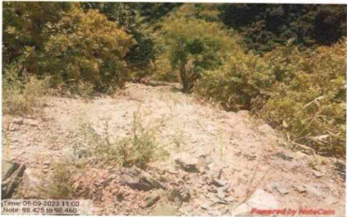
Valley side Bamboo plantation work at km 98+425 to 98+460
