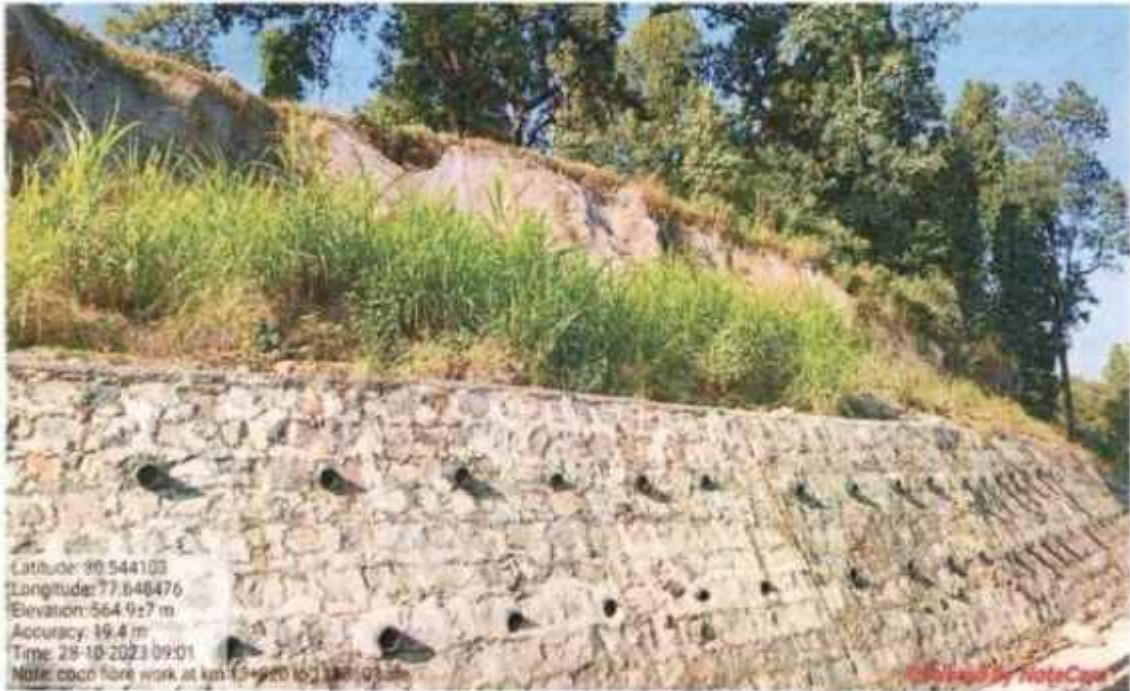
Coco fibre work at km 13+920 13+680.
