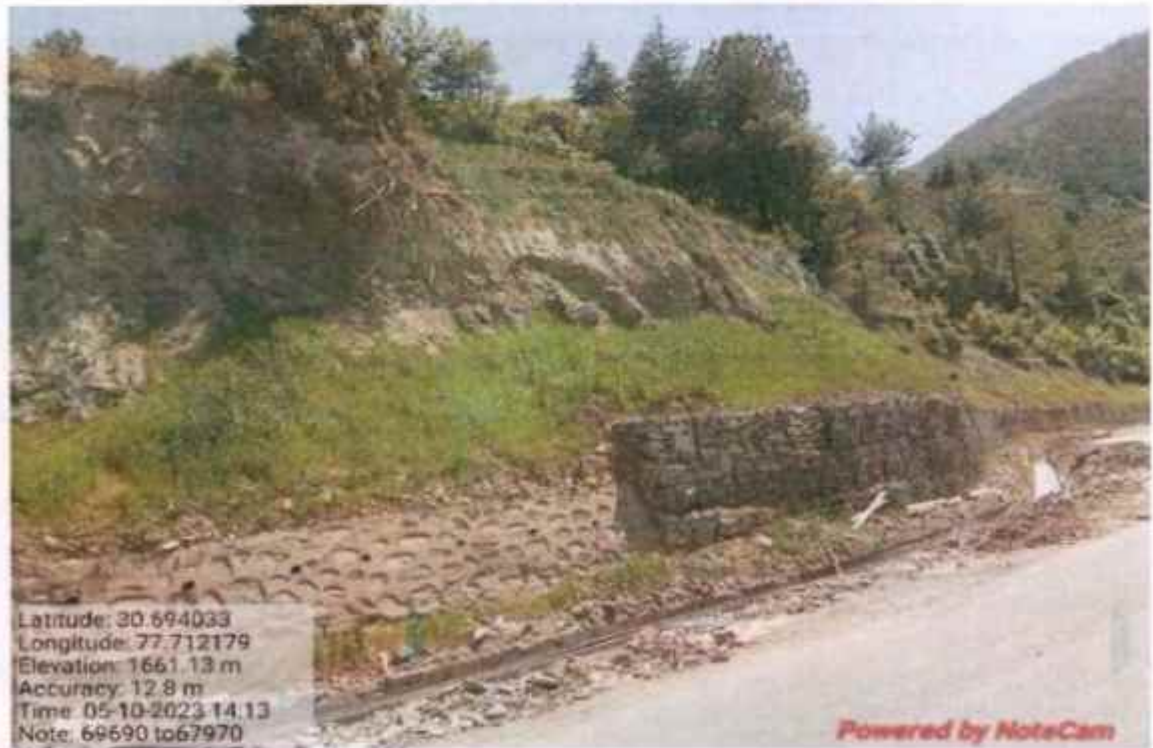
Hydro seeding work at km 69+690 to 69+970
