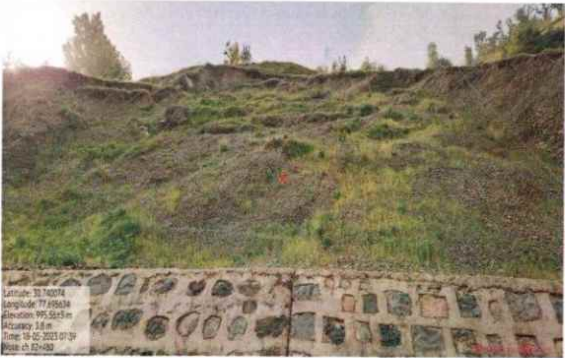
Interlink chain mesh work at km 82+480
