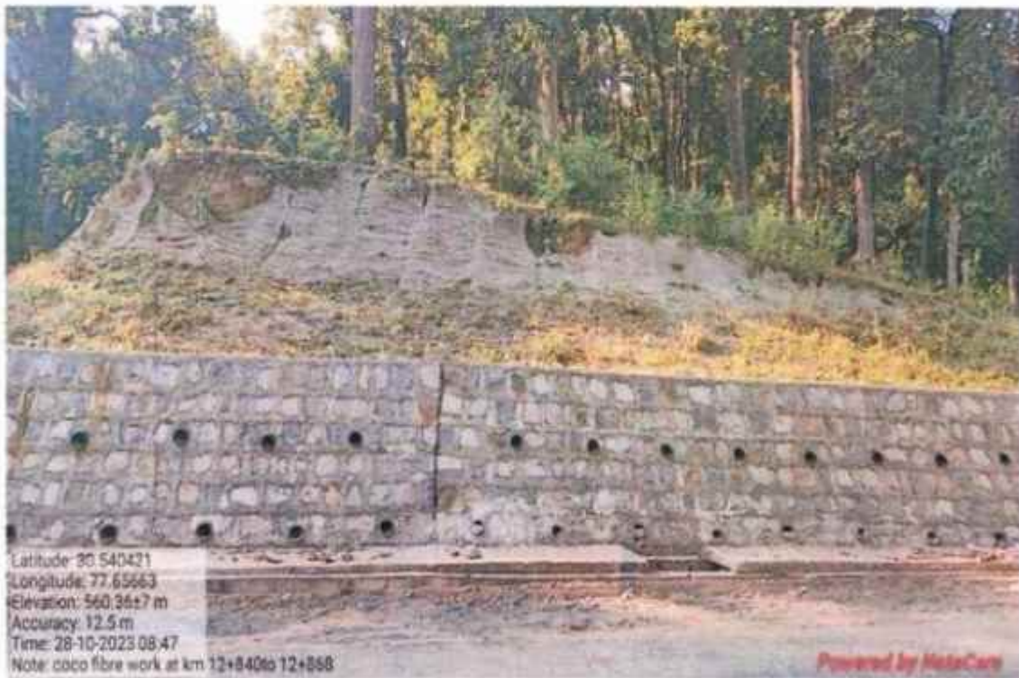
Coco fibre work at km 12+840 to 12.868
