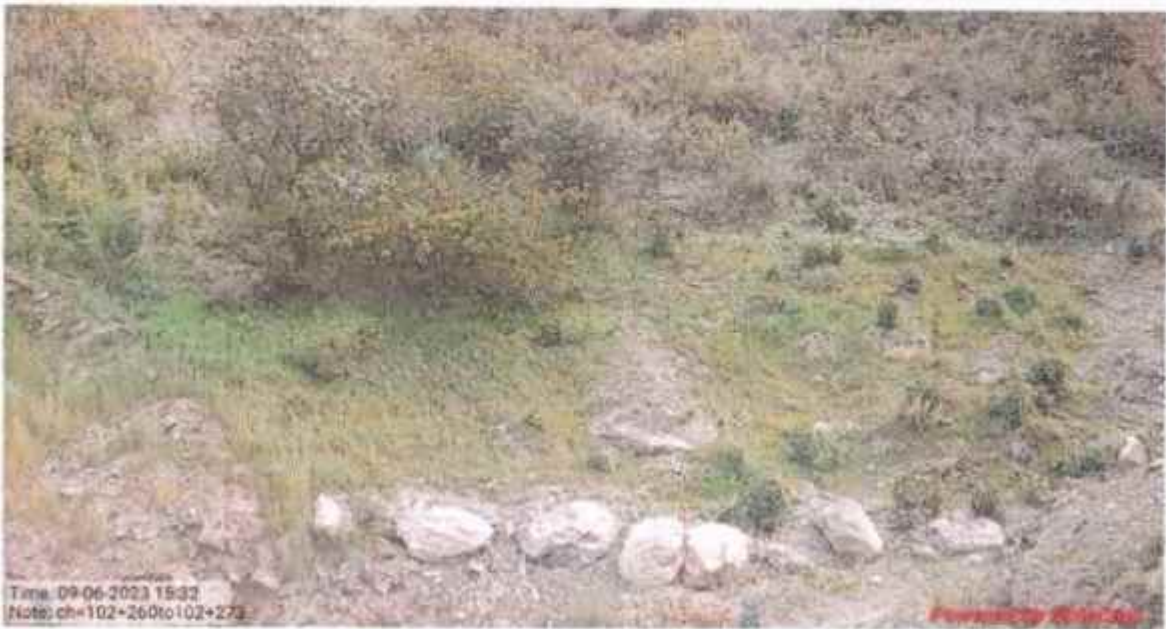
Hydro seeding work at km 102+260 to 102+273
