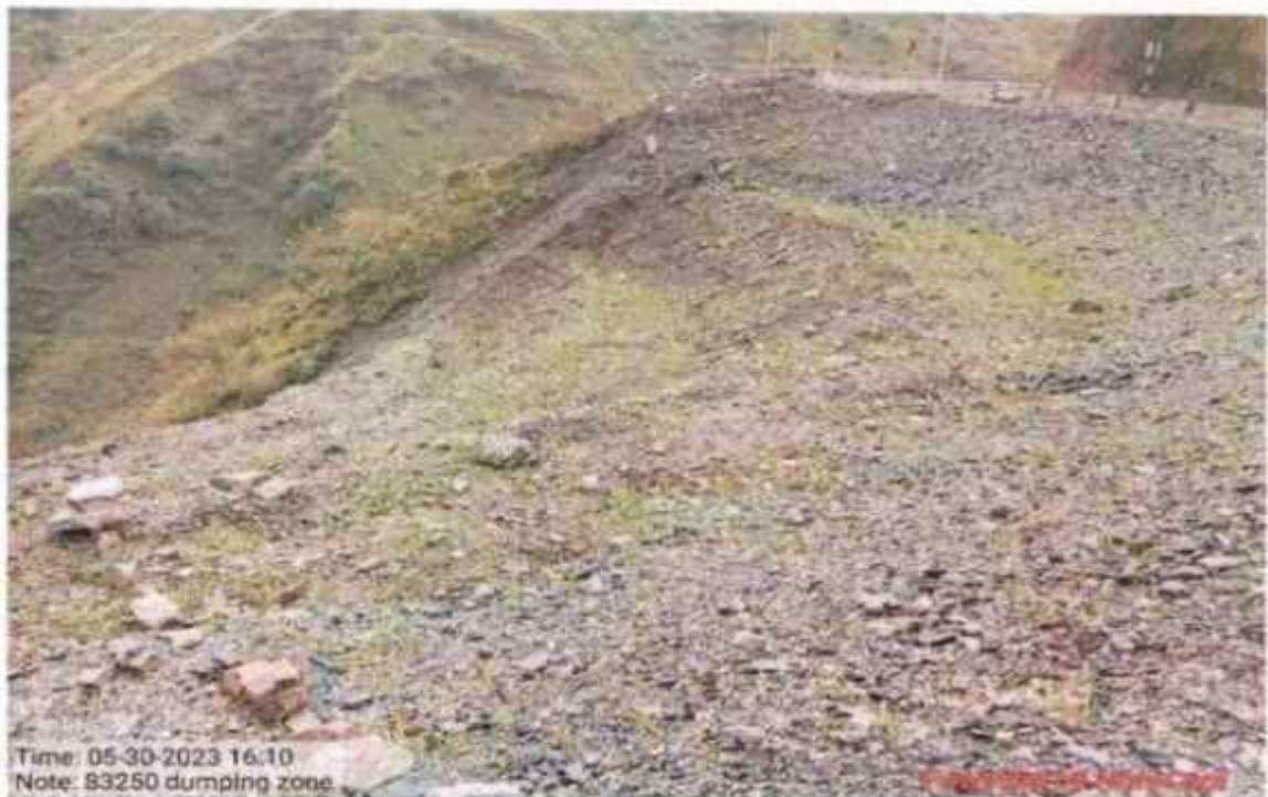
Valley side Bio-Engineering work at km 83+250
