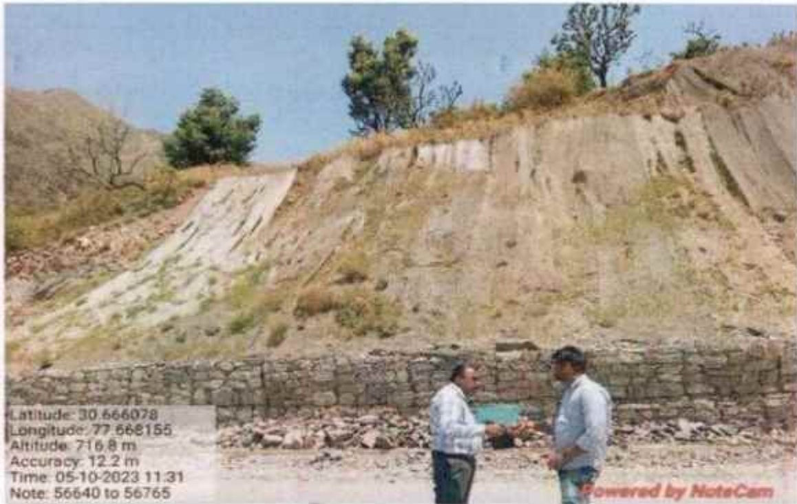
Coco fibre with Grass work at km 56+640 to 56+765
