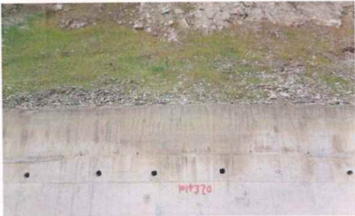
Hydro seeding work at km 101+320
