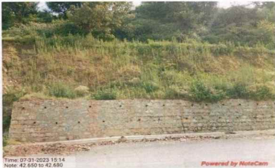
Interlink chain mesh work at km 42+650 to 42+680
