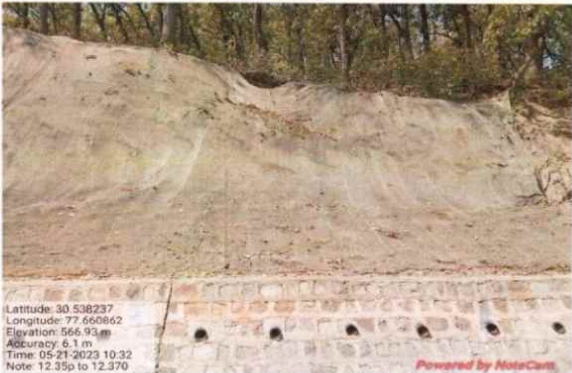
Coco fibre work at km 12+350 to 12.370
