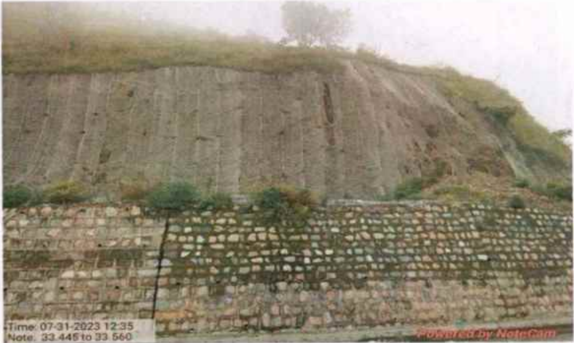
Coco fibre work at km 33+445 to 33+560
