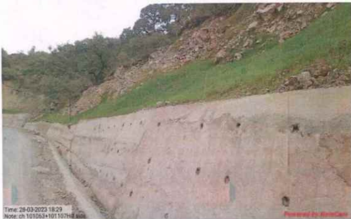
Hydro seeding and Geo cell with Hydro seeding work at km 101+063 to 101+107
