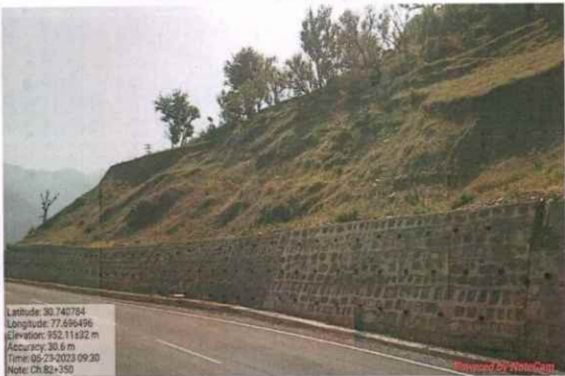
Interlink chain mesh work at km 82+350
