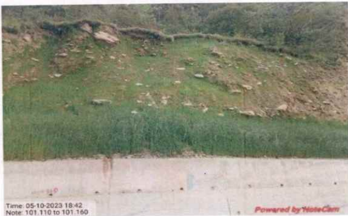
Geo cell with Hydro seeding work at km 101+110 to 101+160
