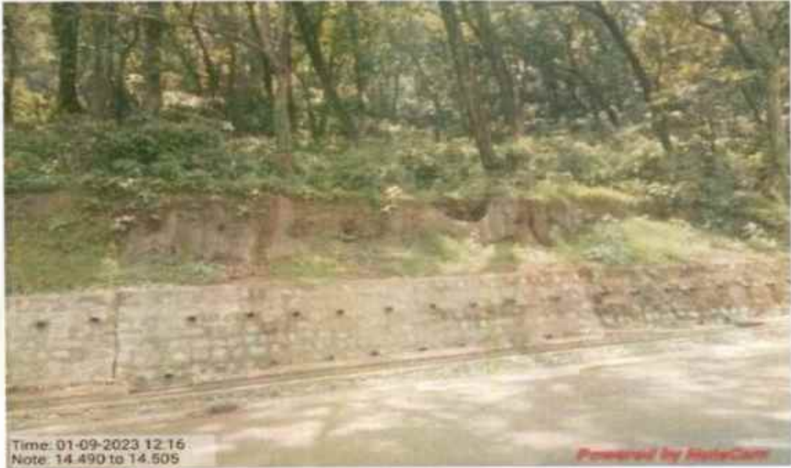
Coco fibre work at km 14+490 to 14.505
