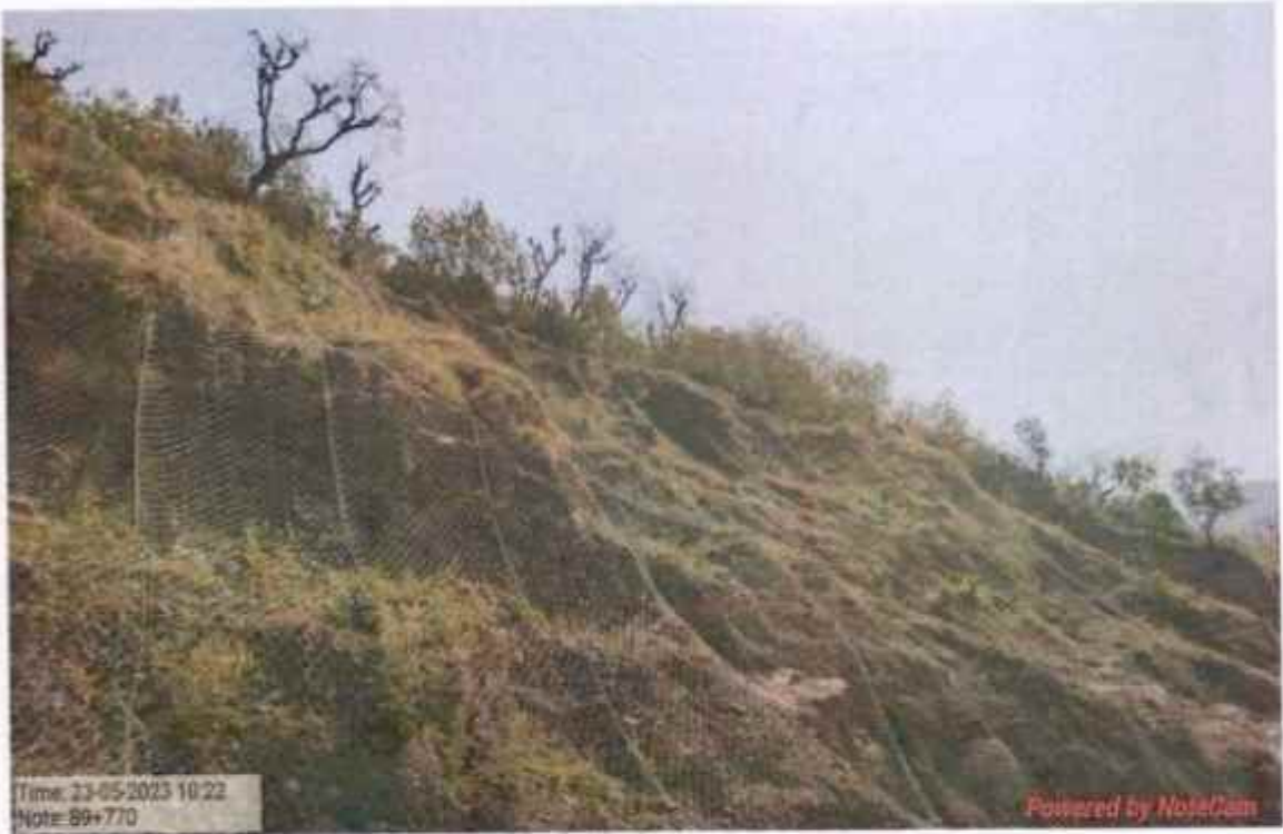
Interlink chain mesh work at km 89+770
