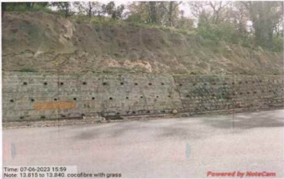
Coco fibre work at km 13.815 to 13+840
