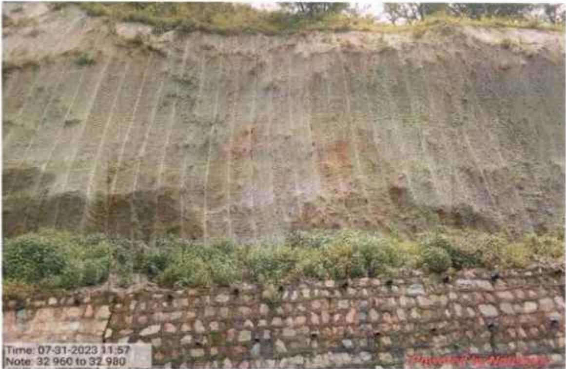
Coco fibre work at km 32+960 to 32+980
