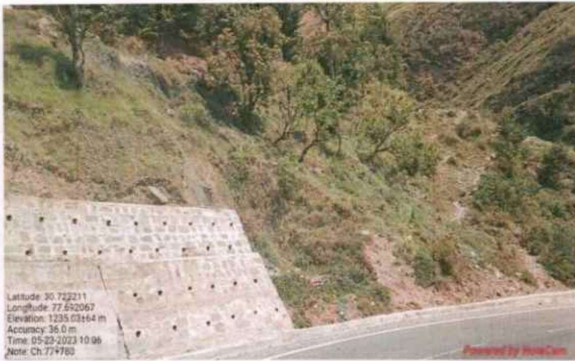
Interlink chain mesh work at km 77+780
