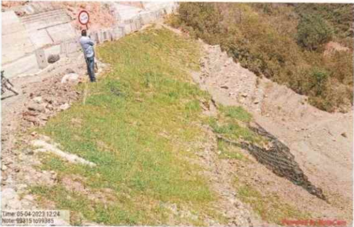
Valley side Geo cell with Hydro seeding and Bamboo plantation work at km 99+315 to 99+385
