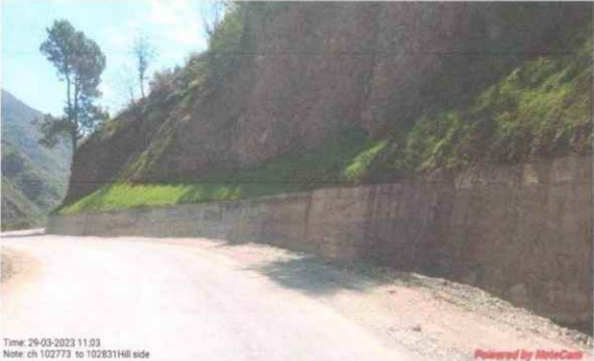
Hydro seeding and Geo cell with Hydro seeding work at km 102+773 to 102+831
