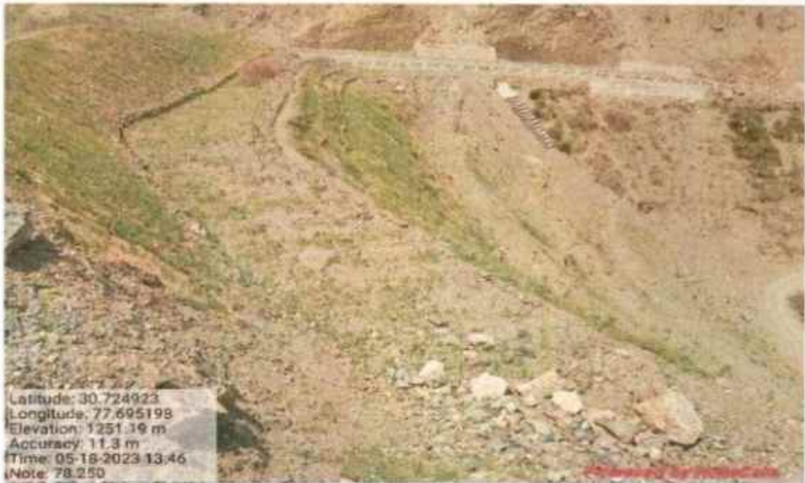
Valley side Bio-Engineering work at km 78+250
