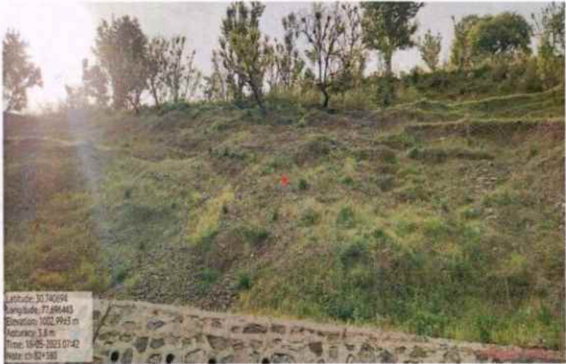
Interlink chain mesh work at km 82+380
