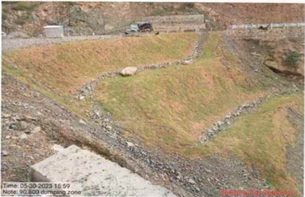
Valley side Bio-Engineering work at km 90+800
