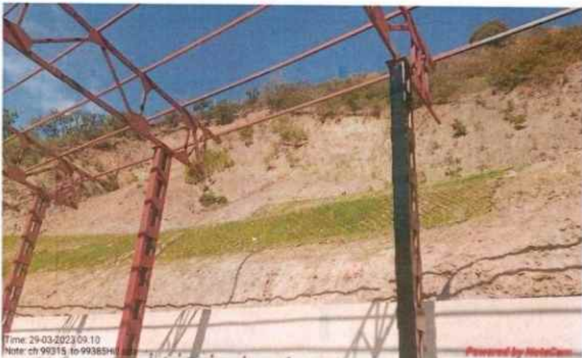
Geo cell with Hydro seeding and Bamboo plantation work at km 99+315 to 99+385
