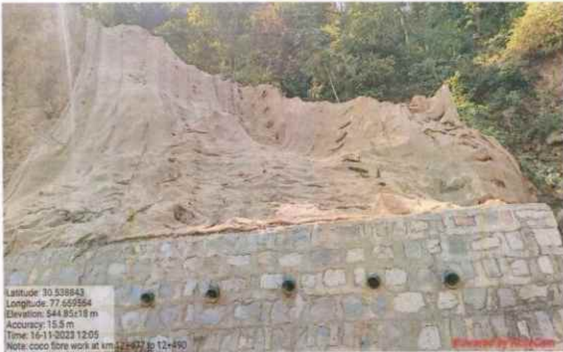
Coco fibre work at km 12+477 to 12+490
